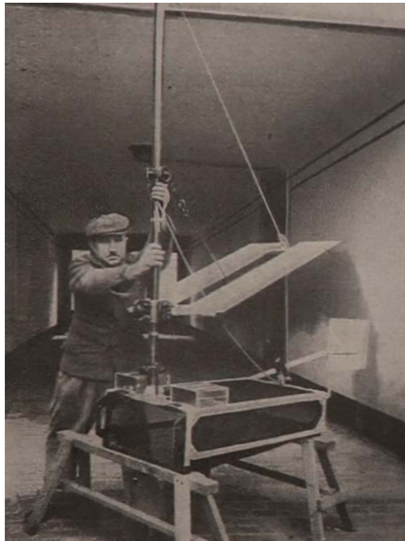
Figure 40 Ehrenberger sampler (Ehrenberger, 1942)
