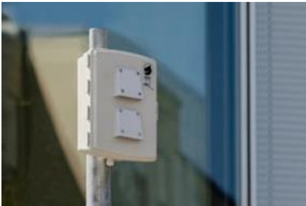
Figure 16: Use of Smart Sense Air Quality Monitoring Solution
