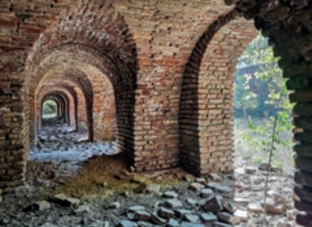
Old masonry from Ada Kaleh island, reconstructed at Şimian Island (RO) © Ministry of Culture of Romania
