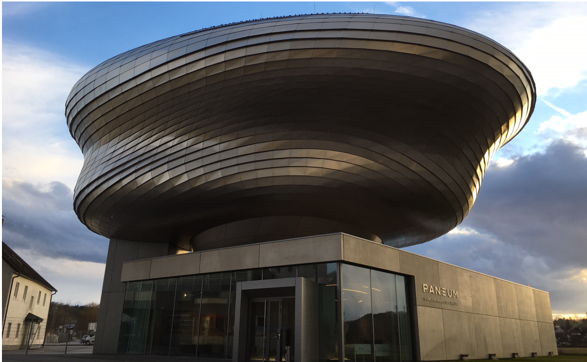
Figure 2: Site visit to Paneum Asten, day 1
