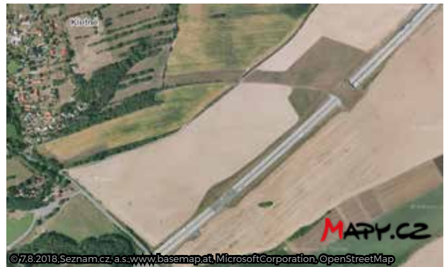
Fig. 11.2 A green bridge on D1 motorway near Suchdol nad Odrou (the Czech Republic) was built on a significant migration corridor between two mountain ranges (Beskydy and Jeseníky). Unfortunately, the crossing point of the migration corridor with the motorway is located in agricultural landscape without a forest cover. Therefore, in order to improve the efficiency of a green bridge, associated land has been purchased to plant new vegetation that will connect the green bridge with further located existing forest cover. © Mapy.cz
