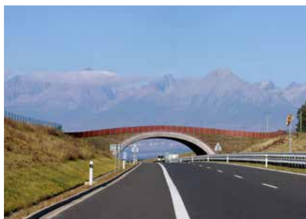
Fig. 1.2 Fauna passages are an example of measures that aim to minimize the negative impacts of transport on wildlife. © Václav Hlaváč
