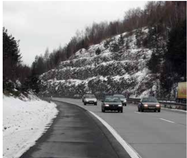
Fig. 9.12 Terracing stabilizes the slopes of deep cuttings and creates micro-habitats for several plant and animal species. © Václav Hlaváč
