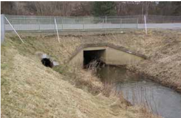
Fig. 10.14 In case it is not possible to adjust an unsuitable bridge as fauna passage, a parallel otter tunnel can be additionally created. It is recommended that terrain modulation or guiding barriers be used in order to help the animals find the entry. © Lukáš Poledník
