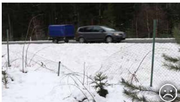
Fig. 10.56 Fences are often damaged, for example by fallen trees or by accidents. Animals usually find these gaps very quickly and get into a dangerous area between the fences. When they are then disturbed, they run across the road and become victims of traffic. © Václav Hlaváč
