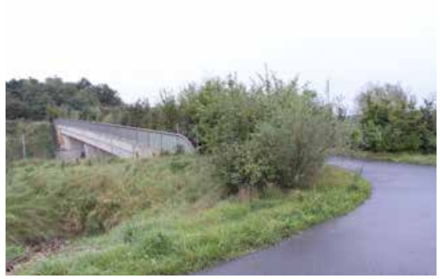
Fig. 10.17 A forest path over a motorway widened by stripes of bushes on both sides allows for the connection of forest environment for many species including mammals living on trees, small birds or bats. It represents a very affordable measure with a strong effect. Dresden, Germany. © Václav Hlaváč
