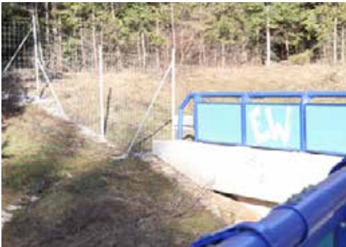
Fig. 10.27 Fencing fluently connected to the protection walls (full railing) is guiding animals which follow the motorway fencing to the entry of a green bridge. D1, Czech Republic. © Václav Hlaváč.
