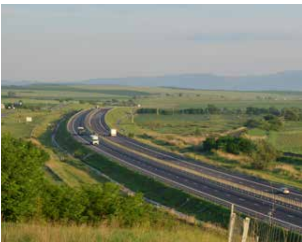
Fig. 9.4 Alignment of a motorway in a flat landscape at ground level with the surrounding terrain is not very disturbing visually but gives only limited possibilities for incorporating effective fauna passages. © Tibor Sos
