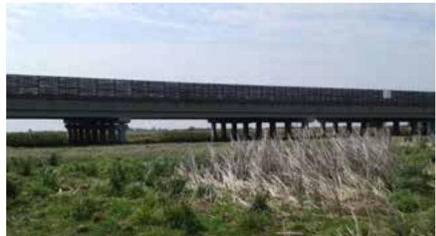
Fig. 6.40 In case it is necessary to overcome the wetlands, a viaduct is usually an optimal solution. However, protection walls to limit disturbances and prevent bird mortality are essential. Motorway M3, Hungary. © András Szirányi
