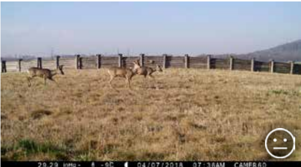
Fig. 10.19 Green bridges represent an ideal solution for most animal categories. Medium sized mammals such as the roe deer use even overpasses that are not planted with bushes. However, usability of such overpasses for mammals such as the red deer or large carnivores is limited. Czech Republic, D1, Suchdol. © Friends of the Earth, Czech Republic
