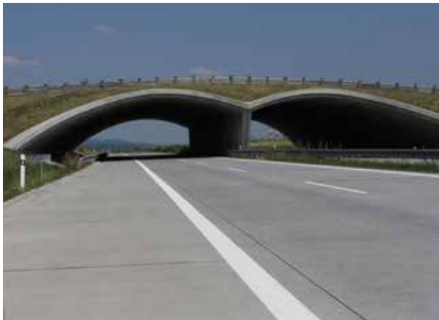
Fig. 9.7 When necessary, it is possible to allow for movement of large mammals even in flat landscapes – by means of green bridges. It however requires larger land occupation to merge the overpass with the surrounding landscape. © Václav Hlaváč
