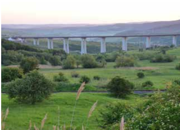
Fig. 9.8 Viaducts are usually better options to cross valleys than embankments because they allow for free movement of animals and partly maintain connectivity of habitats as well. Aciliu viaduct on A1 motorway (Bucuresti - Nadlac) in Romania, Sibiu County. © Tibor Sos
