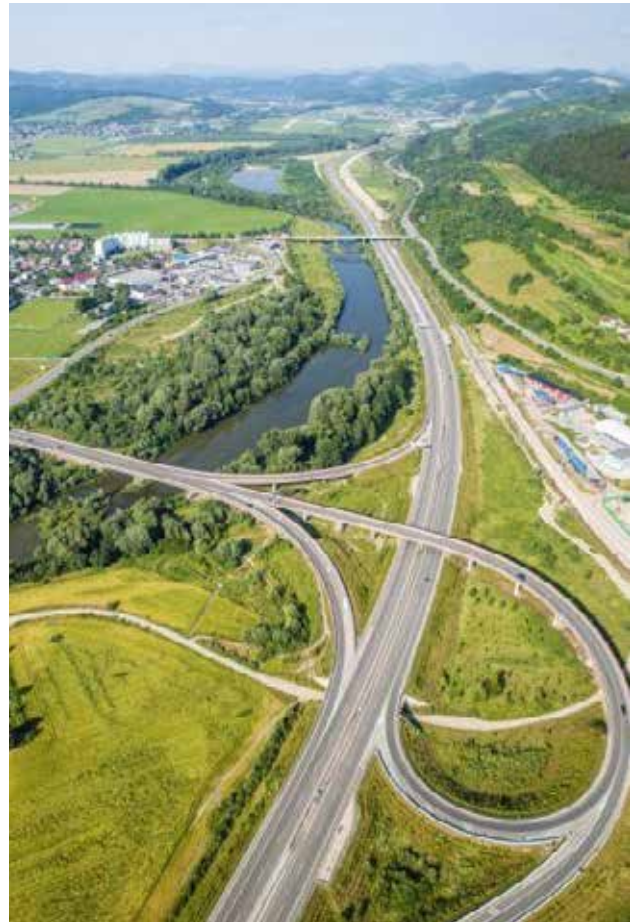
Fig. 7.8 The ultimate objective of TEN-T is to close the gaps, remove the bottlenecks and eliminate the technical barriers that exist between the transport networks of the EU Member States. D1 motorway in Slovakia (in the picture) belongs to the TEN-T network. © NDS Archive
