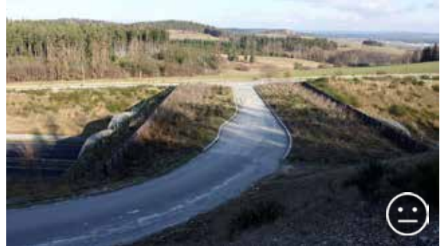
Fig. 10.29 A multi-purpose overpass with a local path, where the main purpose is to allow animal movement. When well implemented, this solution is suitable for small and medium-sized mammals, but large mammals often do not accept it. Multi-purpose overpasses are completely undesirable in places where infrastructure crosses a long-distance migration corridor. Písek, Czech Republic.
