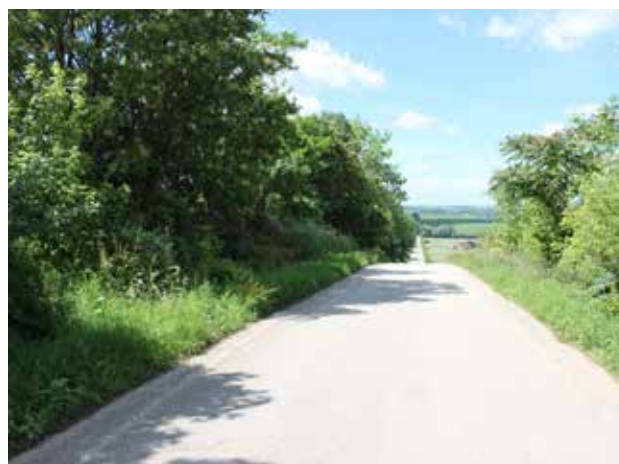
Fig. 9.23 Road verges with high vegetation decrease lookout conditions for both drivers and animals, which can increase the probability of an accident. © Michal Ambros
