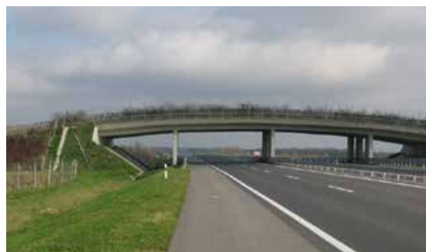
Fig. 6.42 A green bridge can be built even in a flat lowland area where the motorway is at ground level with the terrain. Connecting the bridge to the surrounding terrain however represents a more extensive land occupation compared to a situation where the motorway leads in a notch. Motorway M7, Hungary. © Ábrahám László
