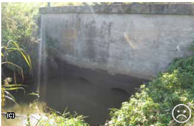
Fig. 10.46 Examples of inappropriate solutions. Culverts where the entrance is technically designed in a way that prevents the animals from entering. © Lukáš Poledník - A) and D), Václav Hlaváč - B), Jitka Matoušová - C)
