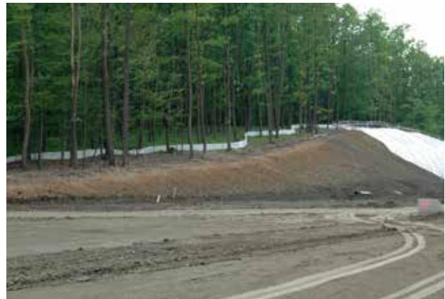
Fig. 8.6 Temporary barriers are used to prevent amphibians from entering the construction site. In such cases animals should be directed to a suitable passage or have to be captured and transferred to appropriate environment. © Naturaservis, Ltd.
