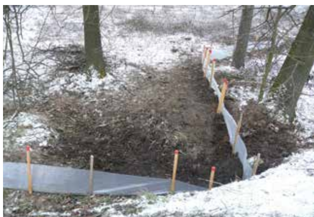
Fig. 10.57 During spring migrations, the installation of temporary barriers can prevent amphibians from entering roads and at the same time direct them to safe passages. The barriers must be removed after the migrations are over. © Jaromír Maštera
