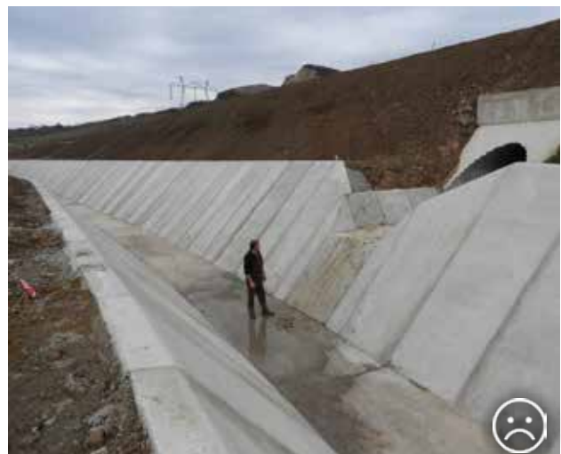
Fig. 9.19 Massive concrete trough for drainage of precipitation waters from a motorway is very disturbing as far as landscaping is concerned, and it does not allow using culverts as fauna passages. Such a solution also represents a trap for smaller animals that have no means of leaving the trough. © Ivo Dostál
