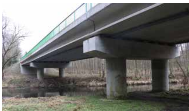
Fig. 6.41 A properly designed bridge across a watercourse allows for free movement of water, semiaquatic and terrestrial animals. Sufficiently wide banks without technical adjustments allow for movement of all animal categories. Moreover, bridges designed in this way are also able to safely convey flow rates during floods, associated with climate change. © Václav Hlaváč
