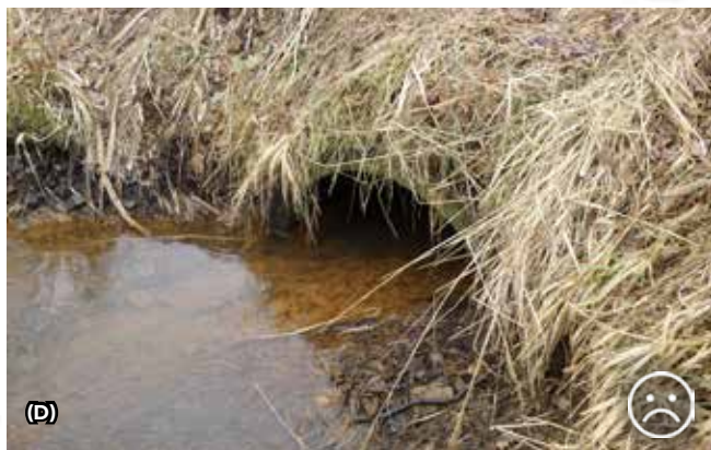
Fig. 10.46 Examples of inappropriate solutions. Culverts where the entrance is technically designed in a way that prevents the animals from entering. © Lukáš Poledník - A) and D), Václav Hlaváč - B), Jitka Matoušová - C)
