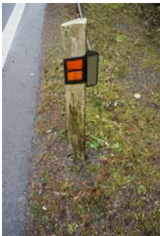
Fig. 12.19 Artificial animal light deterrent equipped on a roadside post. The reflective element reflects light from an approaching car to the road side and by that warns the animals. Decrease of animal traffic mortality due to such light deterrents has so far not been satisfactorily confirmed. Beskydy, the Czech Republic. © Martin Strnad
