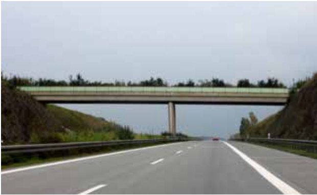
Fig. 10.18 A forest path over a motorway widened by stripes of bushes serves as a fauna passage for small bat species. However, this overpass can be used by a broad spectrum of other animal species as well. Germany. © Václav Hlaváč
