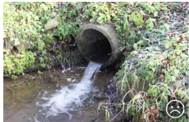
Fig. 10.3 A vertical step on an outflow from a culvert causes a migration barrier for fishes such as the common minnow or the brown trout. © Václav Hlaváč
