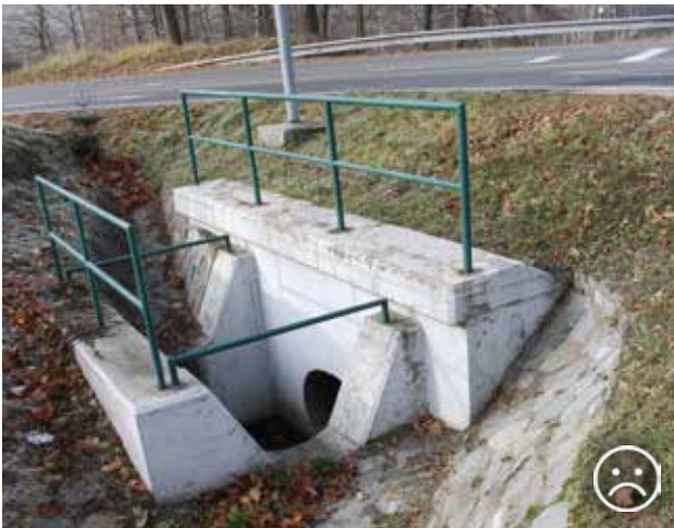
Fig. 10.6 Sumps at the entry or exit prevent amphibians from using such a culvert for migration. Such solutions can moreover create fatal traps where tens of amphibians die. © Václav Hlaváč
