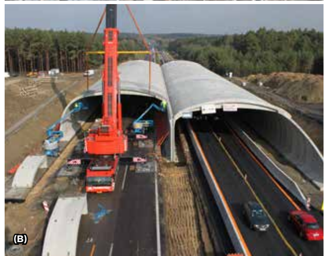
Fig. 9.16 A) Construction of the bored tunnel Višňové on motorway D1, Slovakia. B) Construction of a cut-and-cover tunnel - green bridge near Moravský Svätý Ján, Slovakia. © NDS Archive
