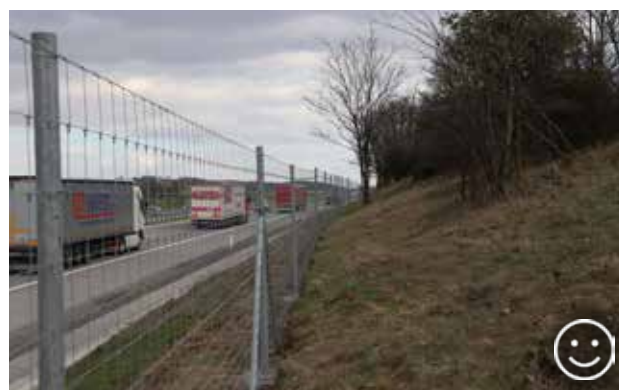
Fig. 10.53 A correctly placed fence. Trees and bushes represent an attractive habitat for a whole range of species; therefore, they should stay outside of the fenced area. It is also easier to check the functionality of fences placed in this manner than compared to fences placed at the edge of a cutting or an embankment. © Václav Hlaváč
