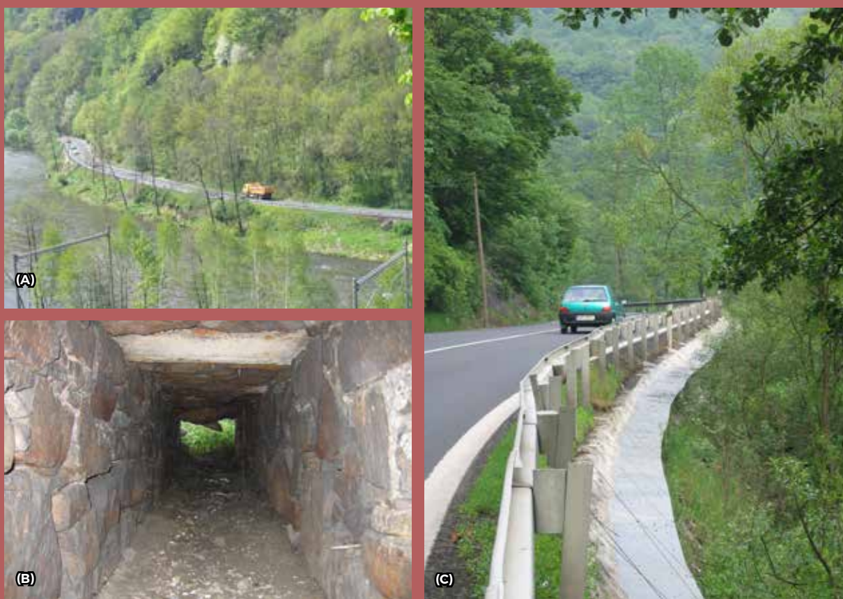
Fig. 10.7 Case study: Special barrier to prevent the Aesculapian snake mortality in the Czech Republic. © Photos by Zamenis, z.s., Source: Musilová et al. 2010
