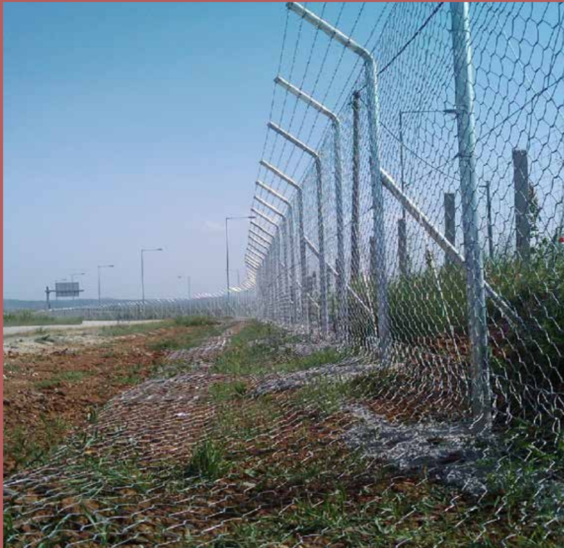
Fig. 10.55 Case study: Fence design for protection of bears (example from Greece). © Lazaros Georgiadis/ARCTUROS
