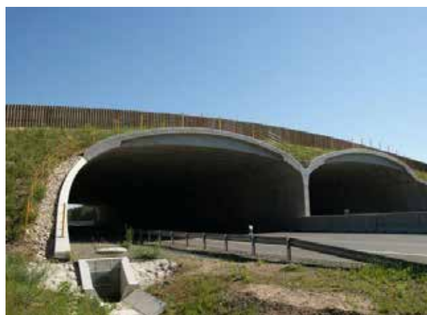
Fig. 7.6 One of the objectives of the Protocol on Sustainable Transport is to minimize the negative impact of transport on nature. The Green bridge Moravský Svätý Ján on D2 motorway (Slovakia) was built to support the restoration of animal migration in the Alpine-Carpathian corridor, which was interrupted by high-level roads and settlements between the Alps and the Carpathian Mountains. © Dušan Valachovič
