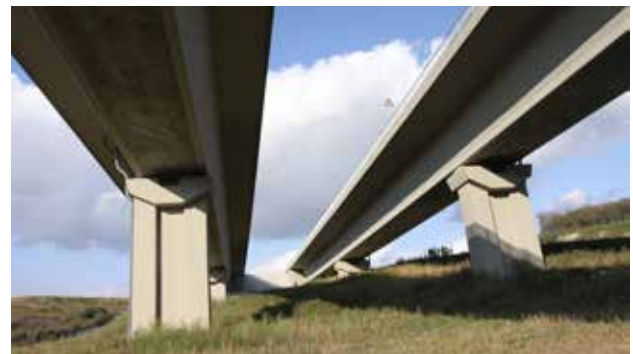
Fig. 10.35 When a viaduct has a split construction, the surface under the bridge has enough light and precipitation for the growth of vegetation. That allows for a better connection of habitats. On the other hand, the overall width of impacted area is greater compared to a unified construction, which is also true for noise intensity under the bridge. Hungary. © Václav Hlaváč
