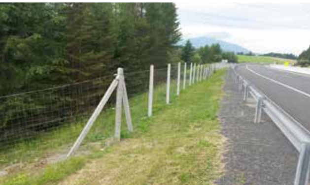
Fig. 6.19 Fences prevent animals from entering the roads and improve traffic safety, but they significantly increase the barrier effect. They should therefore only be built where animals also have the opportunity to cross the infrastructure using a safe fauna passage. © NDS Archive
