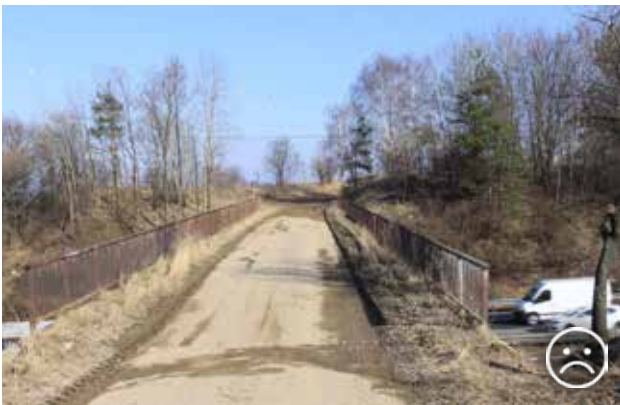
Fig. 10.10 Overpasses for field and forest paths constructed with asphalt or concrete surfaces are not used by animals. Overpasses with grassy stripes on the sides are sometimes used by the hare, the stone marten or the fox. Disturbance by traffic in the case of a motorway constructed below is a limiting factor for most animals. © Václav Hlaváč
