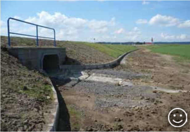
Fig. 10.58 Permanent barriers are built with the goal to guide migrating amphibians to a suitable passage. They are always constructed from both sides - in the direction of spring migration towards aquatic habitats and in the opposite direction from the aquatic to terrestrial habitats. © Jaromír Maštera
