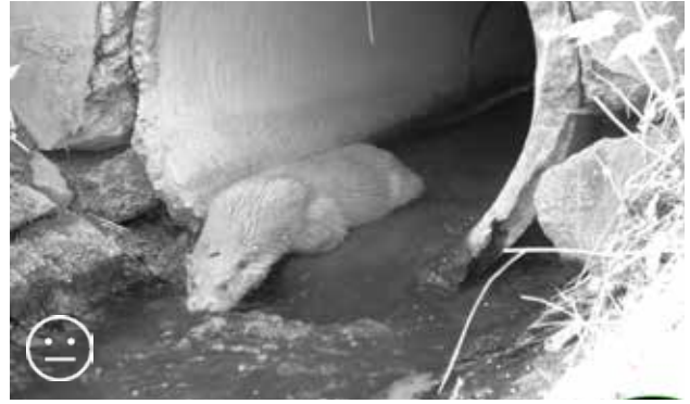
Fig. 6.35 Culverts can – with a suitable design – serve as fauna passages for many animals. Rectangular shape is always the preferred solution. Tube culverts are not an optimal solution, but otters are able to use them at times of lower flow rates. © Václav Hlaváč, phototrap picture
