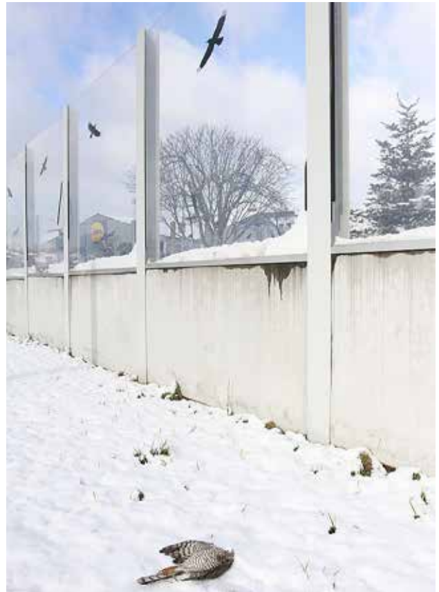
Fig. 6.43 Transparent walls along roads in towns are often the cause of high bird mortality. Formerly used silhouettes of raptors are not a functional protection, so it is necessary to apply a solution that allows the birds to note the barrier in time. © Václav Hlaváč
