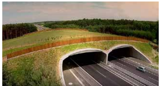
Fig. 6.36 In cases when bridges that could be adapted for use as fauna passages do not exist, special passages must be built to ensure a safe crossing of the motorway with the wildlife corridor. Overpass on D2, Slovakia. © NDS Archive
