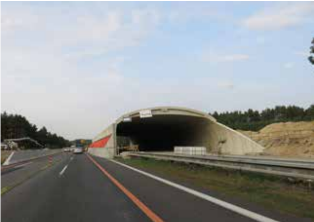
Fig. 8.11 Green bridge near Moravský Svätý Ján (Slovakia) was built during operation of existing motorway D2. The original motorway was completely impermeable in a long section; in this place it crosses the Alpine-Carpathian wildlife corridor. © Václav Hlaváč
