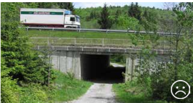
Fig. 10.40 This underpass with a forest path does not represent a suitable passage for fauna. Dimensions w = 6 m, h = 5 m, l = 33 m ( OI = 0,9 ) are insufficient for large mammals, medium-sized mammals such as the roe deer or the wild boar use such underpasses only when disturbances are eliminated (protection wall along a motorway, limited human activities). The Czech Republic, motorway D1. © Václav Hlaváč
