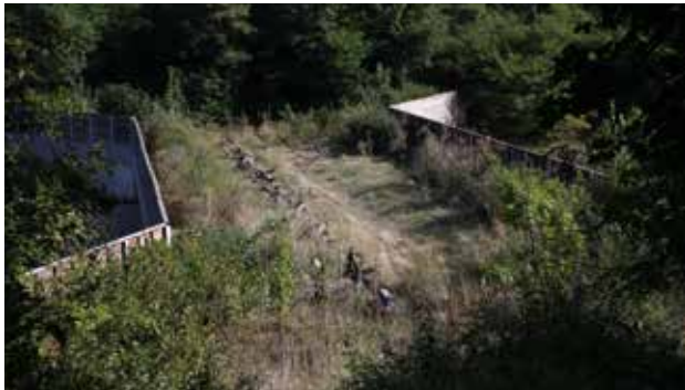
Fig. 10.25 A green bridge with suitable management. Dead wood and planting of bushes on the sides were used during construction and subsequent succession led to a good natural connection to the surrounding environment. France. © Václav Hlaváč .
