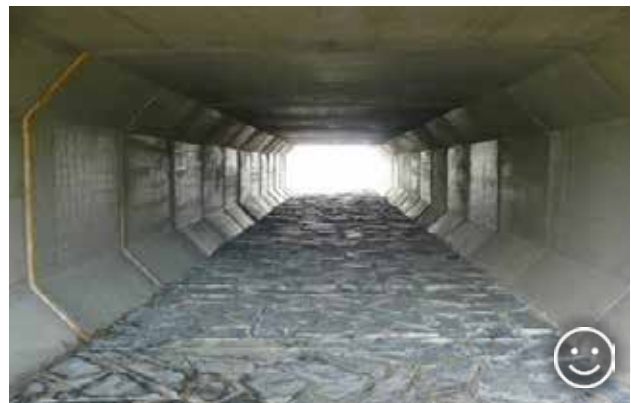
Fig. 10.5 A rectangular culvert is always a better solution for amphibians than a tube culvert. The surface of the underpass is very important for amphibians; a stone pavement is a suitable solution. © Václav Hlaváč
