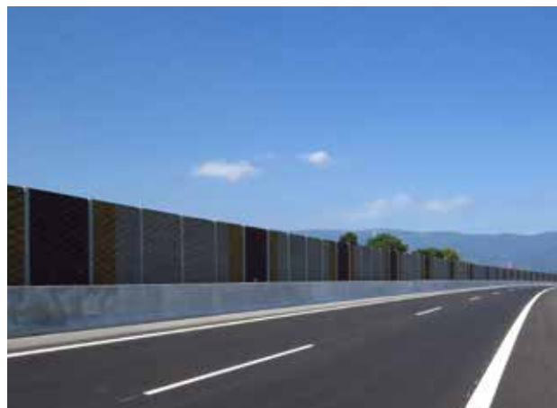
Fig. 4.8 A noise protection wall eliminates the effect of disturbance while also increasing the barrier effect. © Tomáš Flajs
