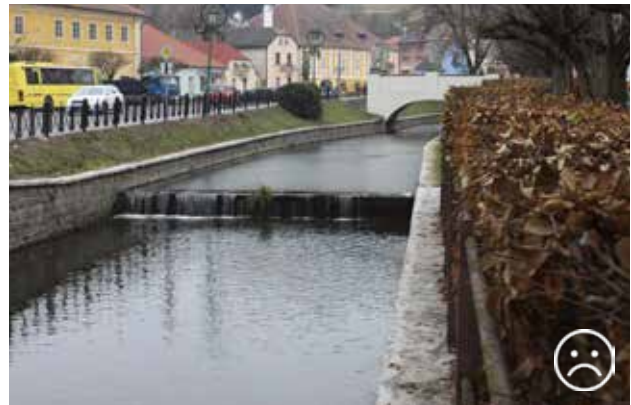
Fig. 10.15 A weir in combination with vertical walls on both sides of a watercourse in a town, forces animals such as otter or beaver to walk around such a place. The animals then often have to cross roads while going around such barriers. © Václav Hlaváč
