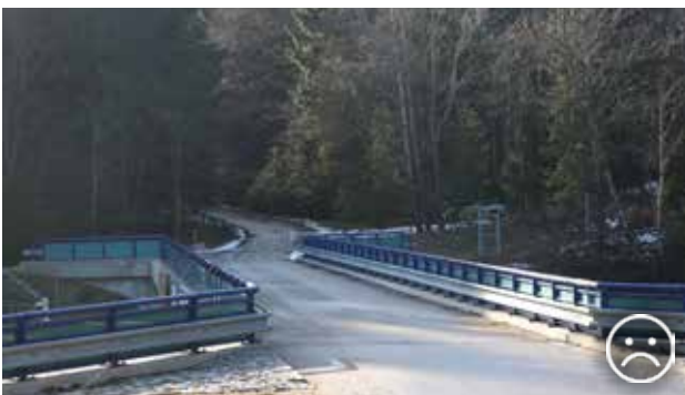
Fig. 10.31 Non-transparent full railing was installed on this bridge with a forest path for disturbance elimination. However, the asphalt surface is completely unsuitable for animal movement, therefore this solution is in general insufficient. Czech Republic, D1 near Jihlava. © Václav Hlaváč
