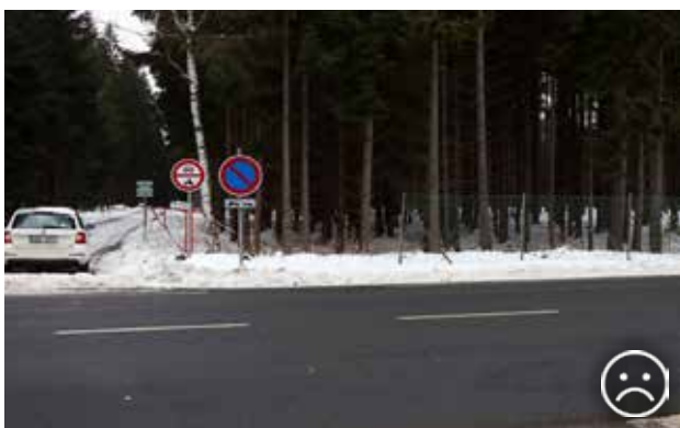
Fig. 10.52 Fencing interrupted by a connection to a forest path. This first-class road was fenced because of a high number of collisions with animals. Unfortunately, due to several exits of connected forest paths the fencing is not continuous. The number of accidents in the observed section increased even more after the fencing was installed, because the passing animals were getting inside of the fenced area without a possibility to escape. © Václav Hlaváč
