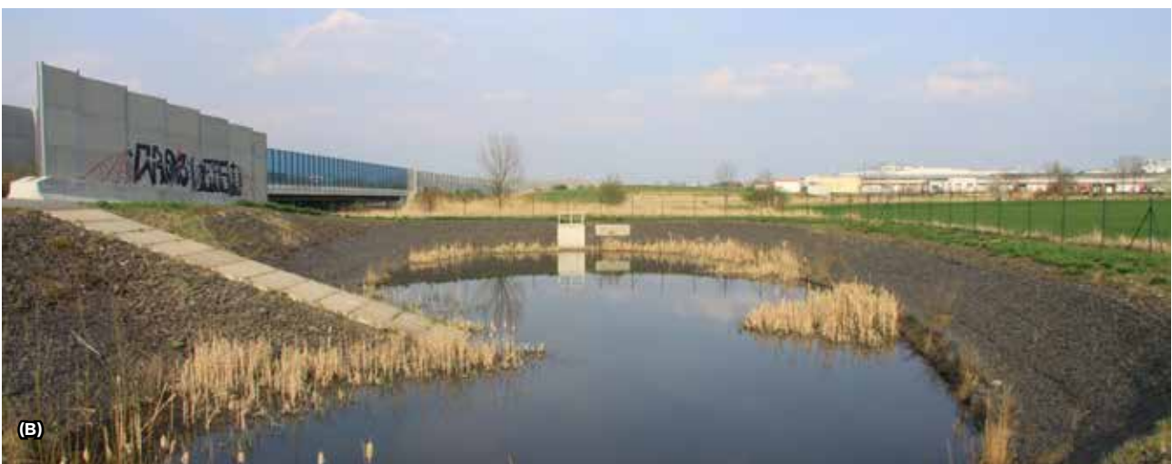
Fig. 4.12 Reservoirs to capture water from motorways are sometimes part of their constructions. When constructed as concrete tanks with vertical walls (A), they form traps for many animals. Optimal solution is to design these capture tanks as natural habitats (B). © Petr Anděl (A) and Martin Strnad (B)
