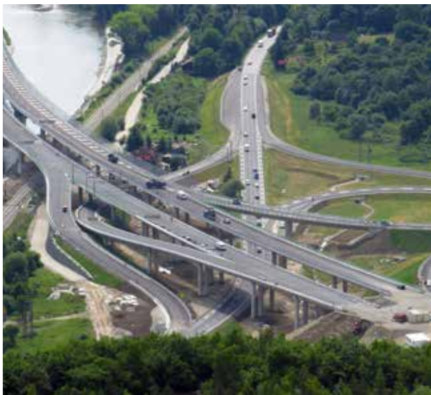
Fig. 9.15 Infrastructure junctions always comprise a significant land occupation. In their design, it is necessary to avoid destruction of valuable communities and creation of ecological traps for animals that are drawn by attractive habitats inside the junctions or for migrating animals that follow motorway fencing and can be pushed to dangerous places. Junction near Vrútky, Slovakia. © Tomáš Flajs
