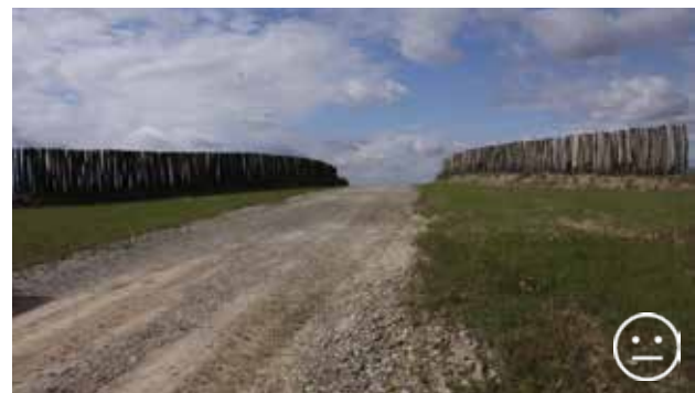
Fig. 10.32 A multi-purpose overpass like this has only a limited use for fauna. Suitable hiding places and microhabitats for small animals are missing, similarly, to bushes for larger animals. The need for hiding places is increased by the fact that the animals do not see a safe habitat at the other side of the overpass. © Václav Hlaváč
