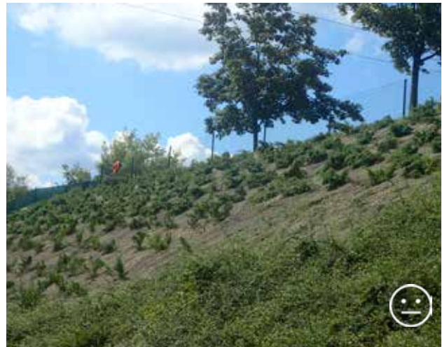
Fig. 9.21 Vegetation planting is often done with the purpose of slope stabilization. However, these bush or tree covers can create an attractive habitat for many species, including large mammals. When the vegetation is planted in the area between a fence and a road, it can tempt animals into the dangerous fenced space. © NDS Archive
