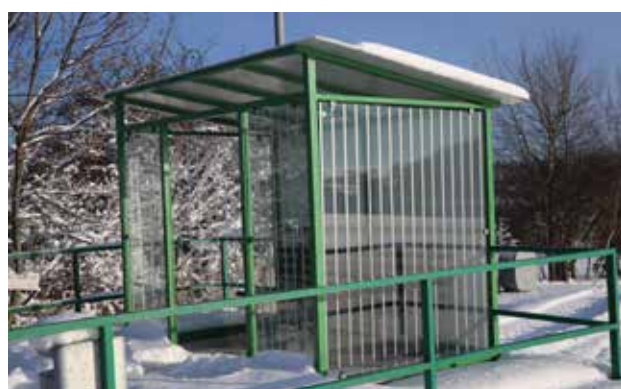
Fig. 10.62 Besides transparent protection walls, bus stops can become places of high bird mortality as well. The means of securing is similar in both cases. (The first bus stop on the top has been secured by school children, who did not want to find any more dead birds there). © Petra Hulvová
