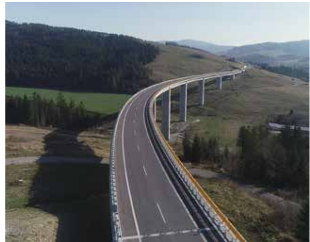
Fig. 9.3 Leading a road higher along a hillside allows for good solution of permeability for animals (e.g. viaducts over smaller side valleys), but has a disadvantage in impacting new natural areas. D3 Svrčinovec - Skalité, Slovakia. © NDS Archive
