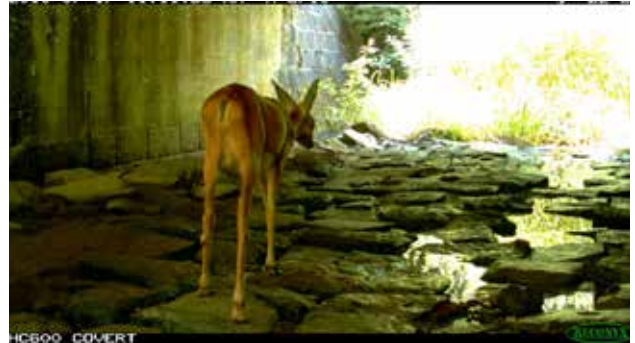
Fig. 10.20 The roe deer usually use underpasses with openness index greater than 1. This underpass under a railway is 5 m wide, 3 m high and 15 m long (OI = 1). © Václav Hlaváč, photo trap
