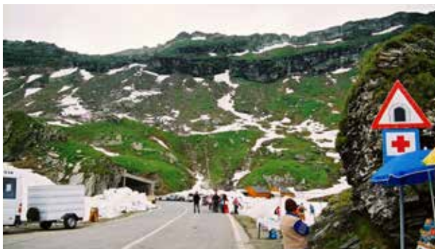
Fig. 6.37 In addition to traffic itself, accompanying human activities along roads increase the impact on sensitive mountain ecosystems. Connectivity should always be ensured by a sufficient number of tunnels. Transfăgărășan, Romania. © Blanka Dovrtělová
