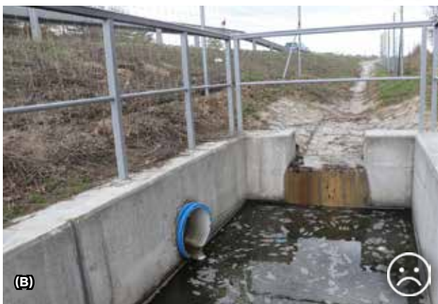
Fig. 9.17 A small retention reservoir becomes a trap for many small animals when water level drops. It would be suitable to design such reservoir as natural or at least with one inclined wall, so that escape of animals is possible. D1, Czech Republic. © Petr Anděl (A), Václav Hlaváč (B)
