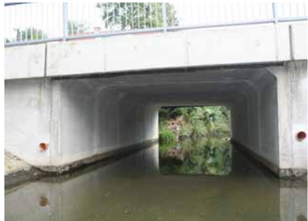
Fig. 4.4 A bridge without dry banks creates 'psychological barrier' for otters, although they are physically able to swim through such a bridge. Experience shows that most otters do not use such underpasses and cross the road instead. © Václav Hlaváč
