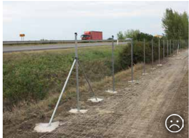
Fig. 9.24 High vegetation between a motorway and a fence attracts animals, because it is often the only vegetation in intensive agricultural land. If the fence is damaged, animals can easily be trapped between the fence and the motorway. Likewise, the fence behind trees is not visible from the motorway, so damage is not detected and repaired in time and the risk of collisions between cars and animals is even greater. © NDS Archive
