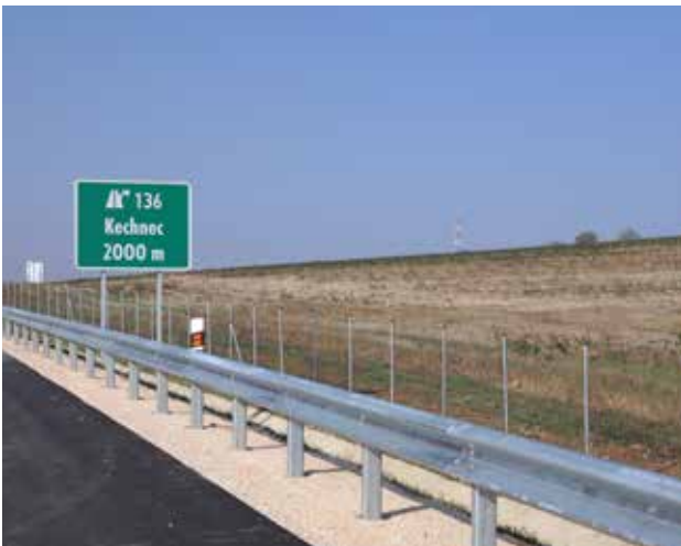
Fig. 9.20 Fences in general prevent animal mortality but increase barrier effect of the infrastructure. © NDS Archive
