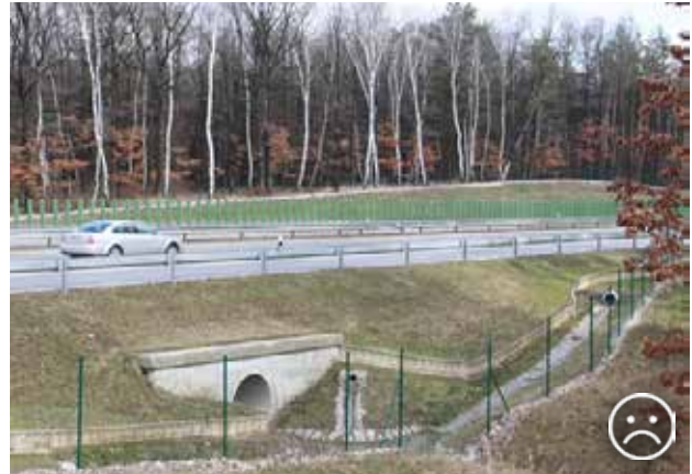
Fig. 10.45 If the entrance into a culvert is on one roadside outside of a fenced area and on the other roadside inside of the fenced area, animals using such an underpass stay trapped between the fences and the road. In case both entrances are inside a fenced area the underpass cannot be used by animals at all. © Václav Hlaváč
