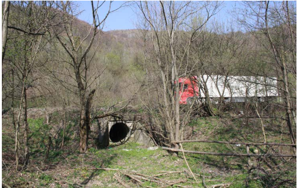
Fig. 64: The culvert under the road Mukachevo - Nyzhni Vorota., 2018.
