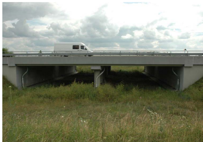
Fig. 32: The underpass zone of valley-bridge in summer season. Author: Zoltán Ilonczai
