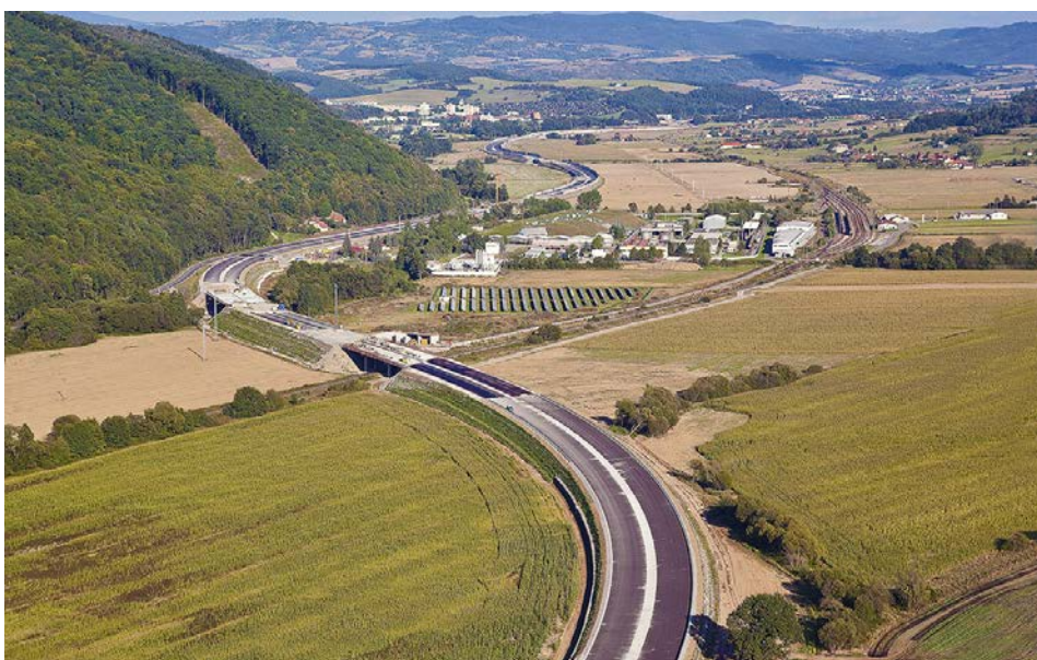
Fig. 34: View on the dual carriageway R2 from the village Pstruša onward.
