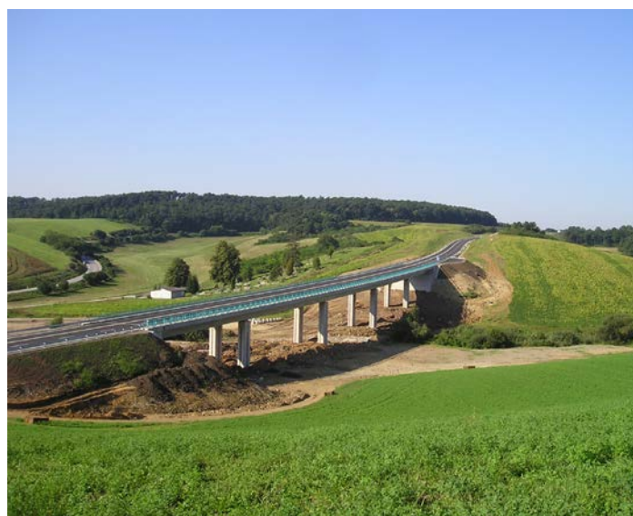
Fig. 33: Viaduct near the village Figa. Source: NDS
