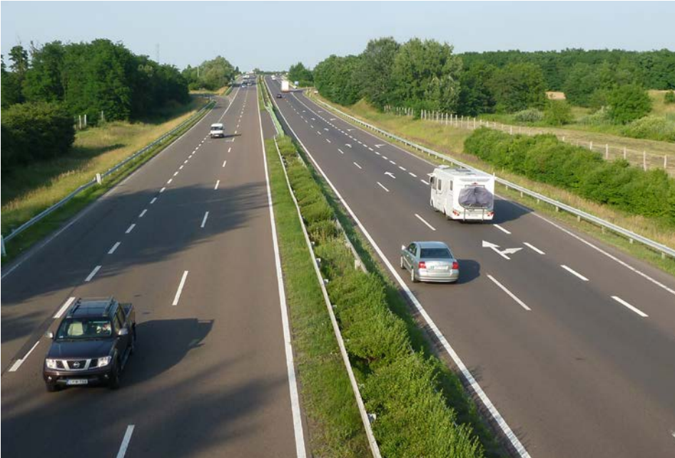
Fig. 8: Mitigation measures are so much more important due to ever increasing traffic intensity.
