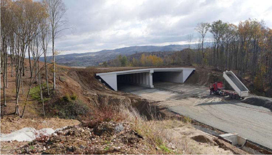
Fig. 7: Green bridges being built on the section 3 of the Lugoj-Deva motorway needs to be integrated into landscape through a local management plan aiming to ensure the functionality of these critical passage points.
