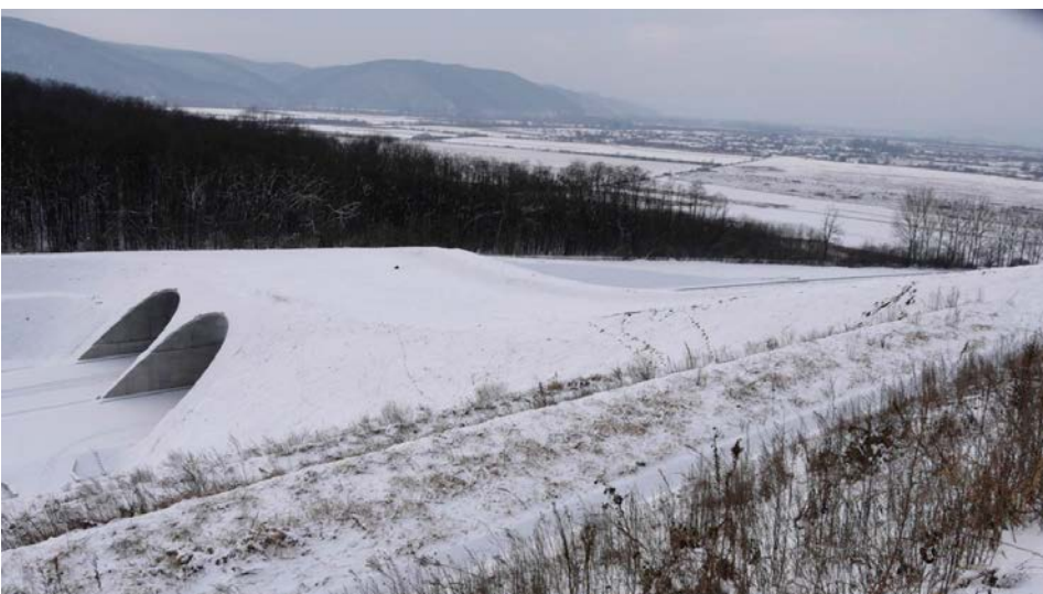
Fig. 8: In order to ensure its functionality, an extension of the Branisca green bridge needs to mitigate the adjacent county road and to lead the animals to/ from the forested area.
