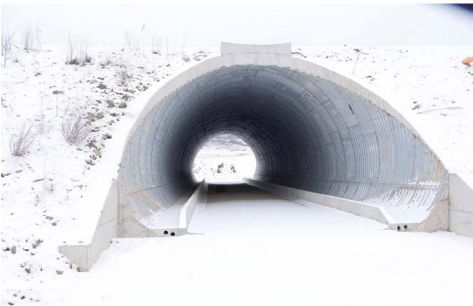
Fig. 3: A large rectangular passage included in the initial technical plan was changed into a semi-circular, reduced in size object, diminishing drastically its potential use for wildlife.
