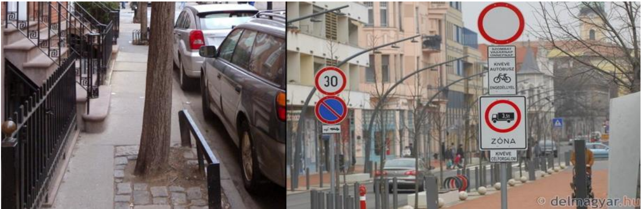
16 Inadequate pedestrian infrastructure and traffic signs
