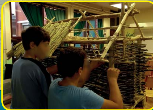
Pupils had to weave the wattle around the main structural elements of the house, its two sides, the front and the end
