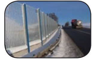
NOISE PROTECTION WALL SECURED FROM BIRD COLLISIONS
