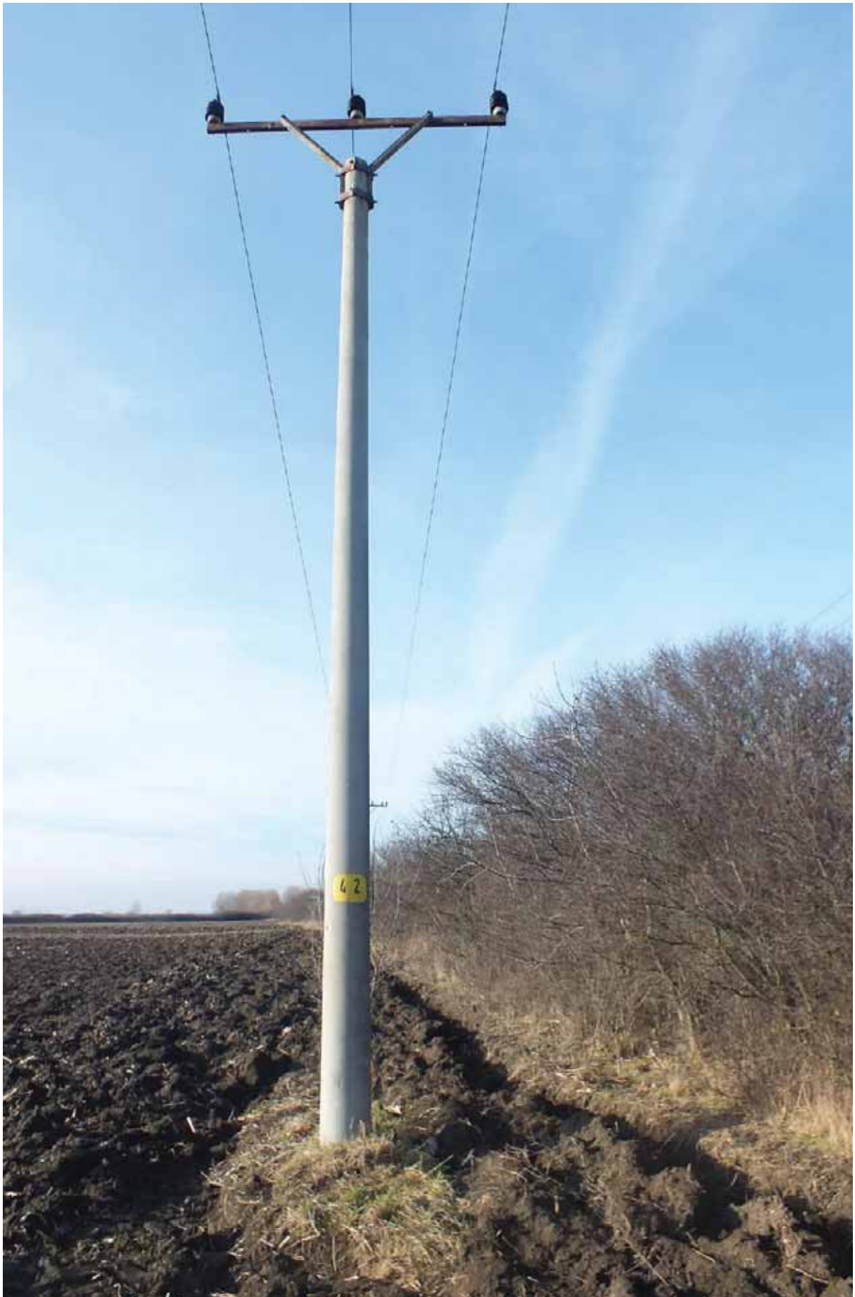
Fig. 5: Medium risk: Electric pole with a vertical position of support insulators on console. © Raptor Protection of Slovakia
