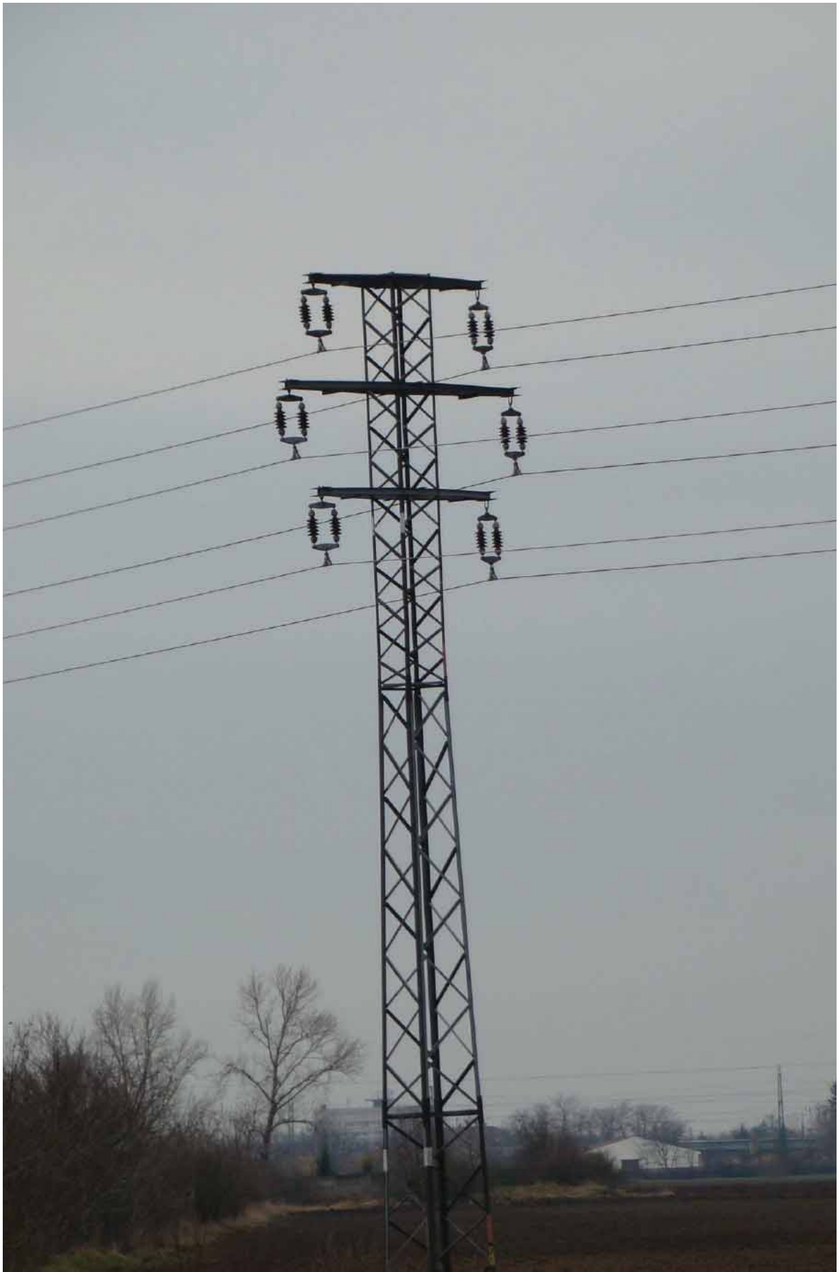
Fig. 11: Low risk: Double circuit electric pole with hanging insulators. © Raptor Protection of Slovakia
