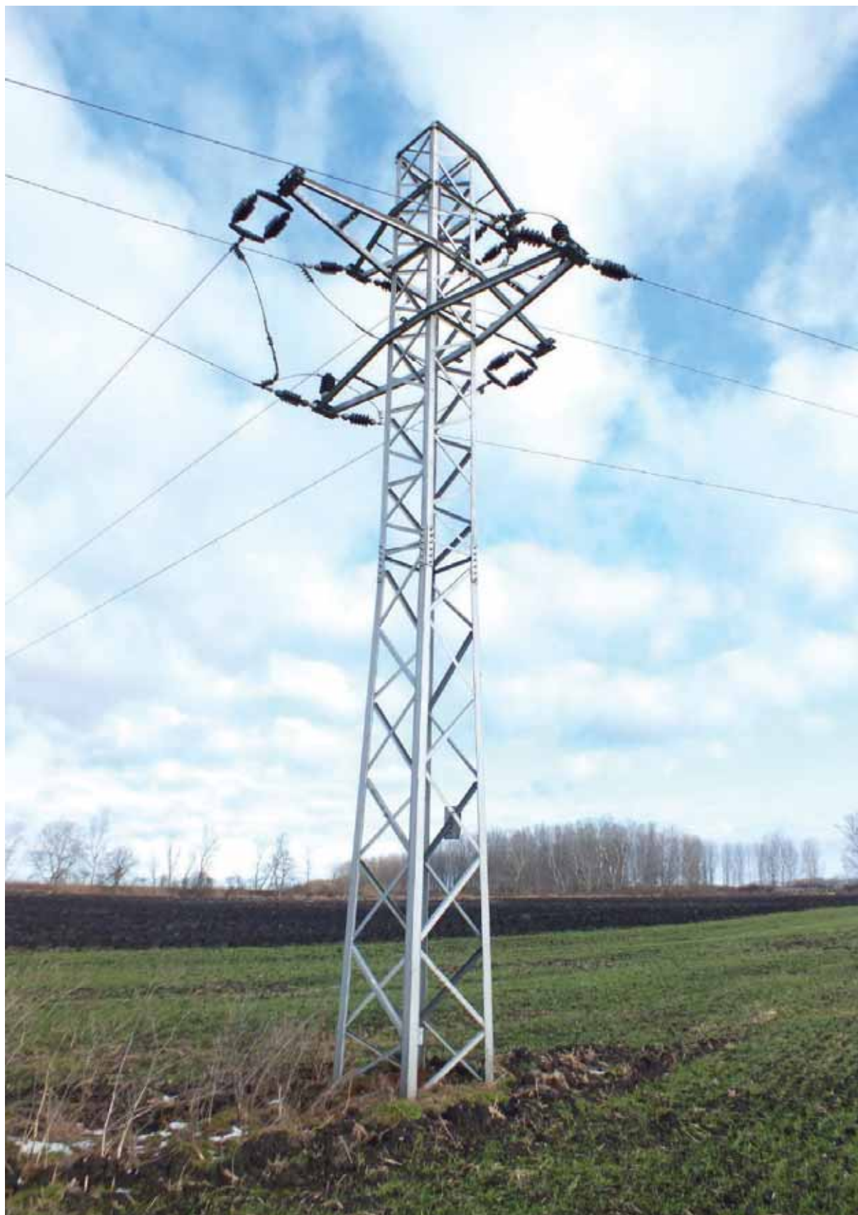
Fig. 1: High Risk: Metal cross-arm pylon with a combination of support insulators and exposed jumper wire locations. © Raptor Protection of Slovakia
