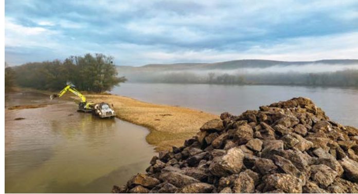
River revitalisation in three steps: an island side arm in Austria has undergone restoration by removing nearly 6,000 tonnes of groynes. The revitalisation supports the improvement of water discharge and sediment transport by enabling water continuity, and will play an important role in the preservation of the character of this island in the long term.
