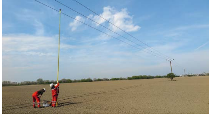
Power line marking in three steps: a very critical medium-voltage power line was marked in Slovakia. These measures were very simple and quick to implement.
