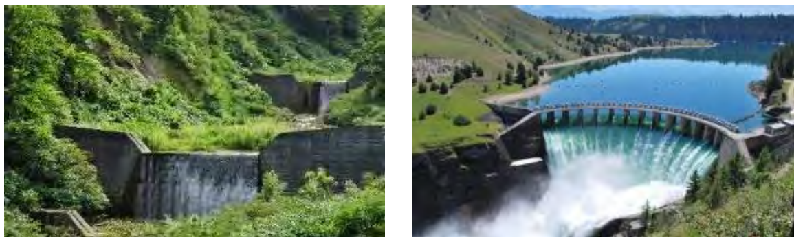
a) Weir for river bed stabilisation on a small river
