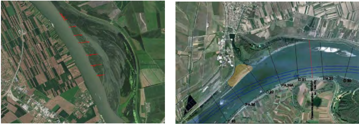
Figure 5.1.124 a) Groyne field built 10 km upstream of the Sava River's mouth; b) T-shaped groyne built at rkm 1,108+500 of the Danube (upstream of the Kovin winter shelter)
