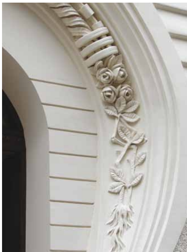
6. 20 Đorđićeva Street: Stucco decoration around the main entrance, after the restoration
