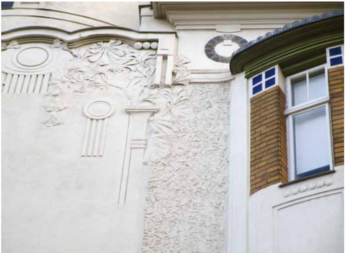
6.a-b Emil Reitmann, "Galileihof", 3-5 Lainzer Straße, 1130 Vienna, 1905, before and after renovation
