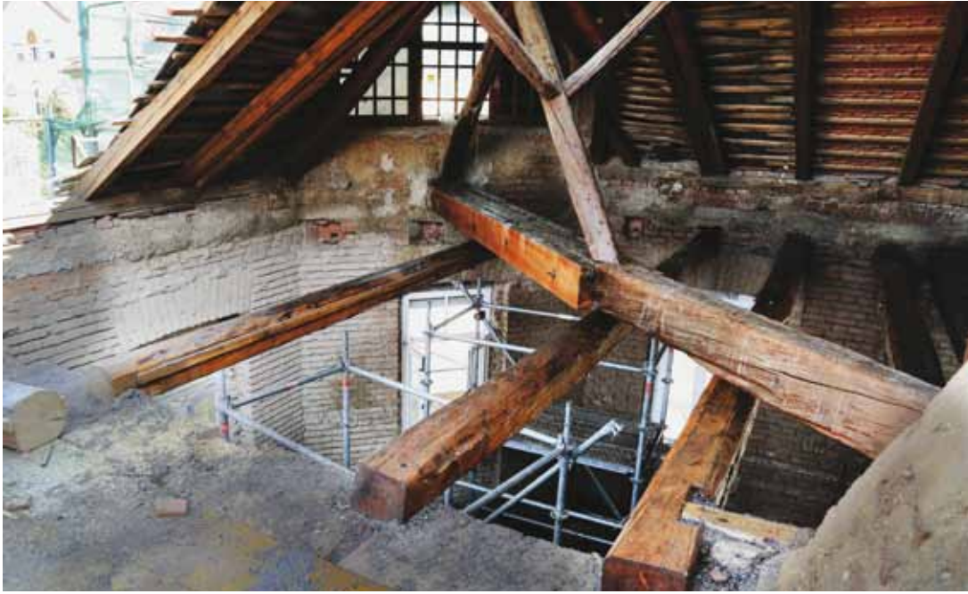
7. The edge of the roof structure
