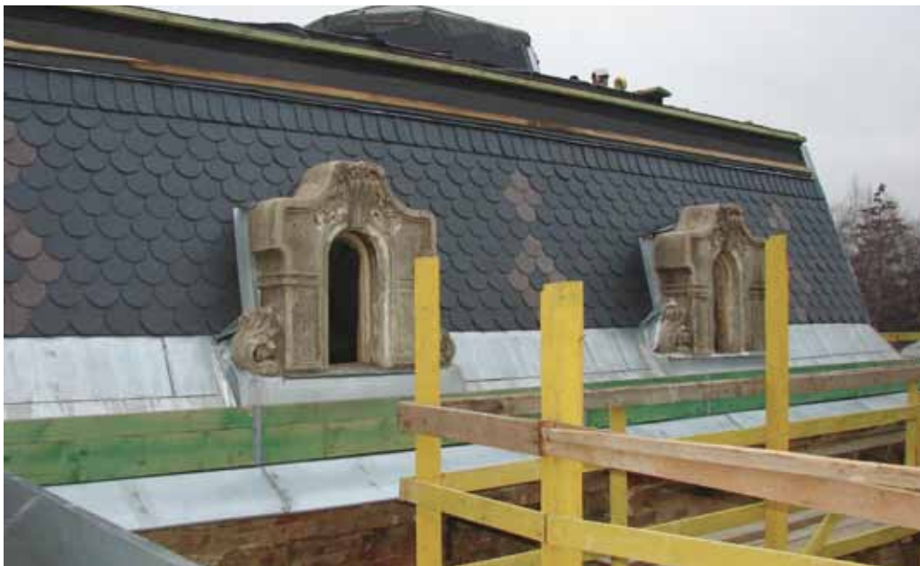
2. The Sofian House, Botoșani, roof restoration, 2016
