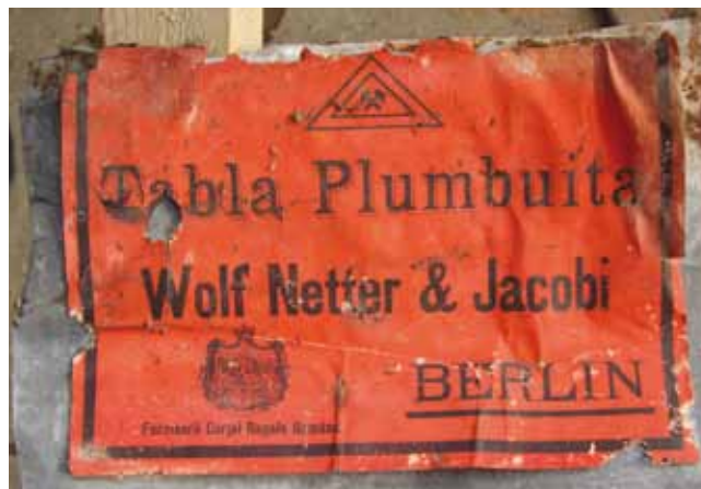
3. The Sofian House, Botoșani, original zinc sheet with the producer’s mark
