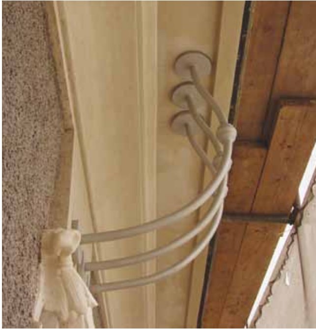
7. 20 Đorđićeva Street: Reconstructed metal pipe under the roof
