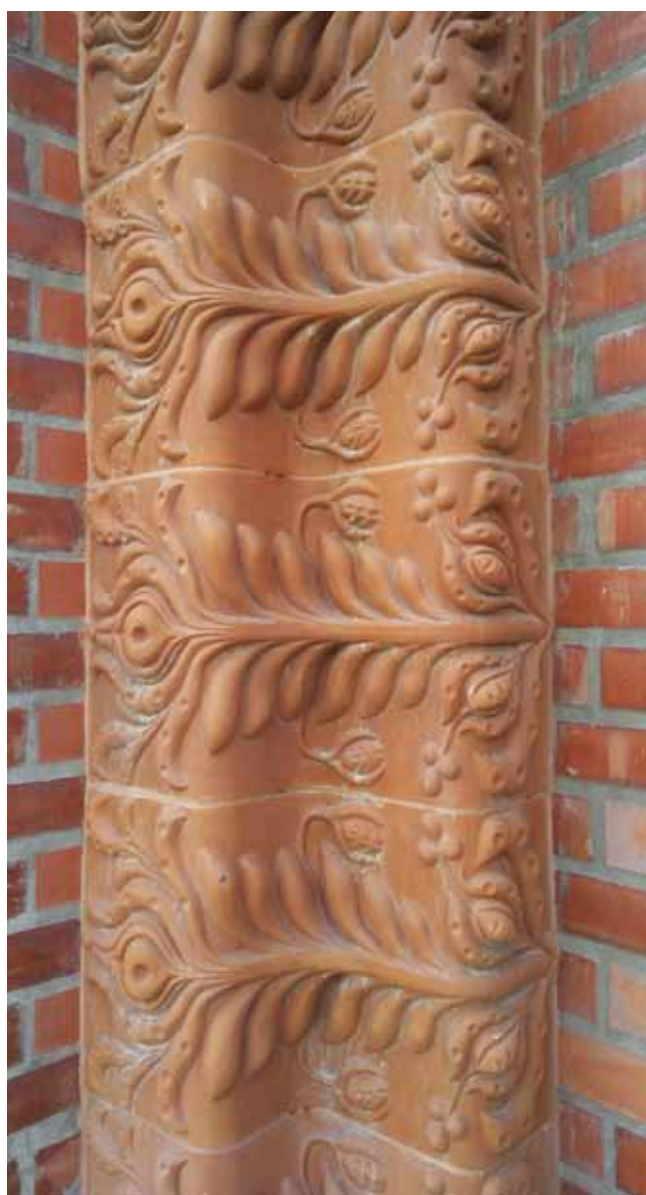
1. Detail of the terracotta on the synagogue's entrance portal
