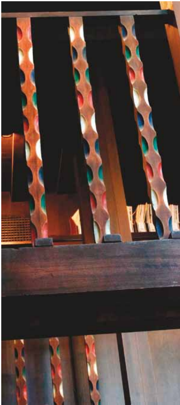
8a-b Detail of chamfered spindles, Mackintosh Library balcony (left: pre-fire c. 2012; right: Laurence McIntosh prototype model, 2017)
