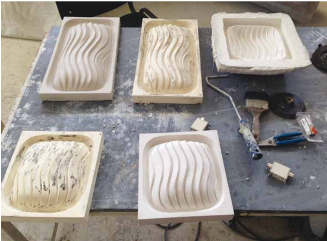
13. 80 Palmotičeva Street: Remodeled stucco elements of the windows during the restoration
