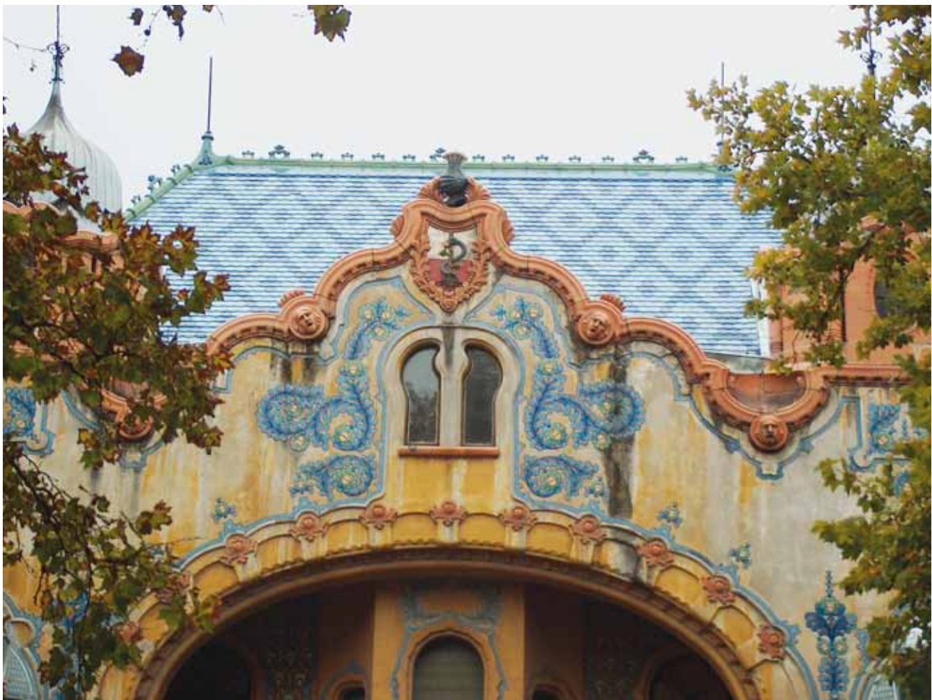
7. Detail of the roof after restoration
