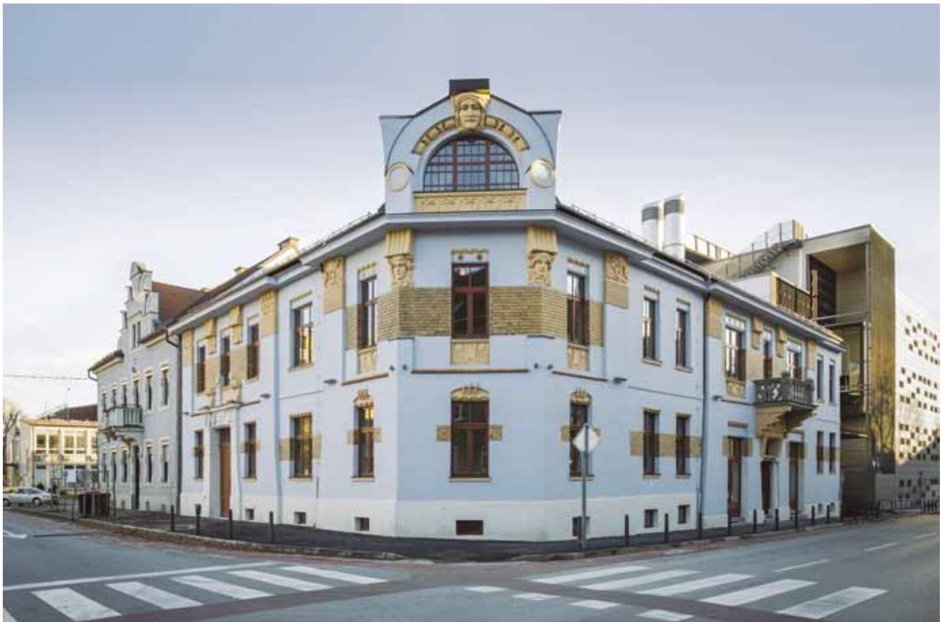
1. The Baroness house after the renovation, 2015
