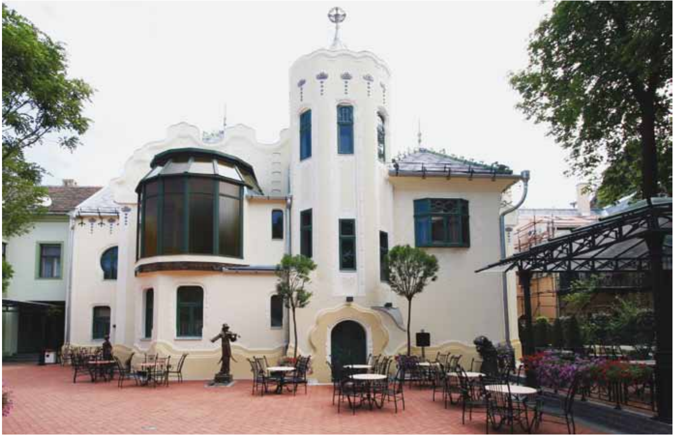
11. The courtyard façade after reconstruction and restoration
