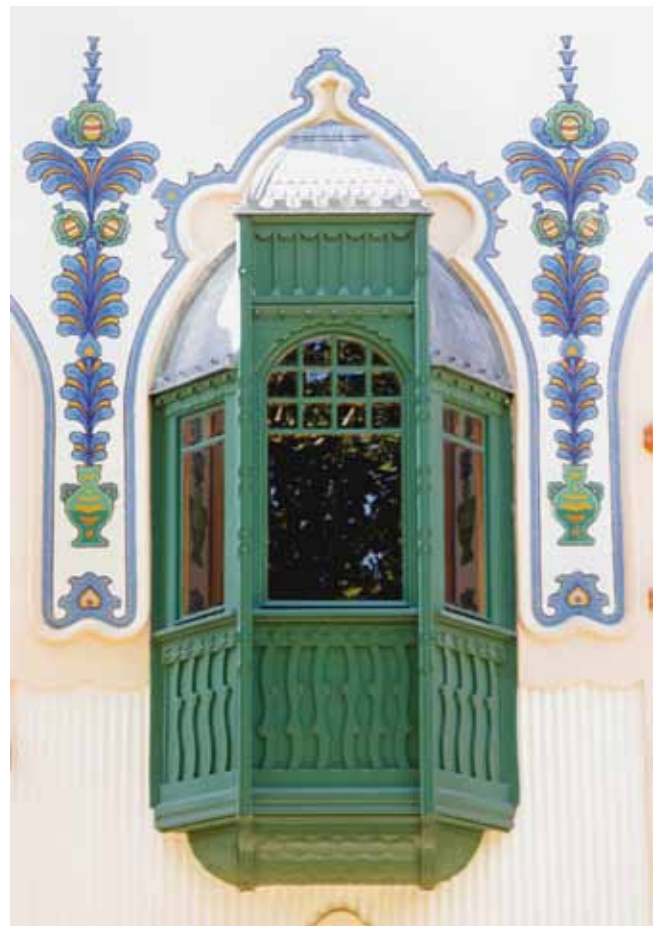
4. An oriel window after the restoration
