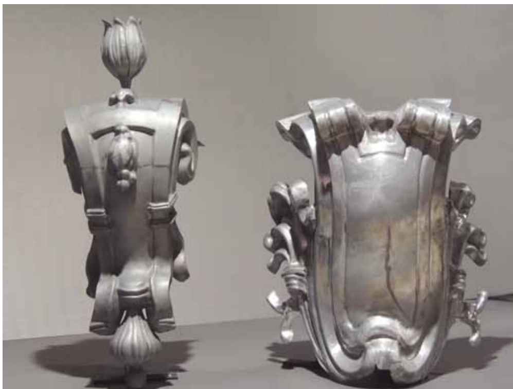
6. The Sofian House, Botoșani, Art Nouveau roof ornaments replicated from titanium zinc sheets, 2016
