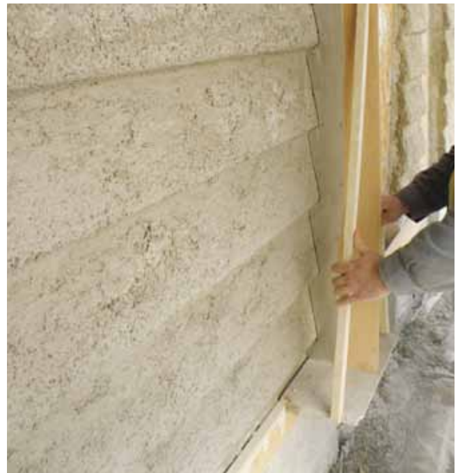
4. 20 Đorđićeva Street: Recreating the special plaster surface
