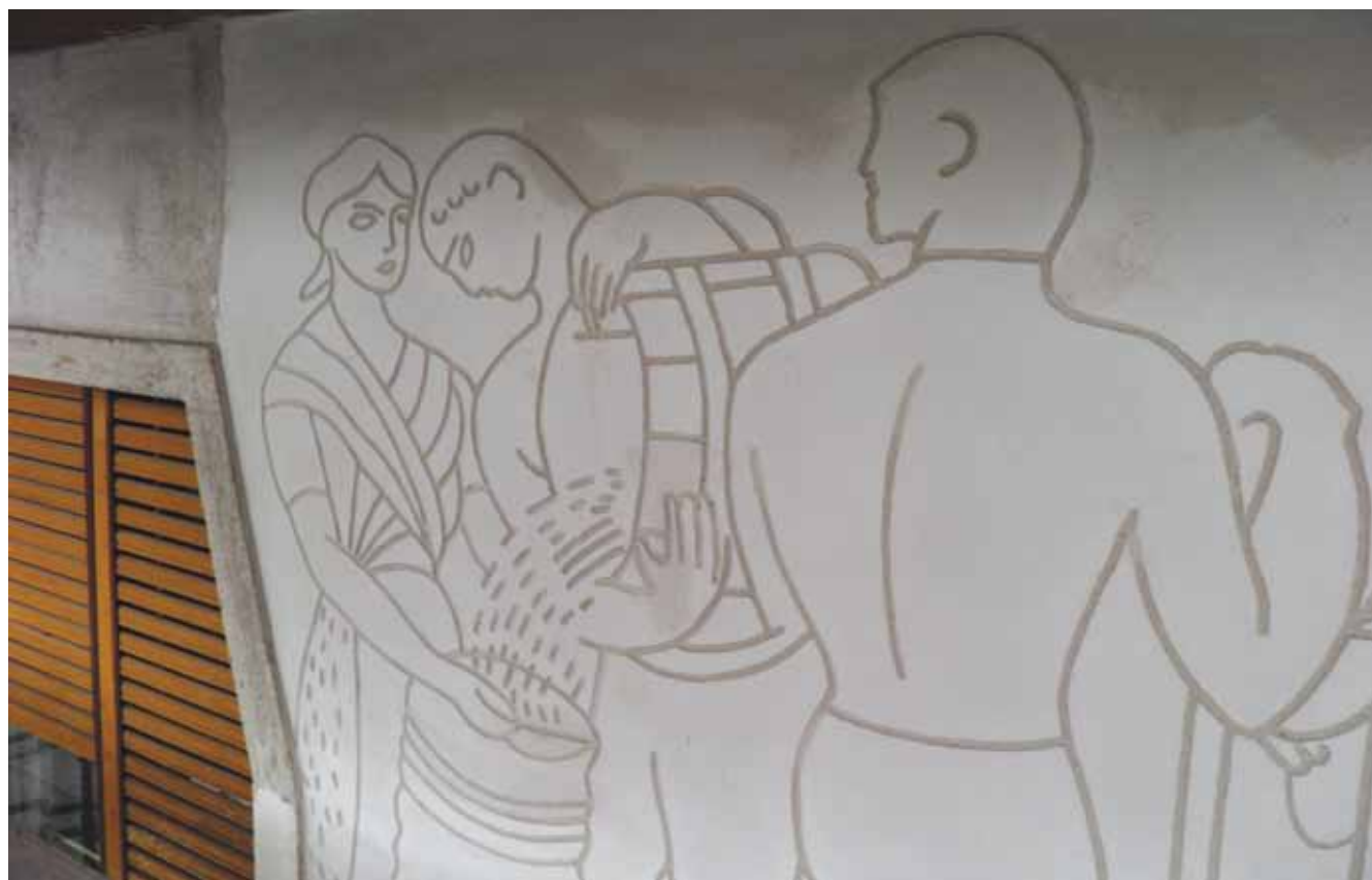
13. Adolf Moskovits Palace, sgraffito, after restoration
