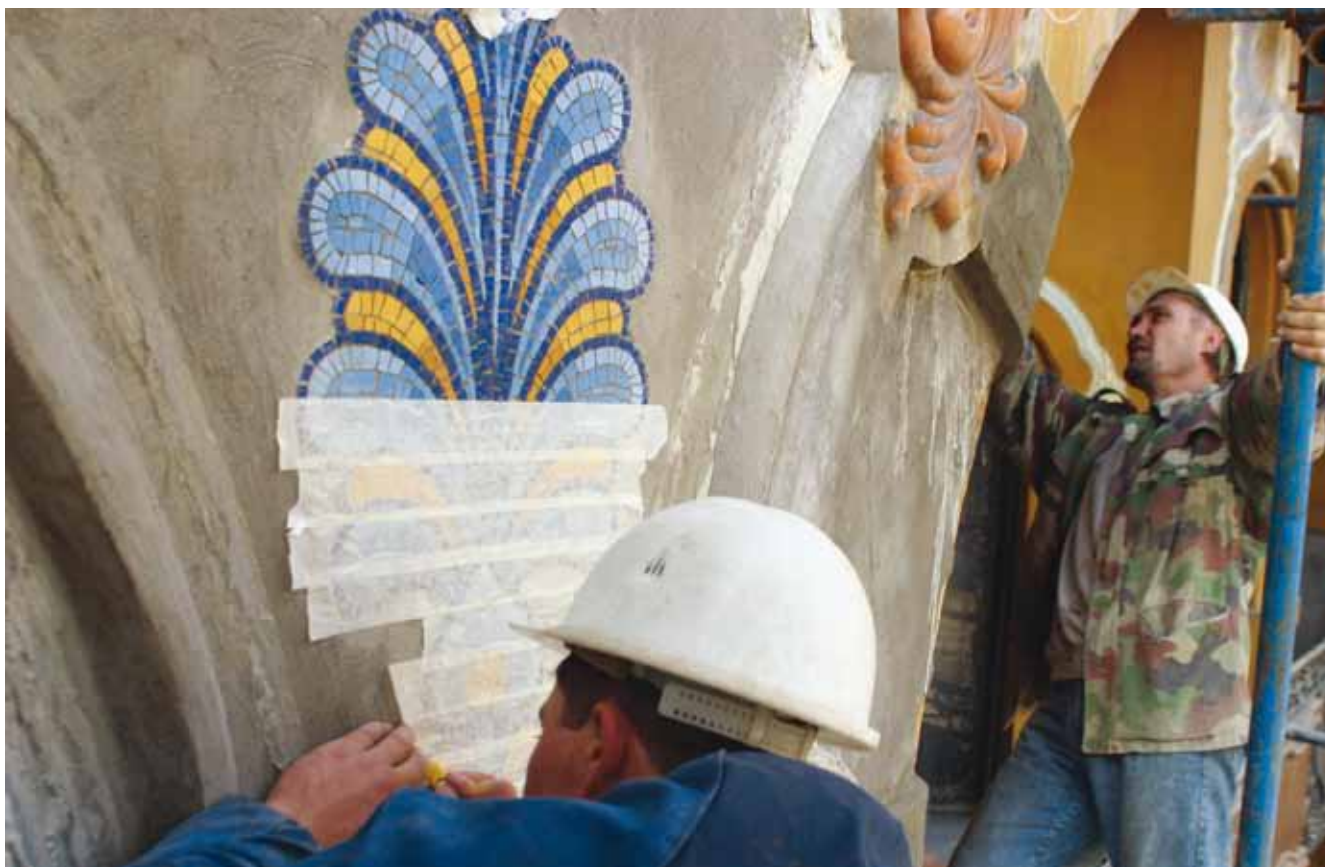
14. Façade restoration work
