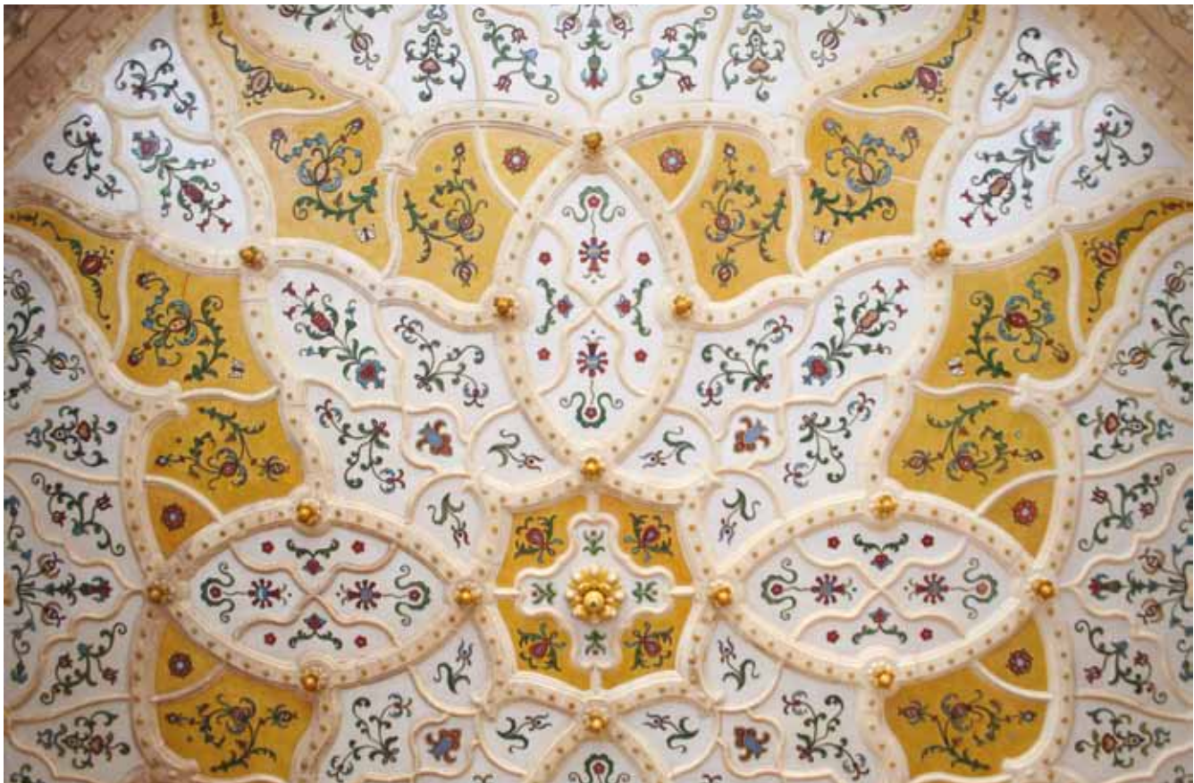
13. The ceiling in the main entrance after restoration
