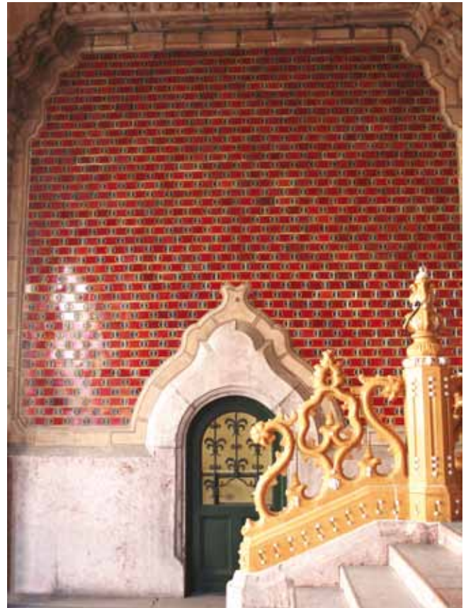
9. The wall covered with ceramics after their conservation and reinsertion
