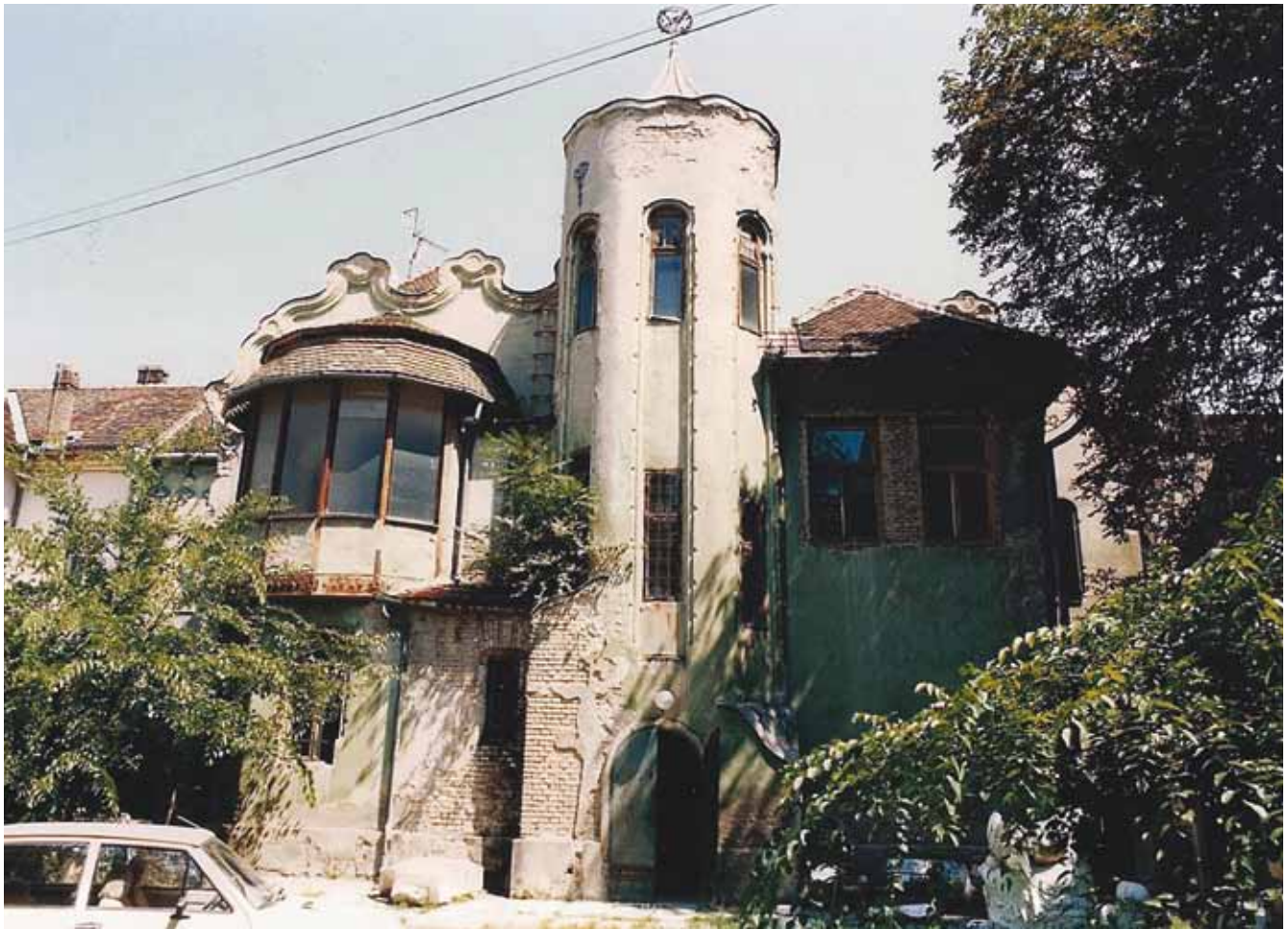
8. The courtyard façade before restoration
