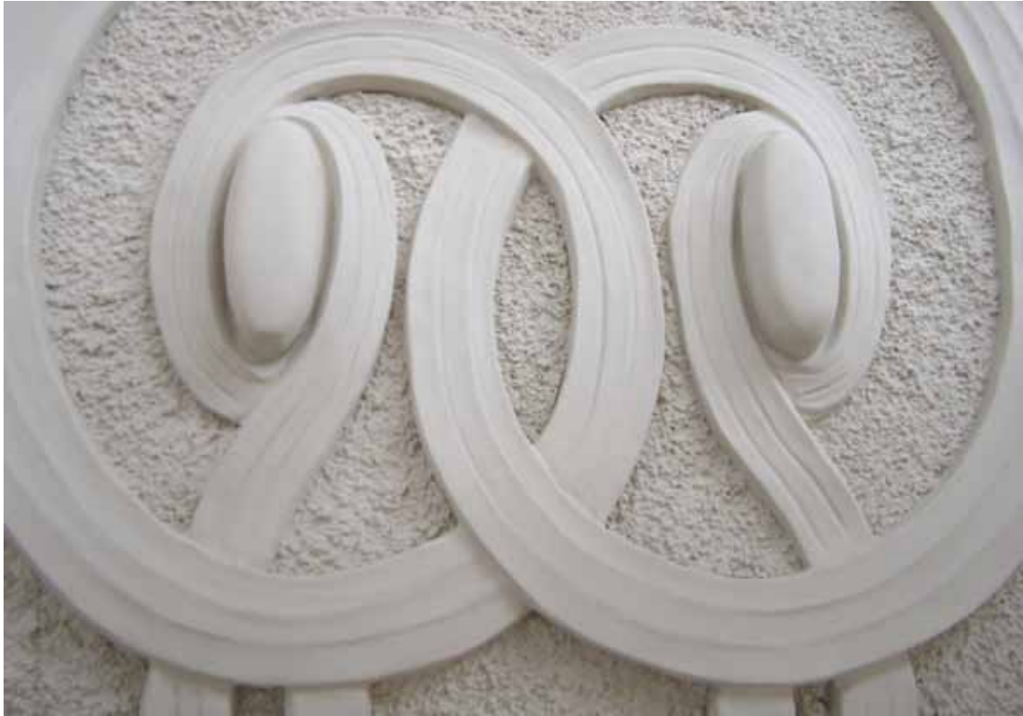
12. 80 Palmotičeva Street: Remodeled stucco elements after the restoration
