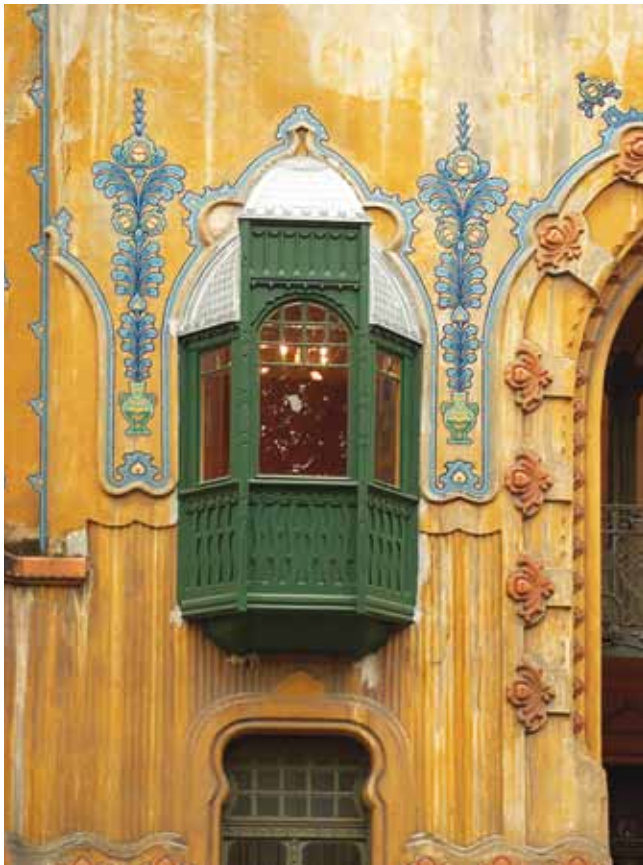
3. An oriel window before the restoration
