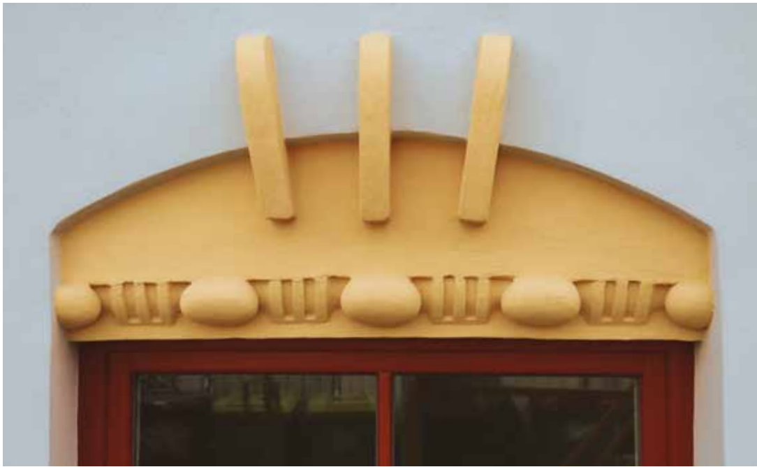
5. The façades and individual details are entirely decorated in the Art Nouveau style
