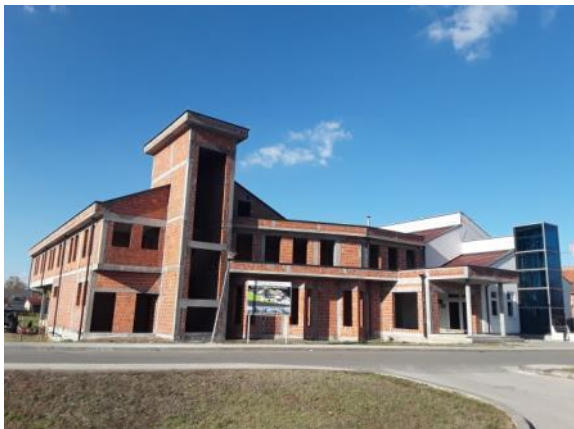
5) Domaljevac Spa - under construction
