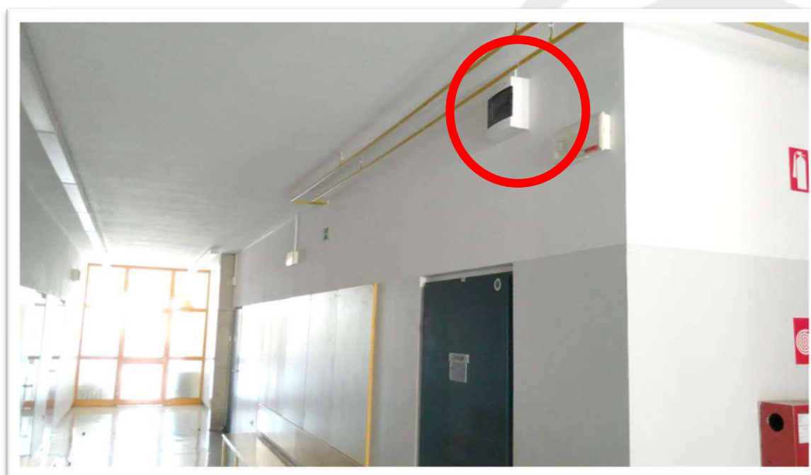
Gateway in the first floor hallway
