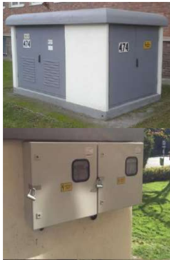
LV measurement in MV/LV Tr. St. Kossuth u.
