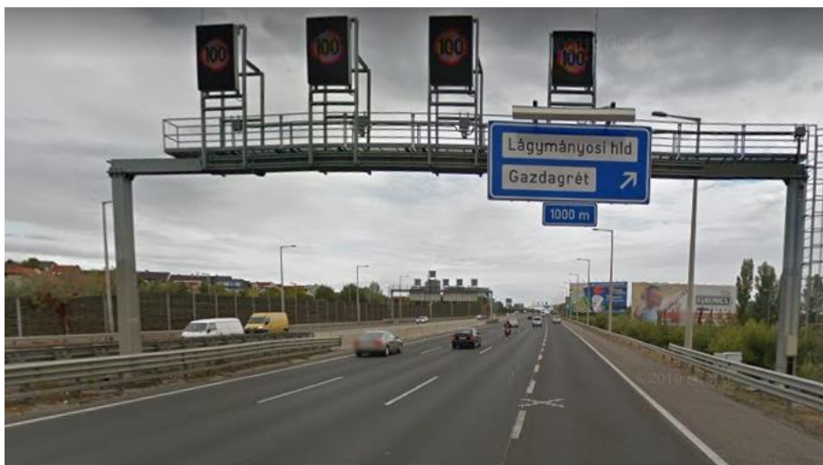
Figure 8. Example of variable speed limit (M1-M7 motorway, Hungary)
