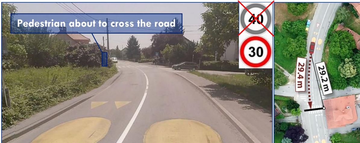
Figure 6: Inadequate visibility in the curve
