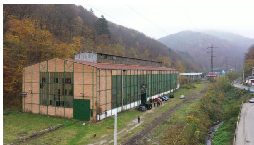
Figure 4. Hala Minda, piloting location (front view). Source: Reșița Municipality
