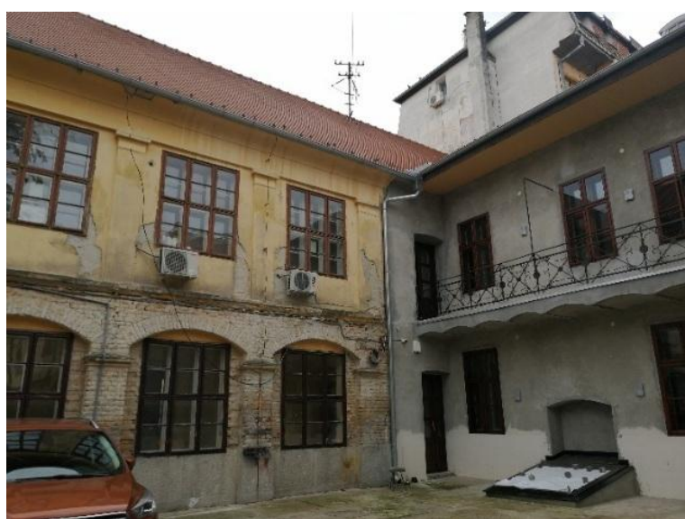
Figure 4. Sombor, Grašalković palace, sections currently in use. Source: City of Sombor
