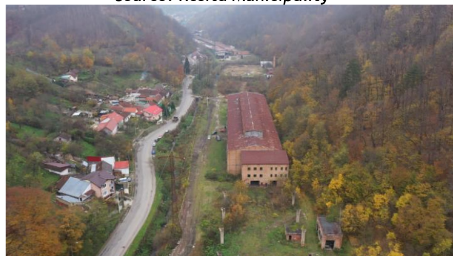
Figure 5. Hala Minda, piloting location (upper view). Source: Reșița Municipality
