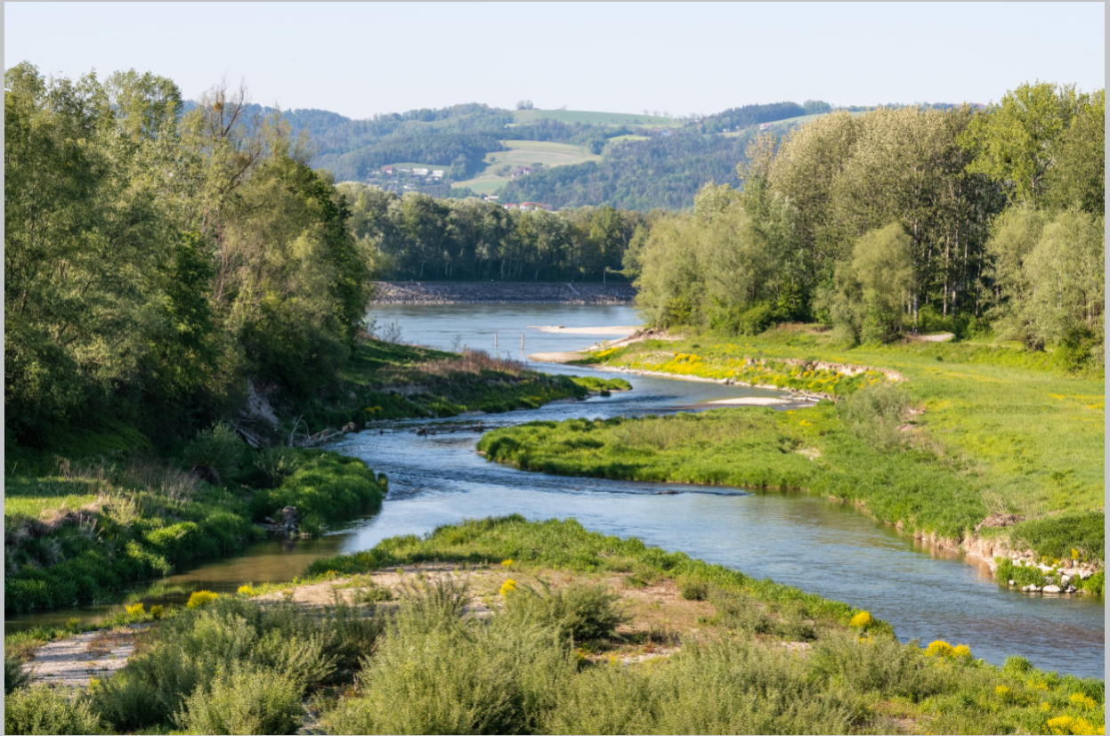
Figure 6: At the hydropower plant Ottensheim-Wilhering in Austria, the Austrian hydropower company VERBUND built in recent years a more than 14-km-long bypass system with the support of a LIFE+ project. The bypass system fulfils the requirements of fish migration and also serves as a habitat. Such solutions are a first choice among migration facilities but they require sufficient place along a river section. When no place is available, e.g. in gorge sections, technical facilities might be an option (Photo: VERBUND 2020).
