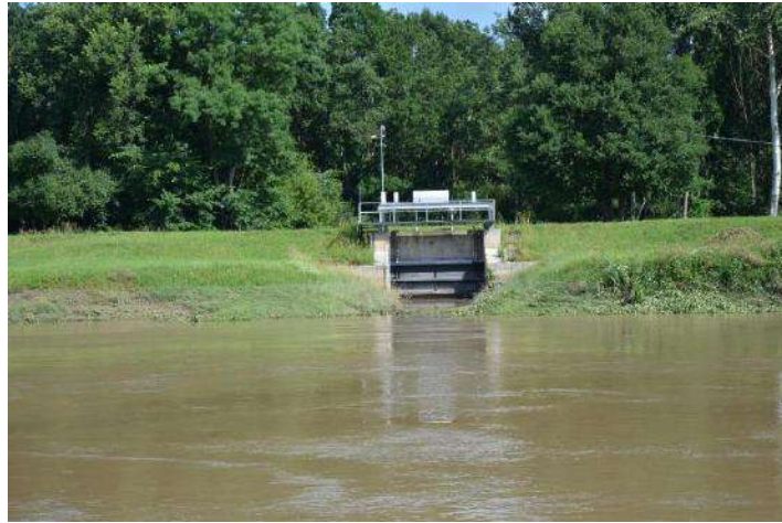
Figure 74: Inflow object to the retention area behind the flood protection dyke (Author: VUVH)
