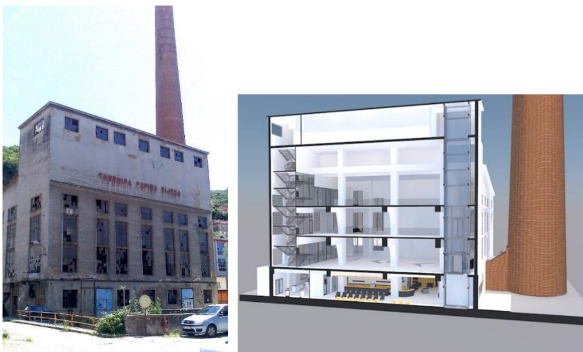
Picture 12. Existing condition of Energana building and Energana in 2023
