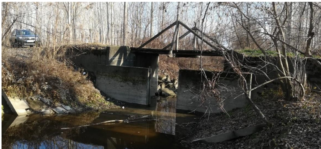
Figure 12 The sluice on Begej canal
