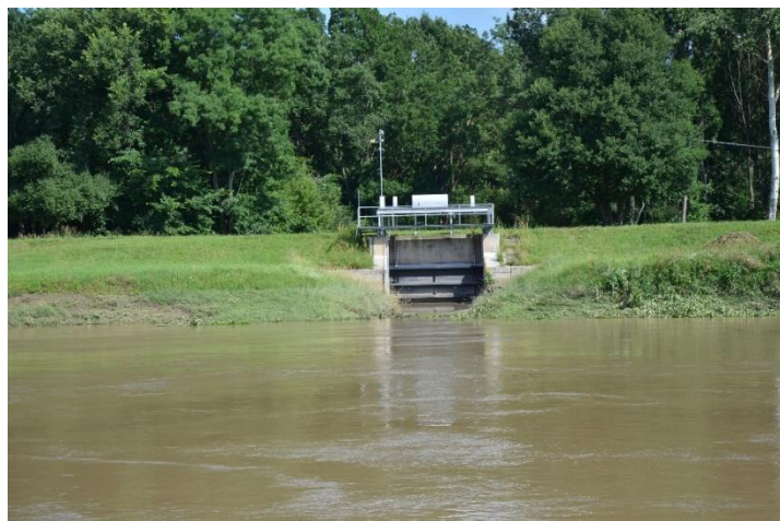
Figure 6: Inflow object to the retention area behind the flood protection dyke (Author: VUVH)
