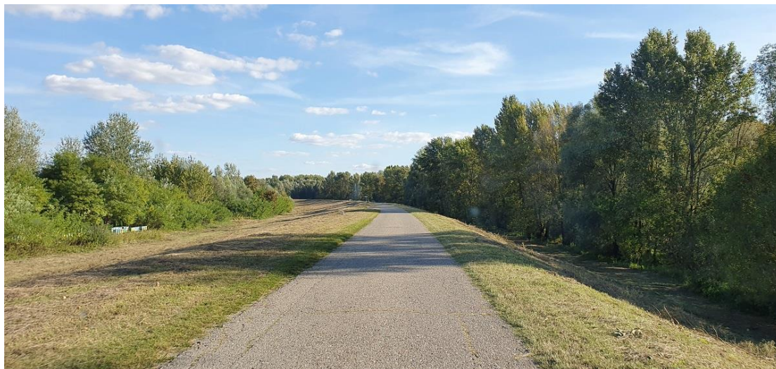
31. Figure: Embankment with asphalt road between Apatin and DTD canal
