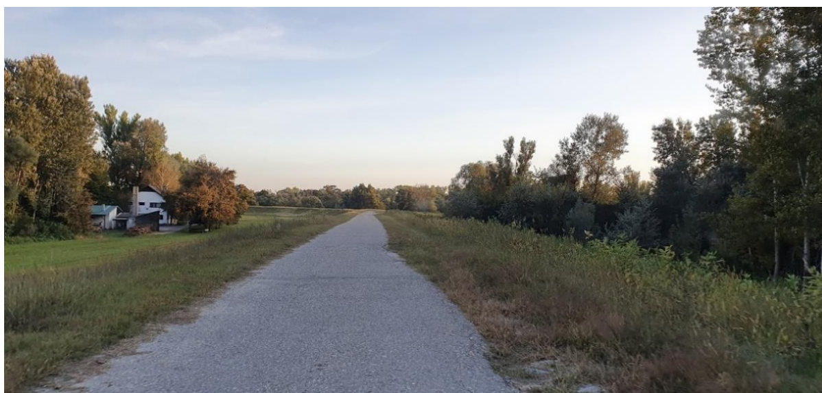
28. Figure: Paved surface on embankment at hunting house Mesarske livade
