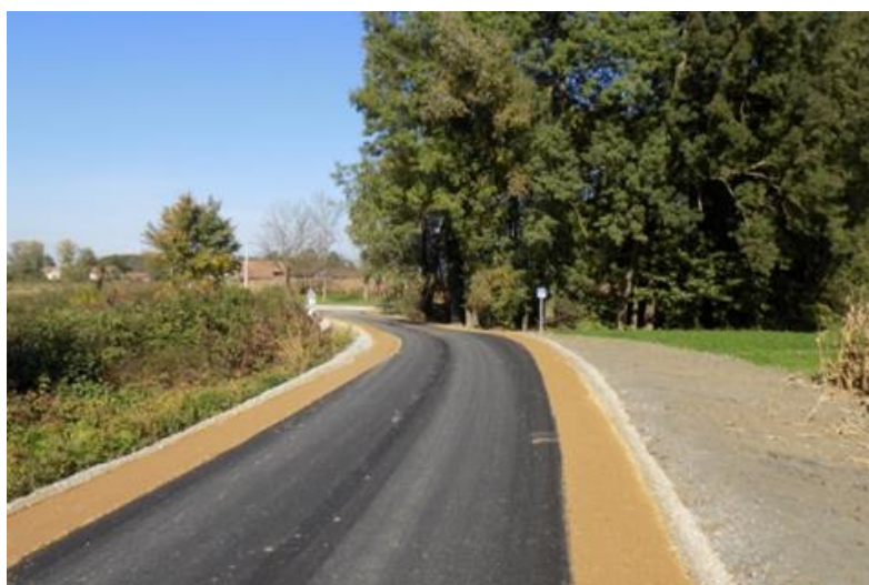
15. Figure: newly asphalted road in Novo Virje
