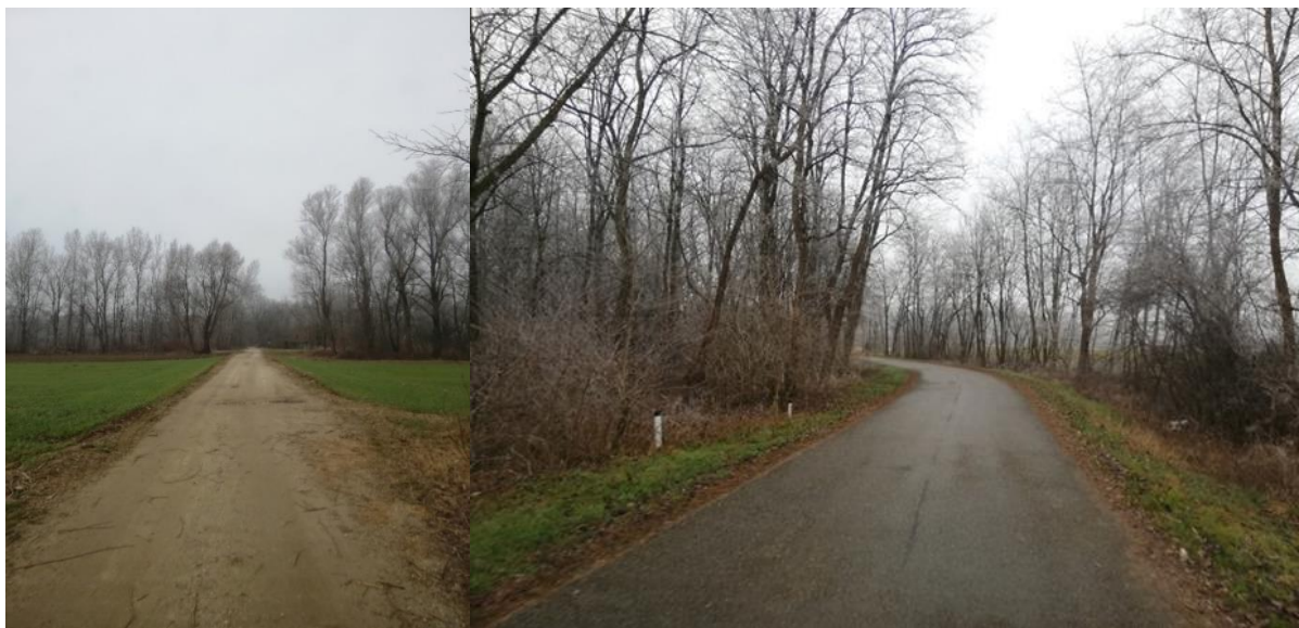
6-7. Figures: Unpaved and paved sections in good condition, south of Krog
