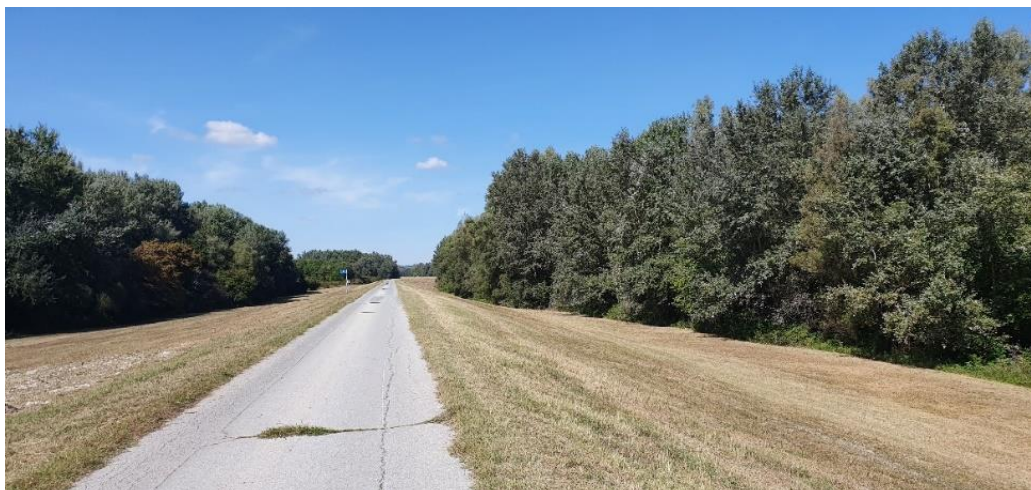
66. Figure: Asphalt part of the embankment north of Zlatna Greda
