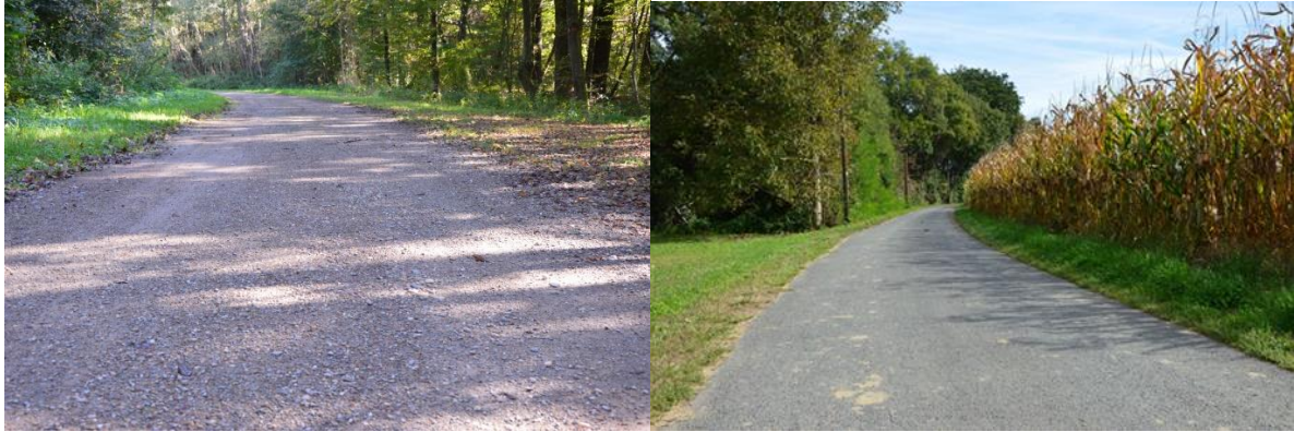
4-5. Figures: Well maintained gravel road near Murturm Tower; then turns into asphalt surface (between „Meinmühle“ and Dietzen
