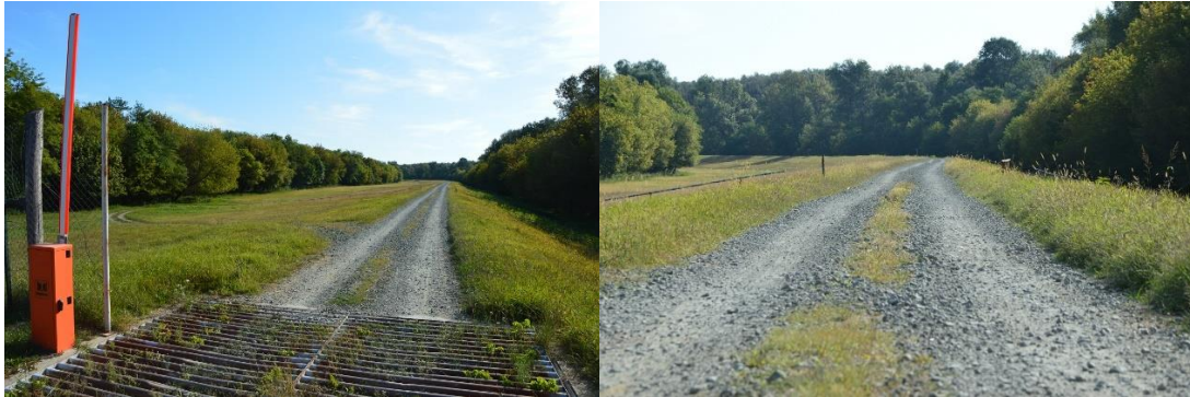
57-58. Figures: Start point of the gravel embankment road near Belišće
