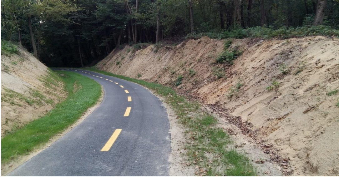
40. Figure: Barcs-Drávatamási, newly asphalt, under construction
