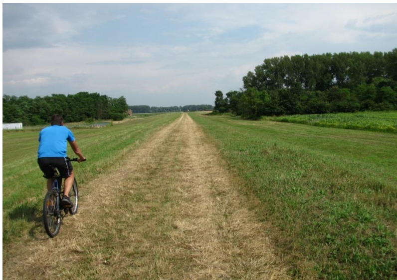
46. Figure: Mailáthpuszta-Szaporca dyke first part, dirt road
