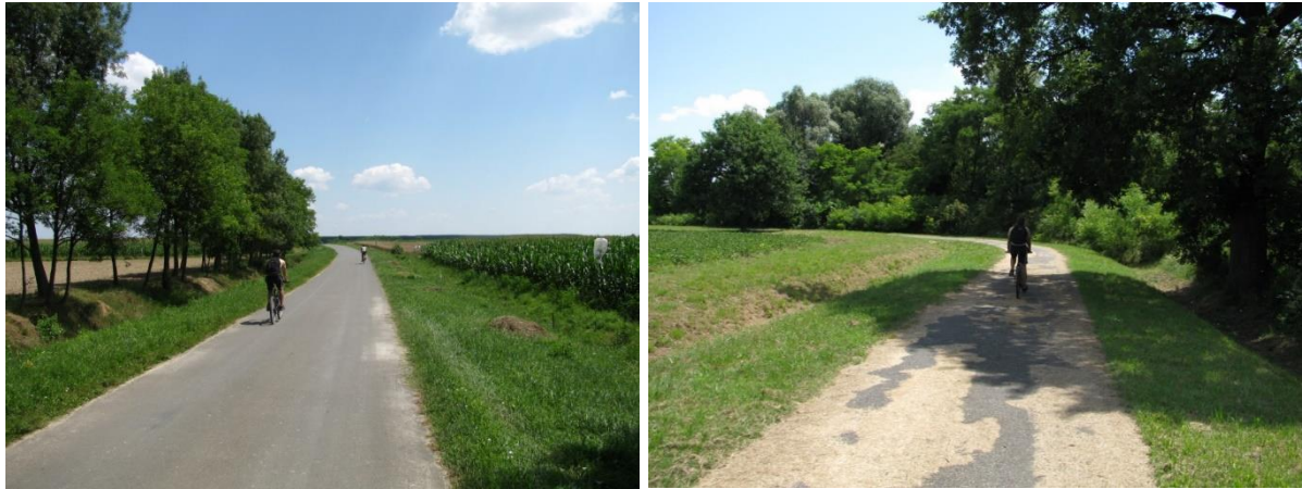
42-43. Figures: Leaving Drávatamási towards Drávagárdony on asphalt (left), Tótújfalu-Szentborbás dyke with asphalt road (right)
