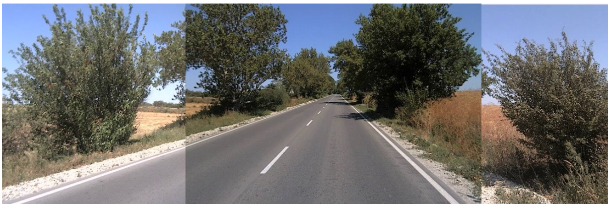
Figure 10 Dangerous objects (trees) on the section I-5
