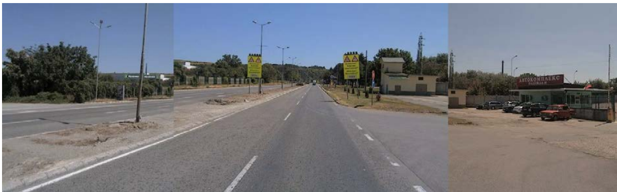
Figure 9 "Informal" intersection on the section I-5
