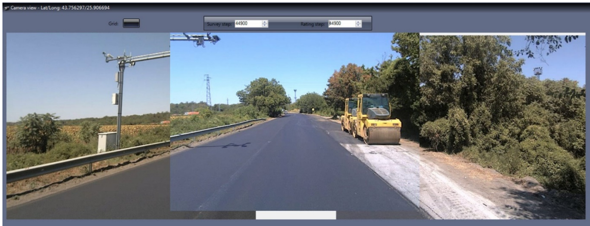
Figure 3 Road works on Road I-5
