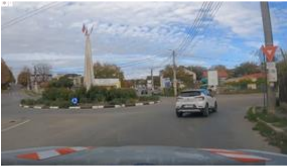
This roundabout in Tulcea, Romania, is lacking any markings (central, cycle path, lanes) and makes it very difficult to navigate by cyclists and drivers together.
