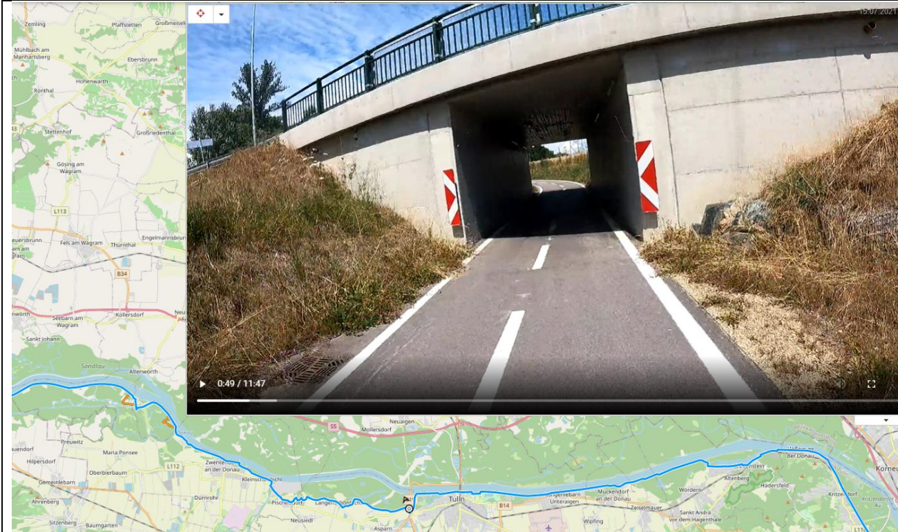
The image shows an underpass which has been constructed just recently. It is a good example for an underpass which is highlighted by two signs on the right and left side at the entry, as well as clear road markings. Moreover, the visual range is very good and allows to see oncoming cyclists in advance.
