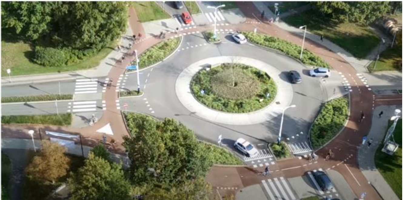
Figure 13: Segregation of two-way cycling facility and motor vehicle traffic on a roundabout in the Netherlands (Source: https://www.youtube.com/watch?v=FR5l48_h5Eo [23.02.2021])
