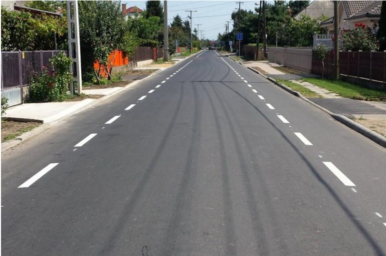
Figure 18: Advisory Cycle Lane in Hungary (Source: Danube Cycle Plans. Picture by jozsanet.hu)
