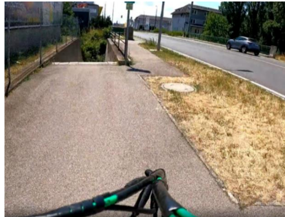
Poorly accessible underpass due to stairs at EuroVelo 9 in Austria
