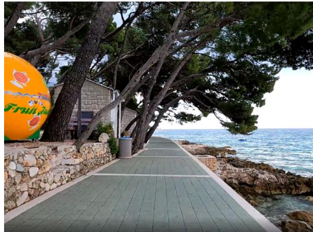
Mixed space of cyclists and pedestrians on the EuroVelo 8 in Croatia, typically with conflicts between walking and cycling tourists during summer
