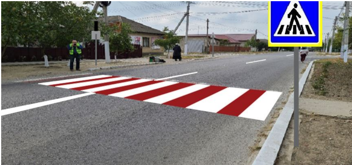
Picture 7-3 Congaz pedestrian crossing with traffic lights
