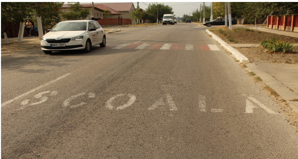
Picture 3-3 Faded markings
