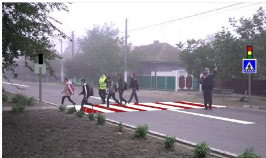
Picture 7-2 Congaz pedestrian crossing with traffic lights
