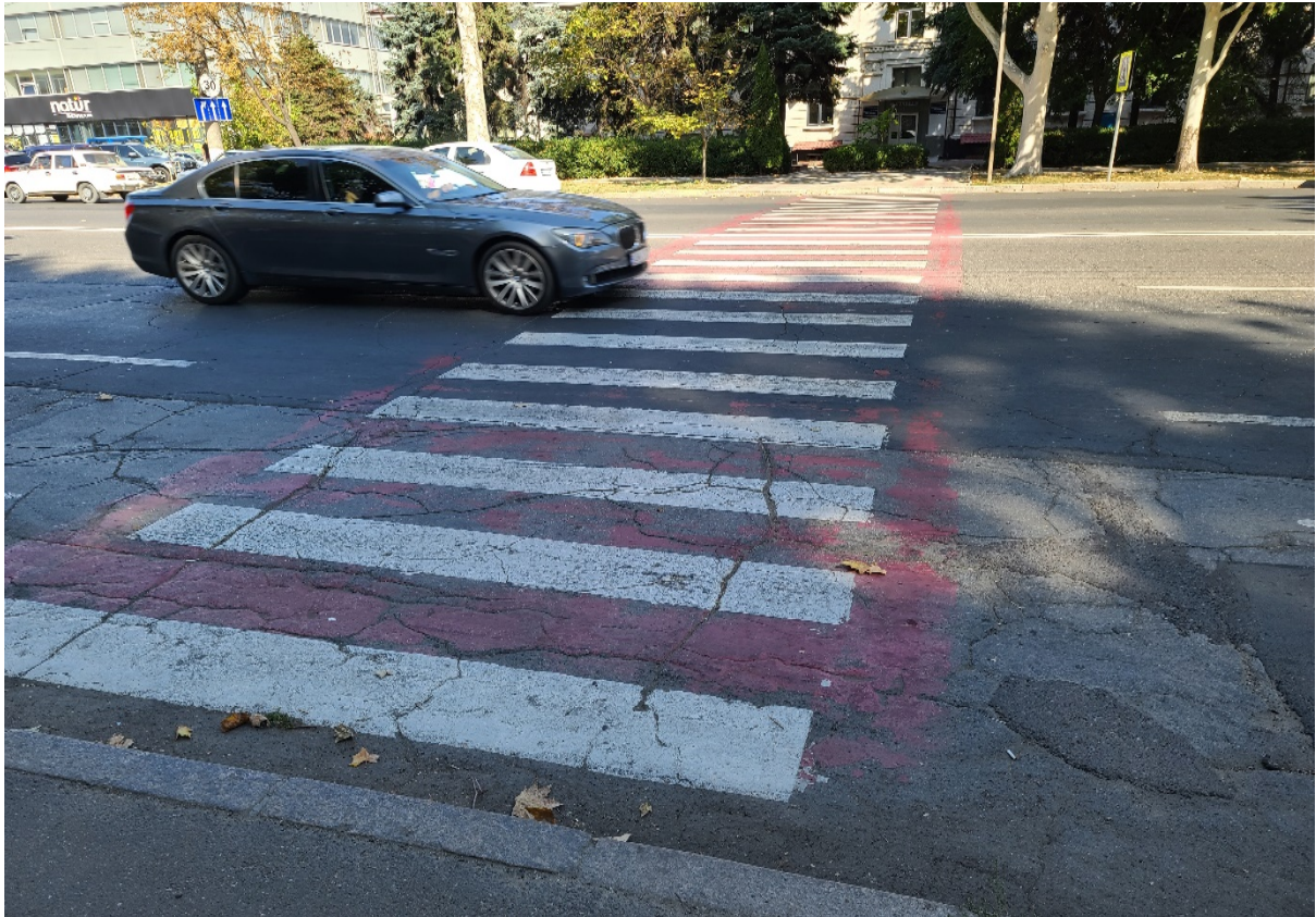
Picture 3-6 The painted pedestrian crossing after one month
