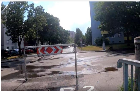
Railing as obstacle at EuroVelo 14 in Austria
