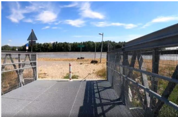
Bollard in the middle of the cycle path at Eurovelo 6 in Austria
