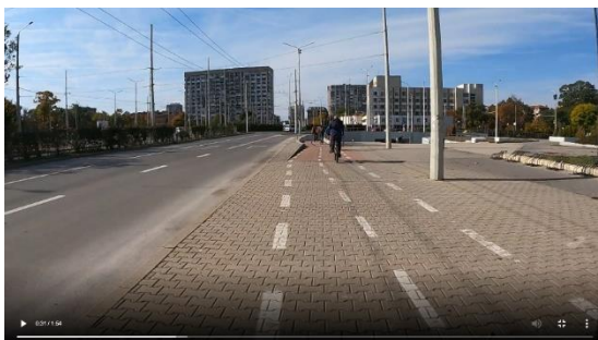
Pedestrian and bicycle lane along the roadway in Ruse, Bulgaria: The lanes are wide enough and do not cross with pedestrians
