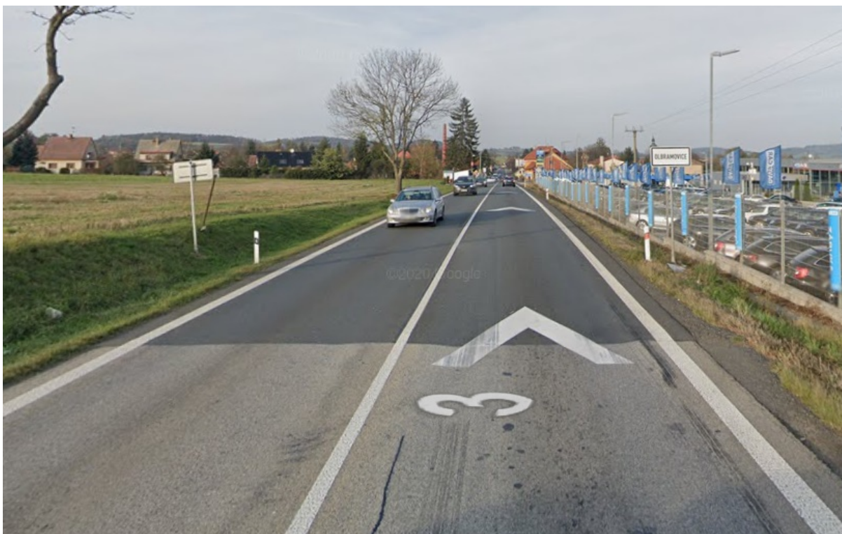
Figure 54 – South entrance to Olbramovice – no physical entry measures, speed limit signs 90-80-60-50 km/h, 13 “safe distance” road marks
