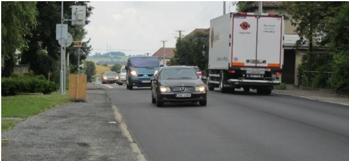
Figure 45 – 1/3 through road in Olbramovice – section with sidewalks on both sides, but levelled wit road surface due to numerous surface treatments
