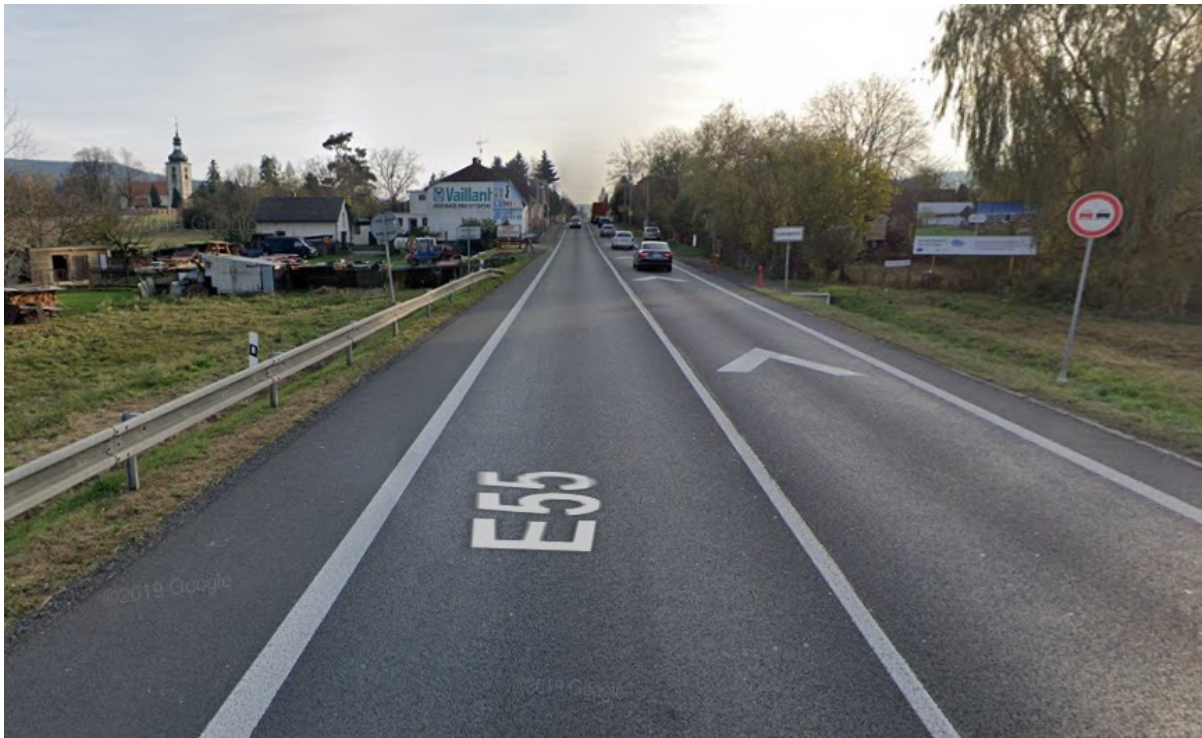
Figure 53 – North entrance to Olbramovice – no physical entry measures, 12 “safe distance” road marks
