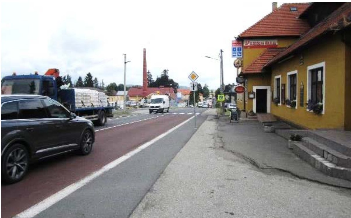
Figure 50 – 1/3 through road in Olbramovice – pedestrian crossing highlighted by coloured road surface but pedestrian facilities levelled with road surface
