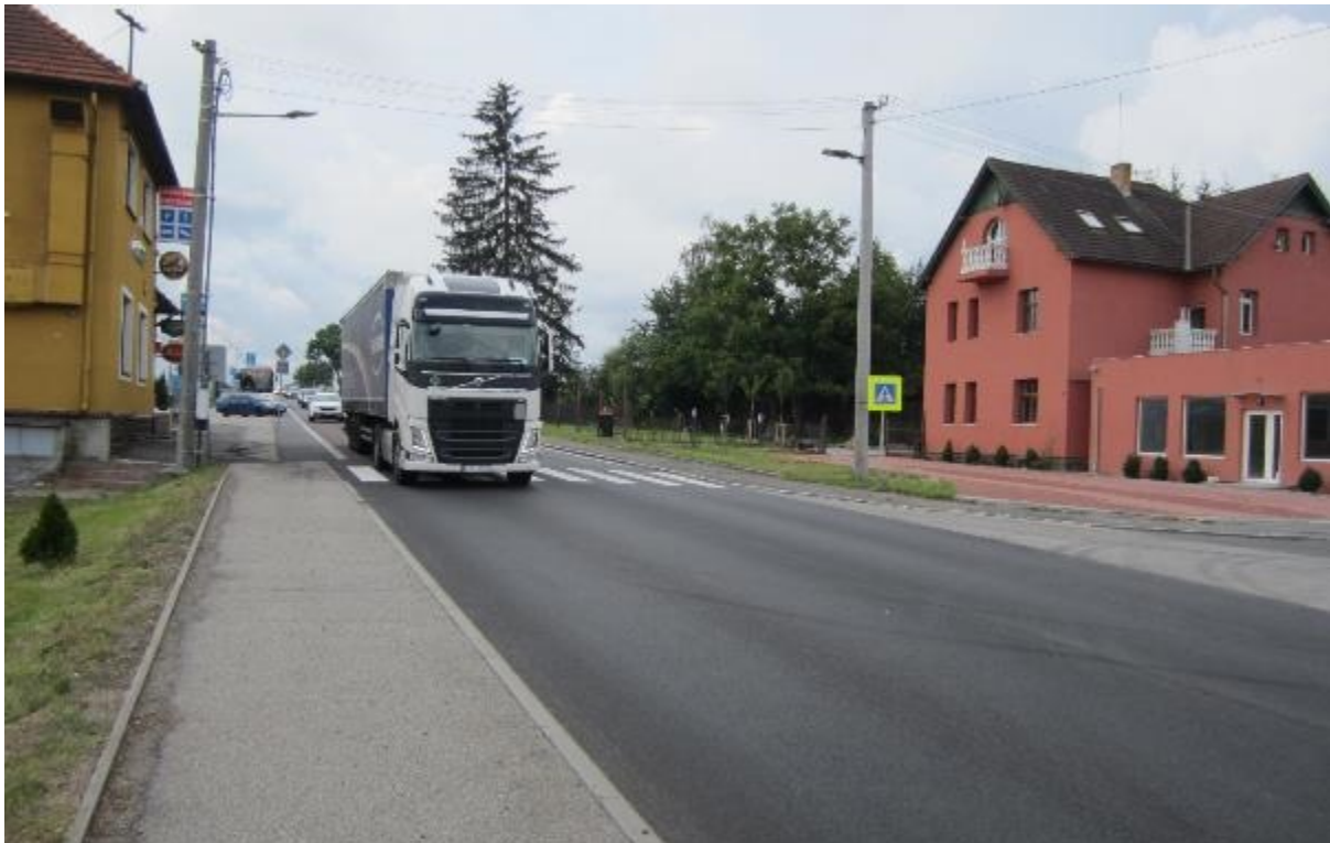
Figure 49 – 1/3 through road in Olbramovice – poorly equipped pedestrian crossing, pedestrian provisions not continuous
