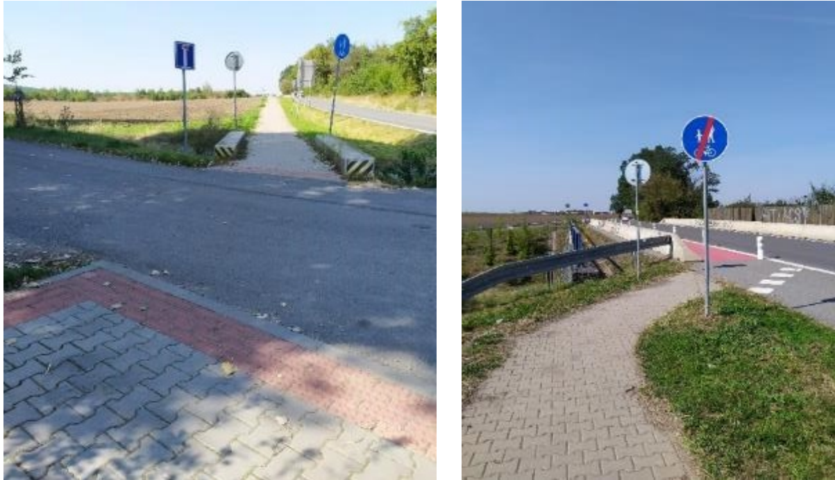
Figure 2 – Pedestrian and cycle path along the road and on the bridge across I/9
