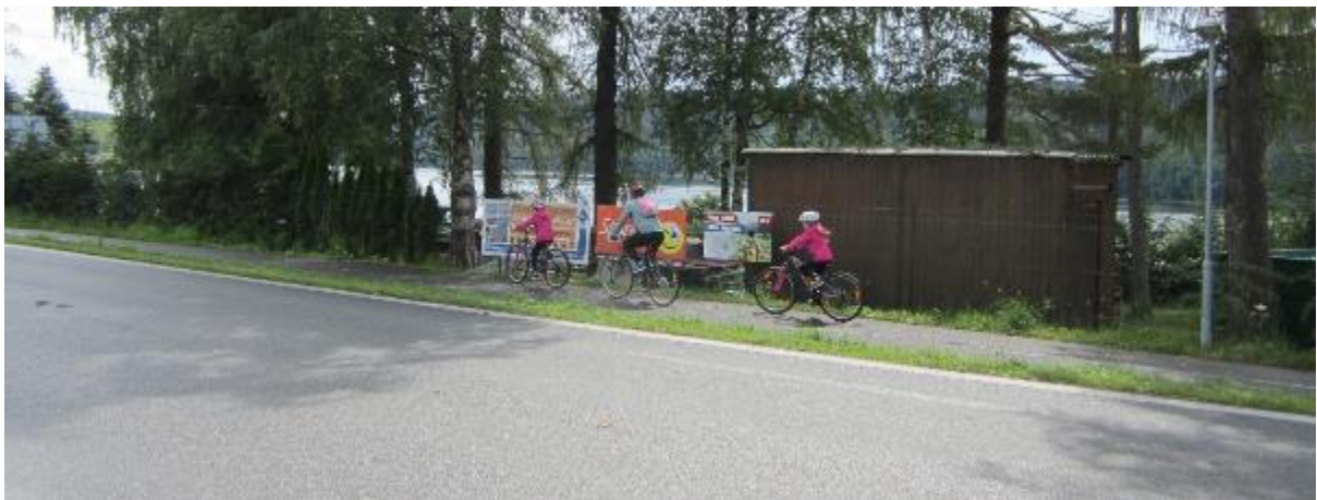
Figure 10 – Recreation area survey, road II/163, parallel mixed-use path along the Lipno water reservoir
