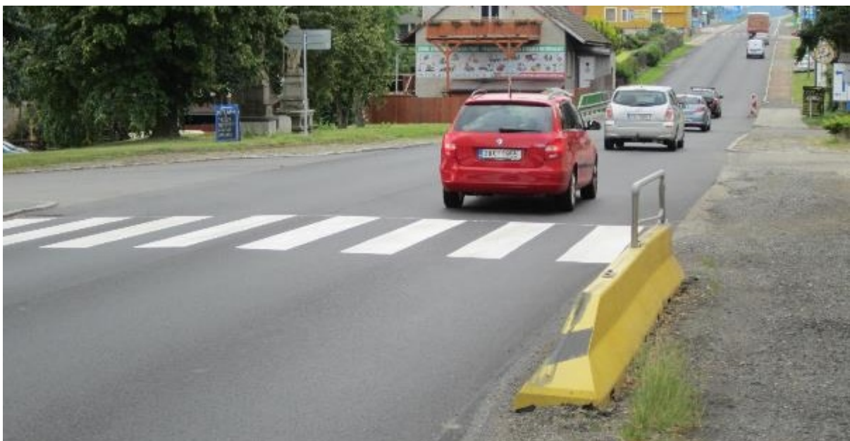
Figure 46 – 1/3 through road in Olbramovice – disputable highlighting of a crossing with a concrete barrier, sidewalks at the same level as road surface
