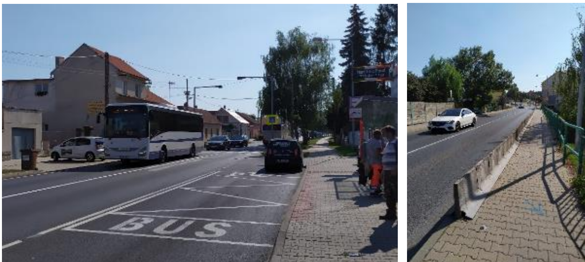
Figure 3 – Public transport stop area with elevated crossing / barrier separating a narrowed sidewalk from busy road
