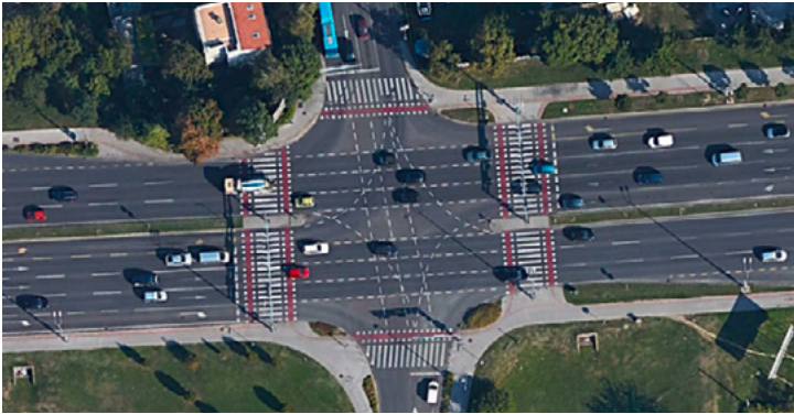
The figure shows an aerial view of a protected intersection on Zagreb Avenue in Zagreb. The infrastructure provides clear guidance for cyclists by means of a painted red cycle path around the intersection as well as guidance across the intersection. Given that cyclists and pedestrians have to cross multiple lanes, refuge islands are provided in between lanes of opposing directions of travel. The whole intersection is regulated by traffic lights [11].
