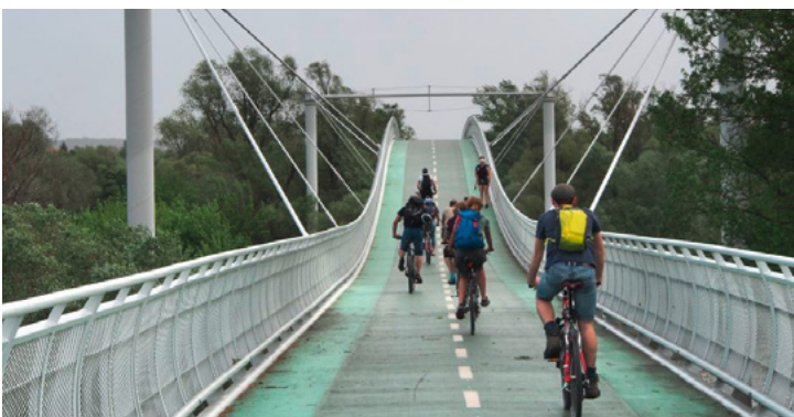
Cycling bridge in Slovakia [6]
