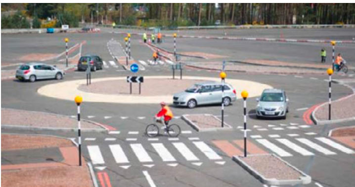
Dutch styled roundabouts where the geometry is arranged in a way that motor vehicles leaving the roundabout approach the crossings at an angle close to 90 degrees to maximise inter-visibility [1].
