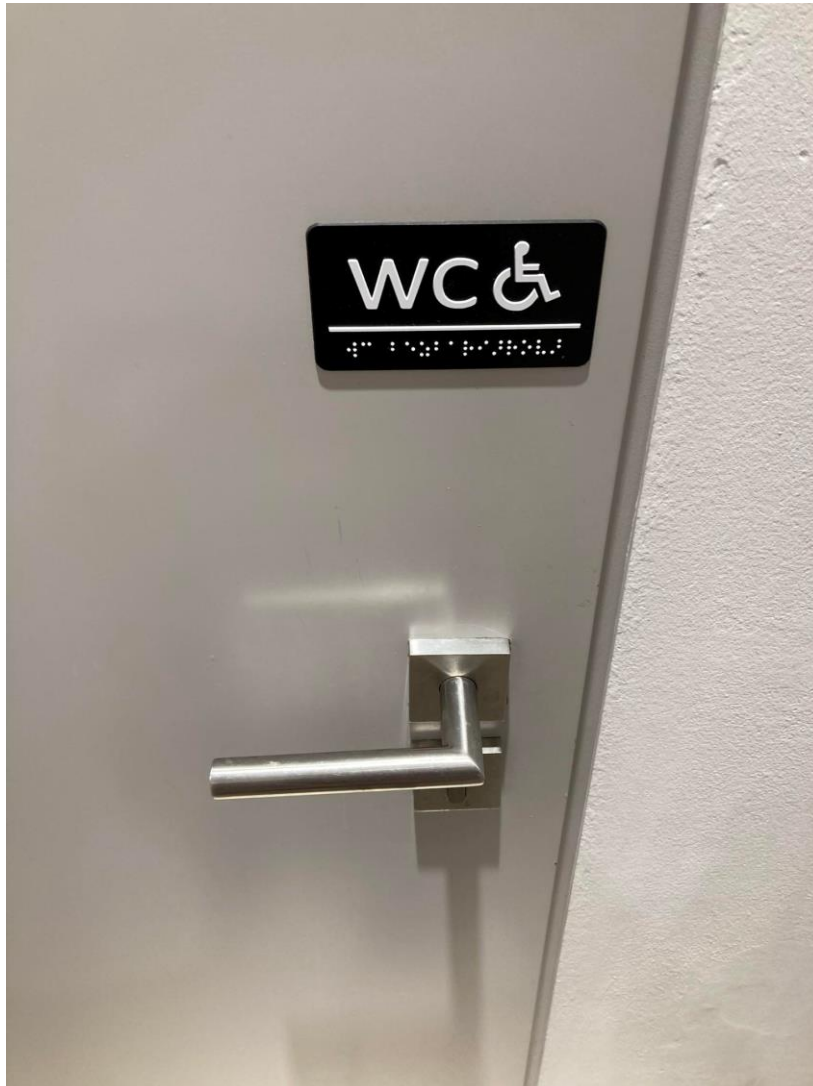
Picture 2: Braille marking on doors
