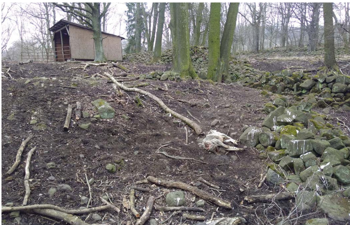
Figure 20: Damage incidents should be reported without undue delay. © Radek Kříček.
