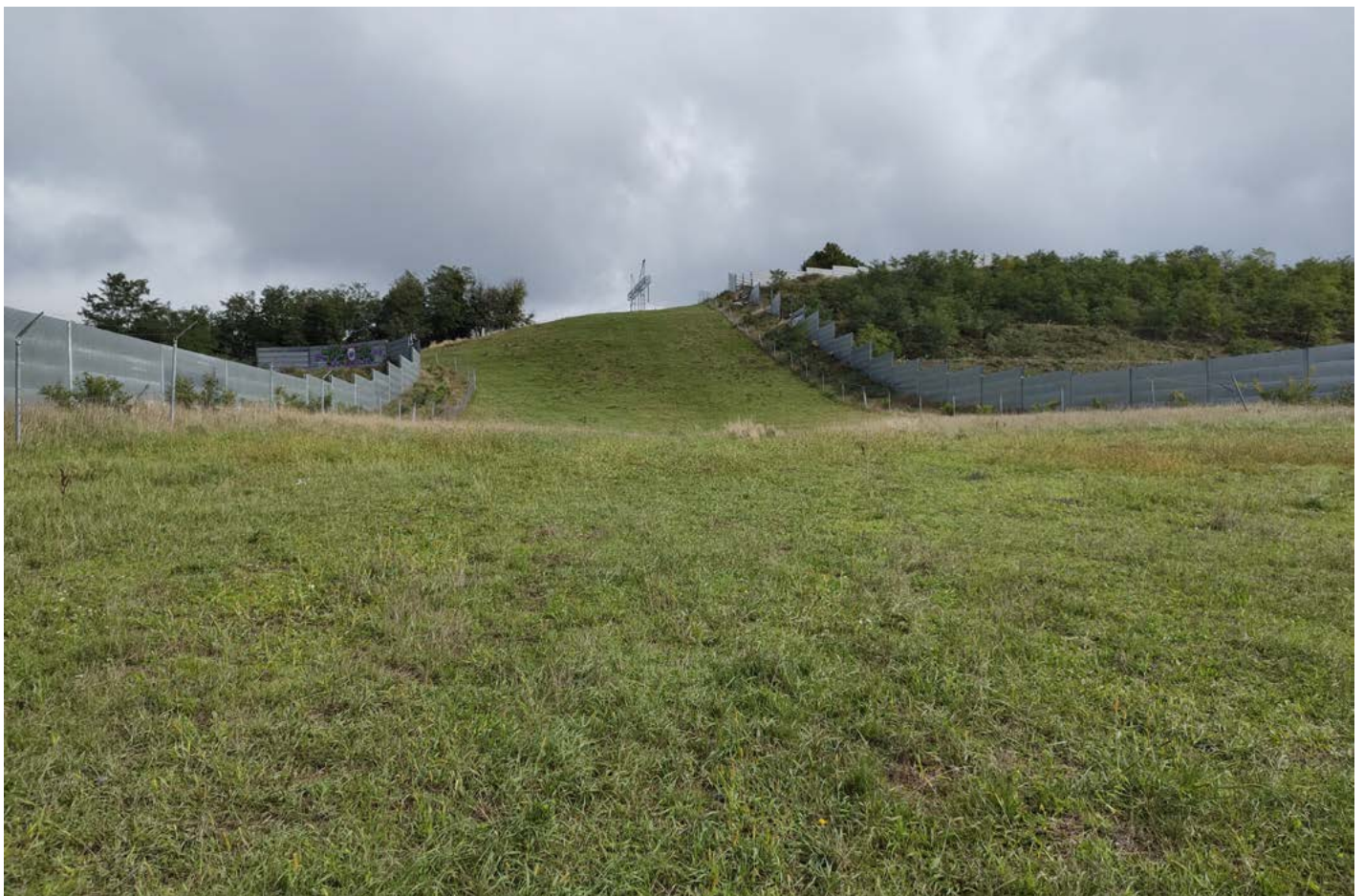
Figure 7: The green bridge over the A1 motorway in Romania is an example of a fauna passage whose functionality for different categories of animals can be significantly enhanced by simple low-cost measures (e.g. planting green islands protected from grazing). © Radek Kříček.
