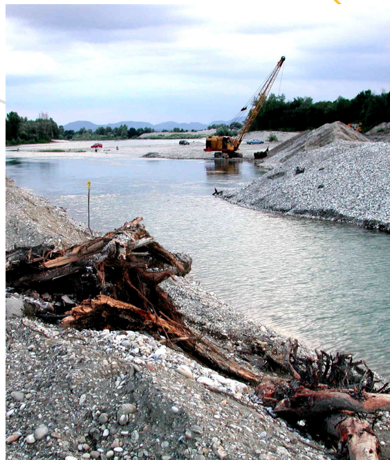
Sediment extraction from the riverbed
