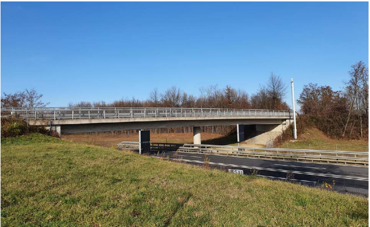
Figure 10 An overpass in the Pötttsching forest© Christoph Plutzar
