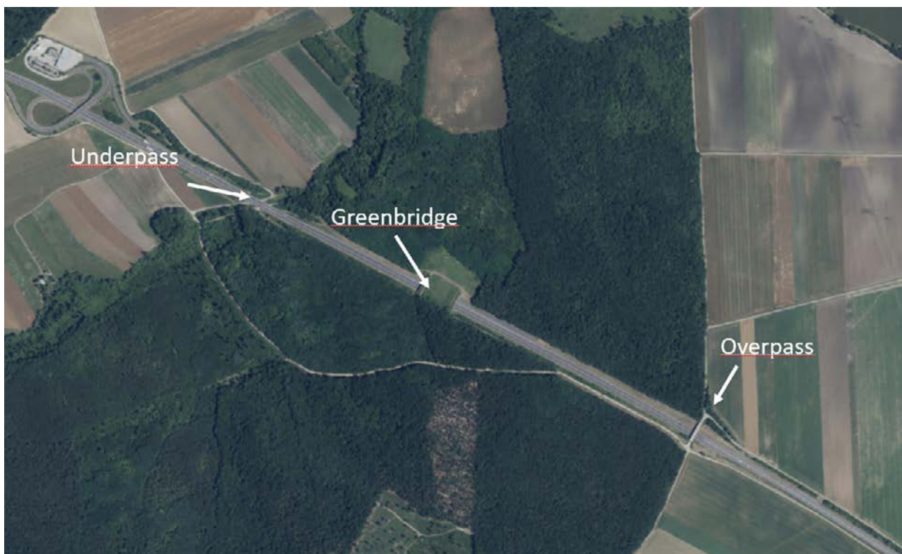
Figure 8 Crossings in the Pötsching forest, © Environment Agency Austria/Geoland Basemap
