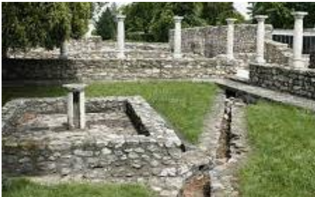
Rainwater channels must be checked and kept clean and functional
