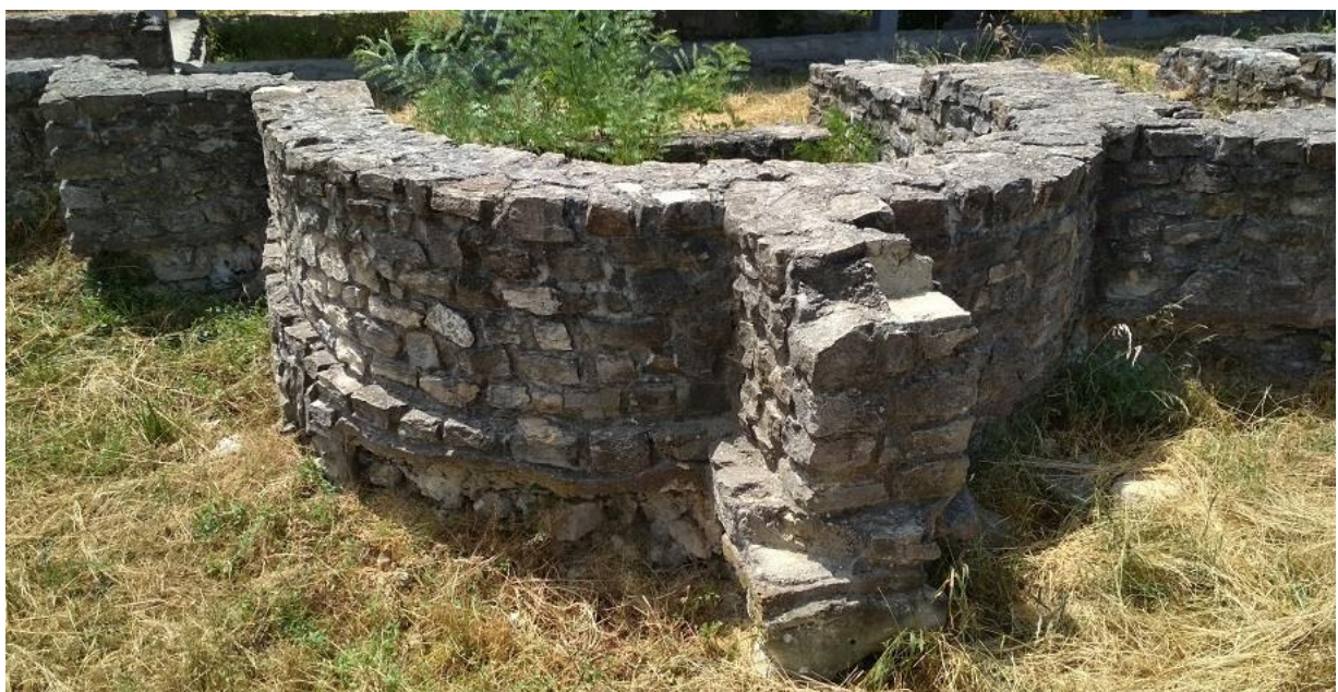
Example of combined weathering and vandalism damage
