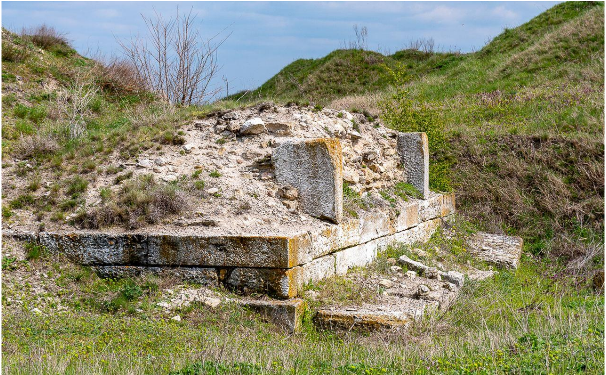
Example of masonry degradation and biological soiling (Sacidava, Romania)
