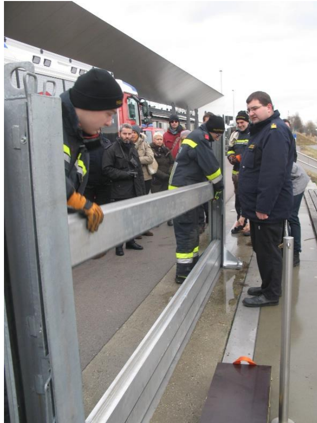
Example of a training exercise of erection of a temporary barrier against flood (Stein, Austria).
