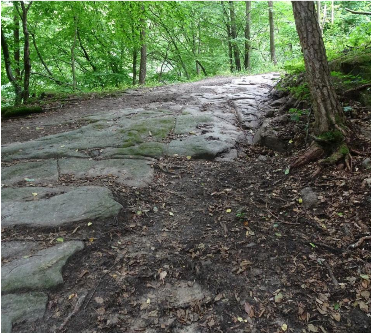
Well maintained road pavement (Bacharnsdorf)
