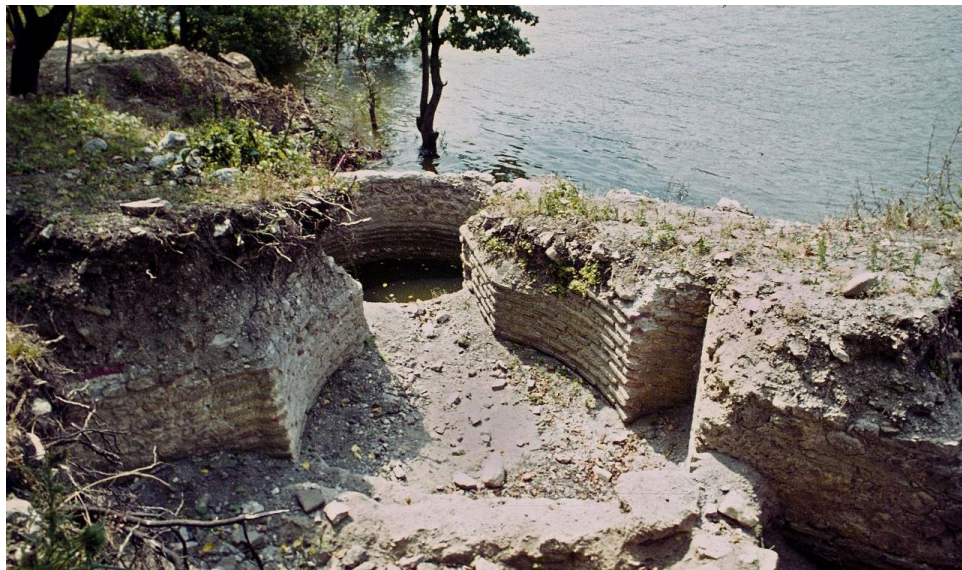
Loss of building elements, loss of integrity due to weather and neglected maintenance (Bosman)
