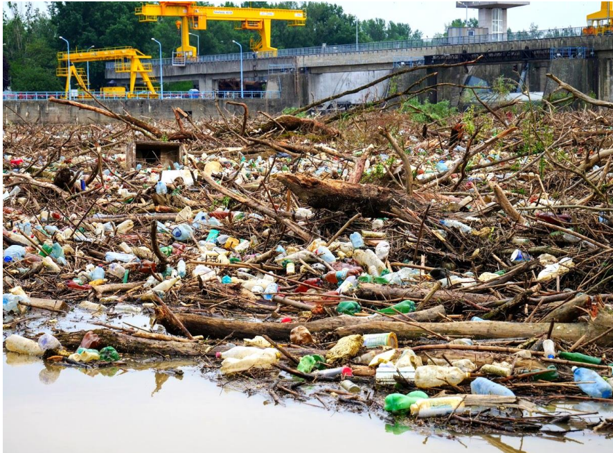
Fig.5. Plastic and driftwood accumulation after a flood in downstream Hungary, at the Kisköre hydroelectric power plant. The temporary structure can be 3 meters thick and reach more than a hectare in overall size.
