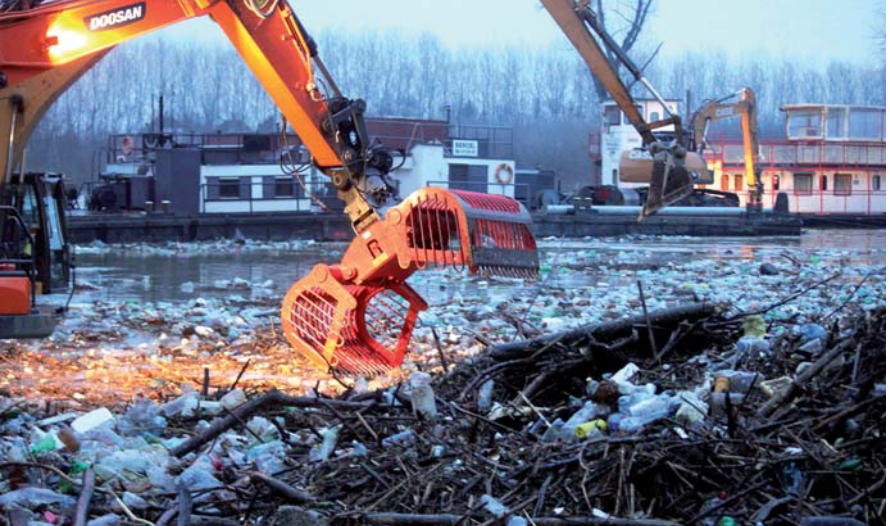
Partial river bed blockage on the river Tisza at Vásárosnamény during a winter flood in 2021. The temporary structure operated by FETIVIZIG successfully recovers about 90% of the floating plastic particles to the shore for recovery
