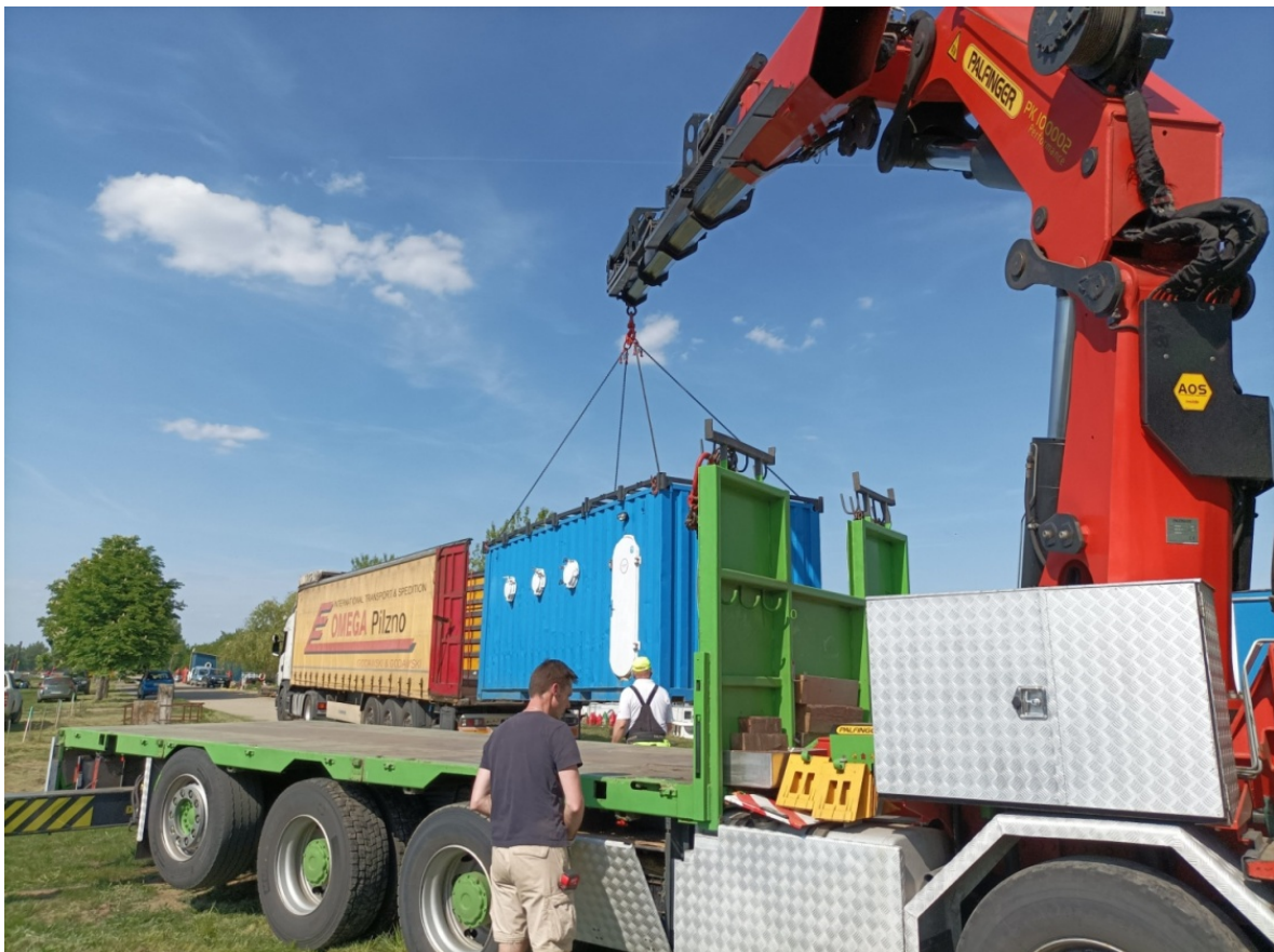
The FLEX containers are lifted by a crane onto the transporting vehicle preparing them for the trip to Slovakia.
