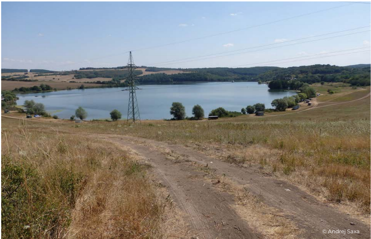
Figure 67 South view of water dam of Ľuboreč.
