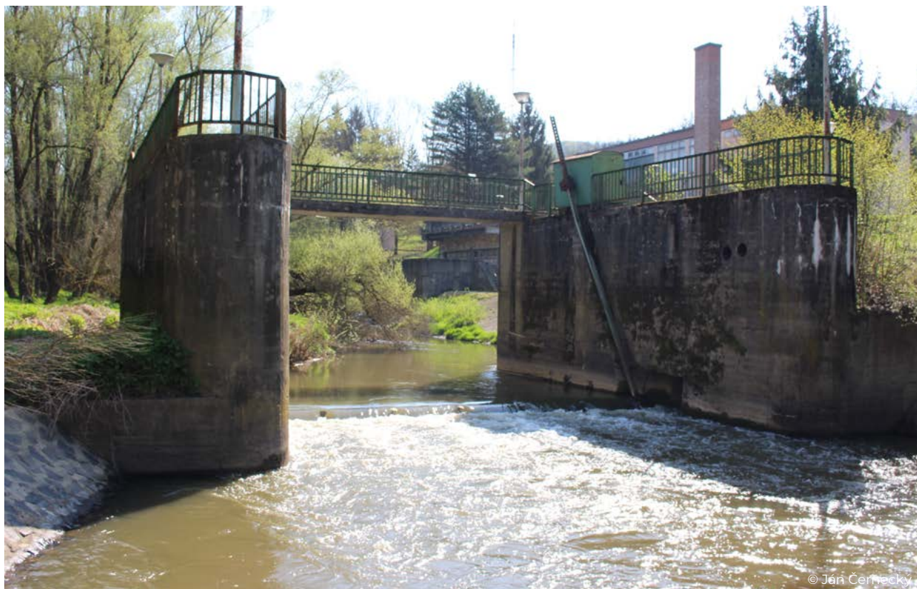
Figure 57 Iron-concrete migration barrier on the Ipeľ River near the village of Muľa.
