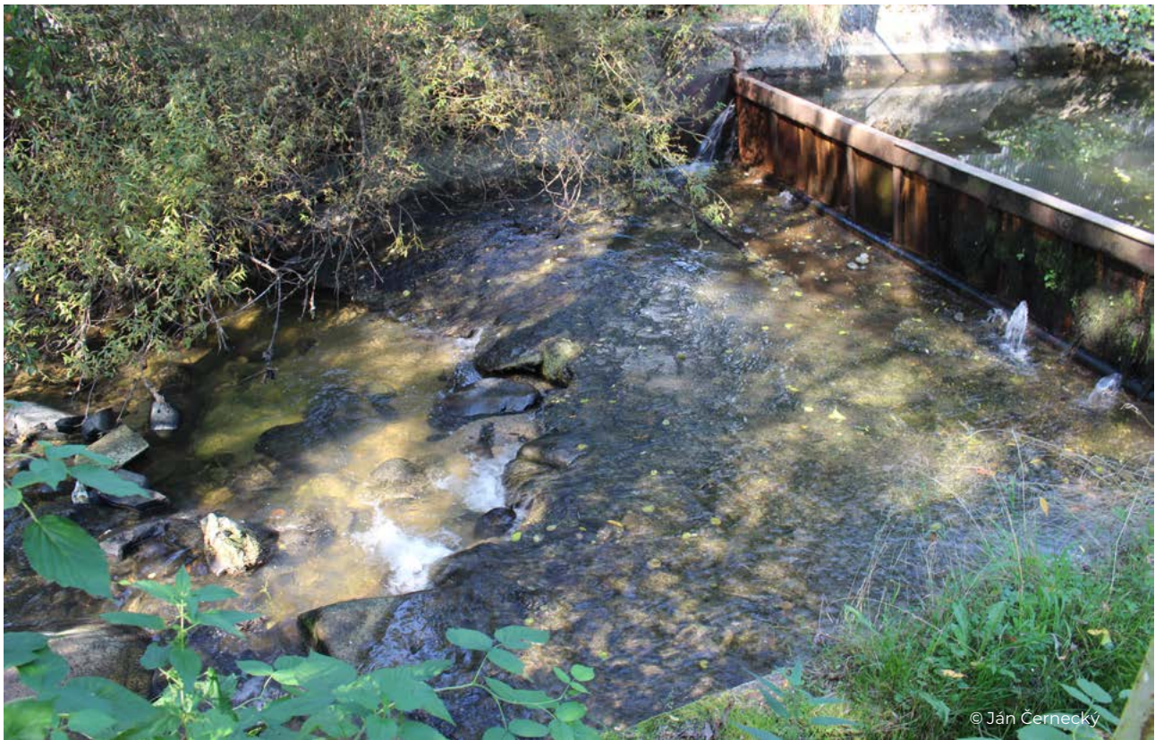
Figure 39 Cross structure on the Slatina River in Hřiňová - part Krivec. In the upper right corner, you can see the outlet of the fish conduit.
