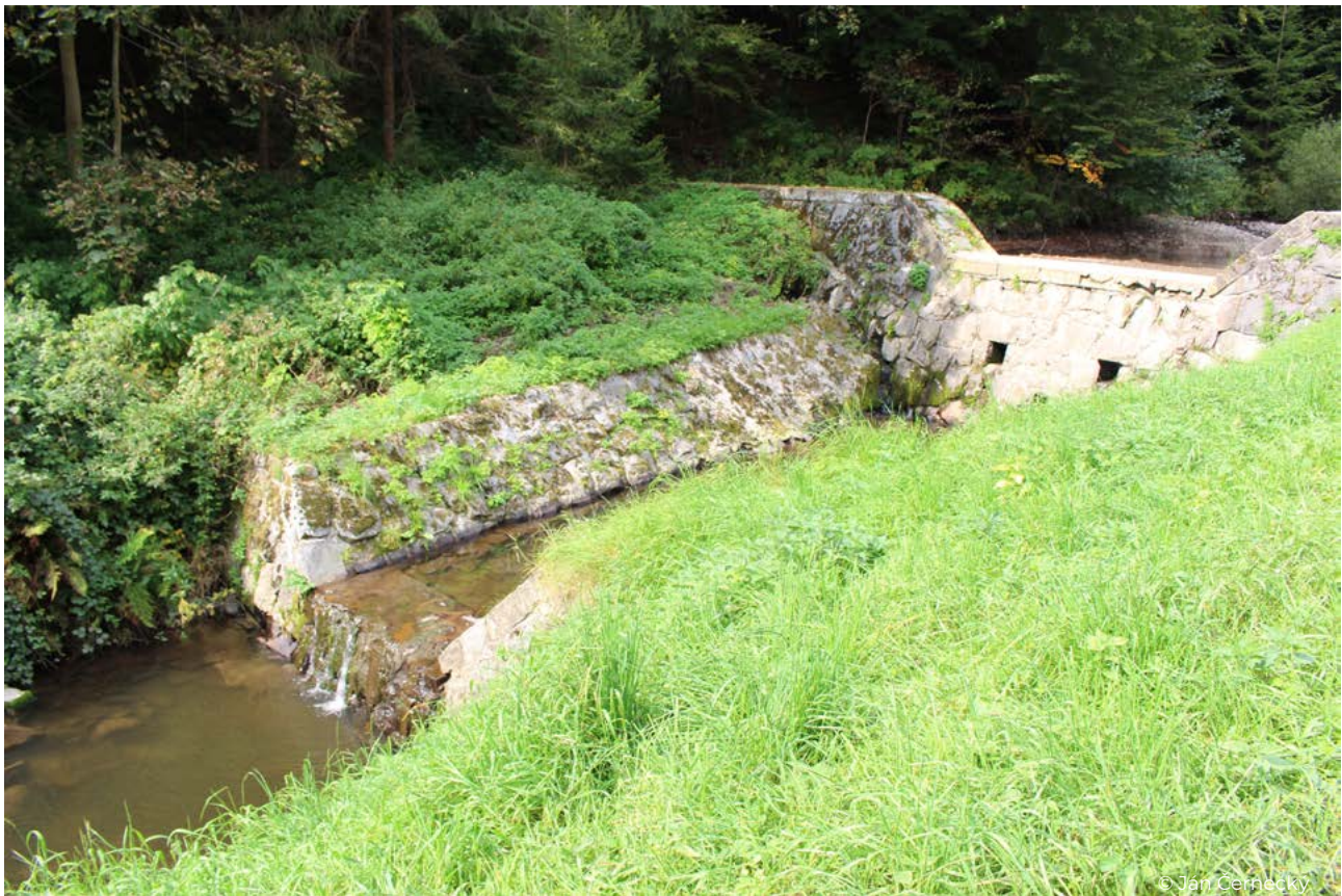
Figure 35 Transverse barrier at Hukava, Hřiňová district, water surface elevation approximately 3 metres.
