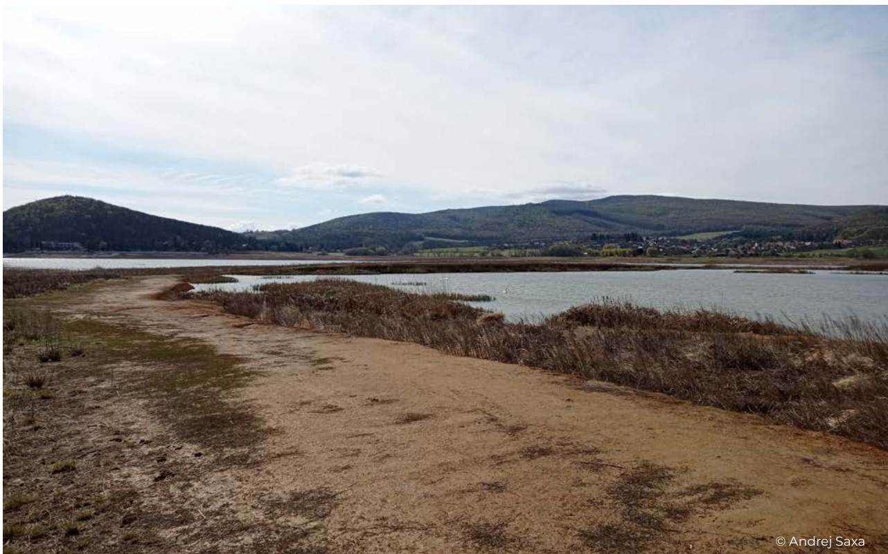
Figure 66 The main works on the facilities of the Ružiná reservoir (from 2019) have been completed and the reservoir is gradually being refilled.
