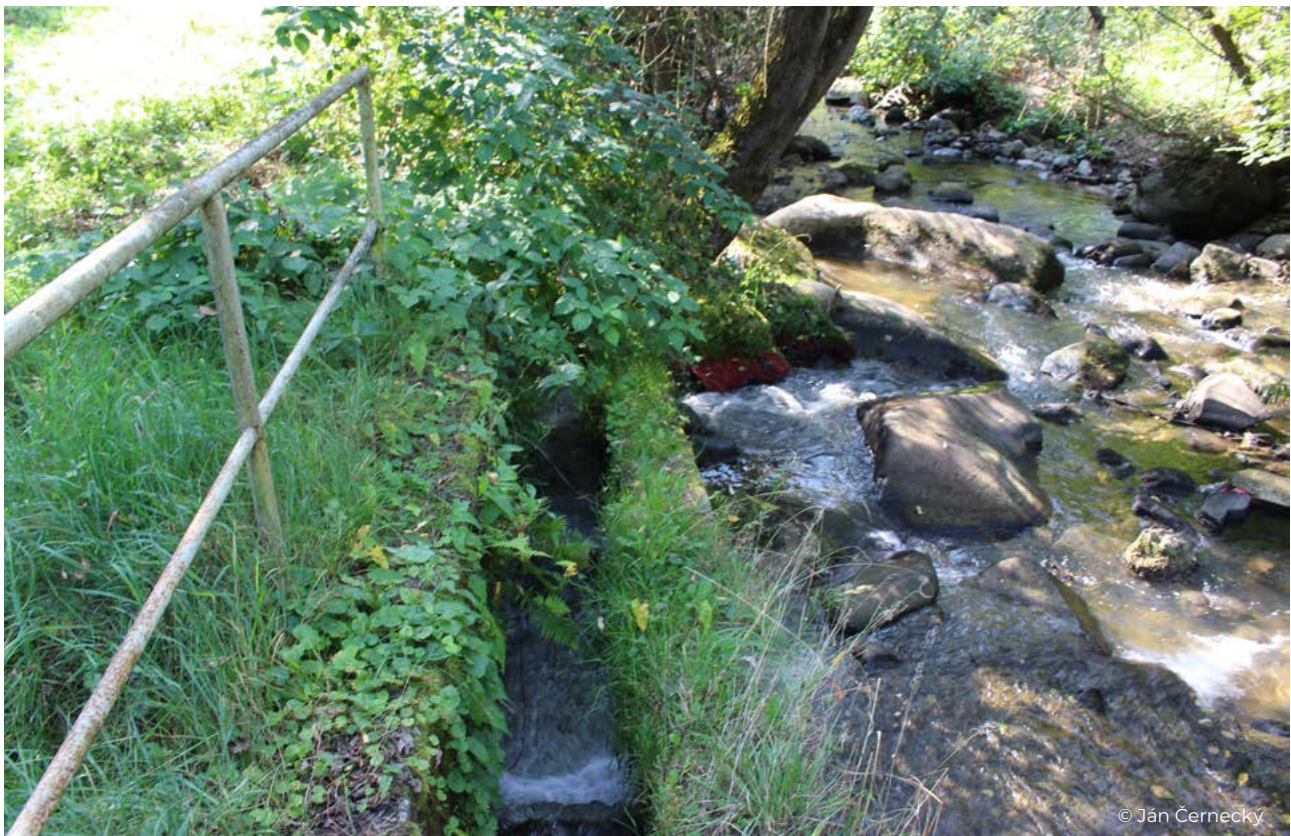
Figure 40 View of the inappropriate fishway at the barrier on the Slatina River (Hřiňová - part of Krivec).
