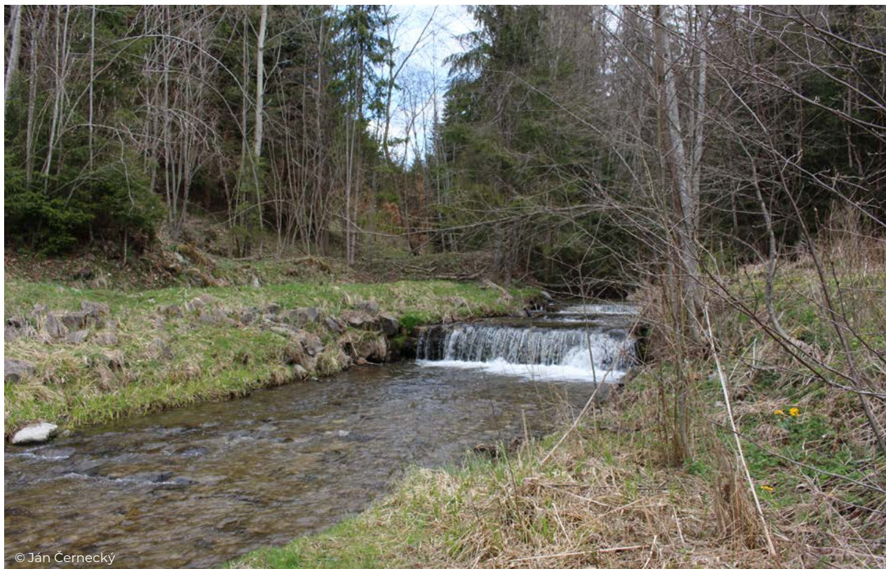
Figure 49 The grade on the Slatina River (above the water dam Hriňová, near the Belovodský Bridge) creates a level difference of approximately 0.5 metres.
