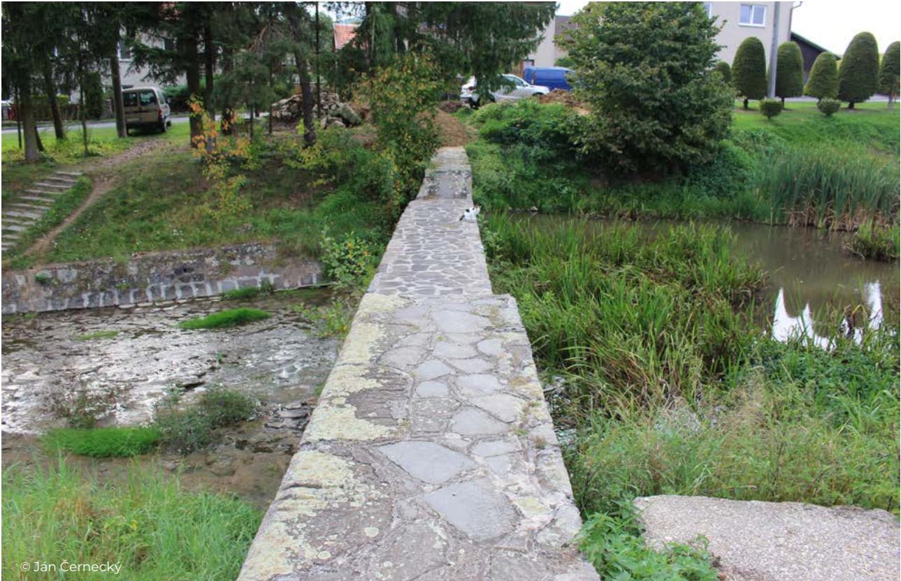
Figure 48 Transverse barrier on the Detsviansky potok brook in the old part of Detva.
