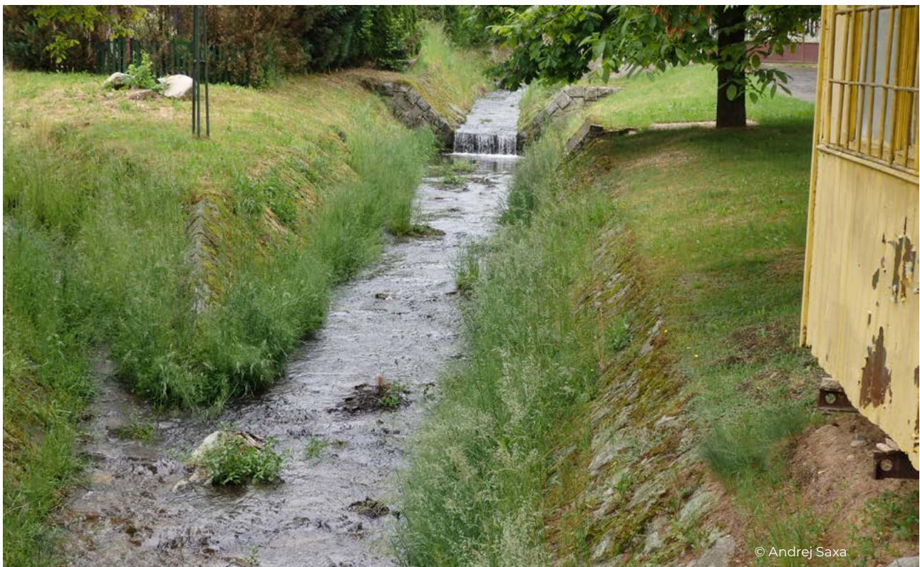
Figure 69 The Dobročský potok brook flowing through the village of Dobroč with straightened and regulated banks and bottom.
