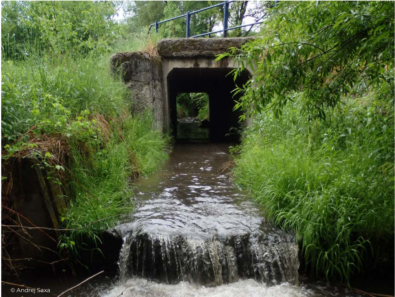
Figure 74 The grade on the Tuharský potok brook below the village of Tuhár stabilises the bridge structure of the road III/2665.
