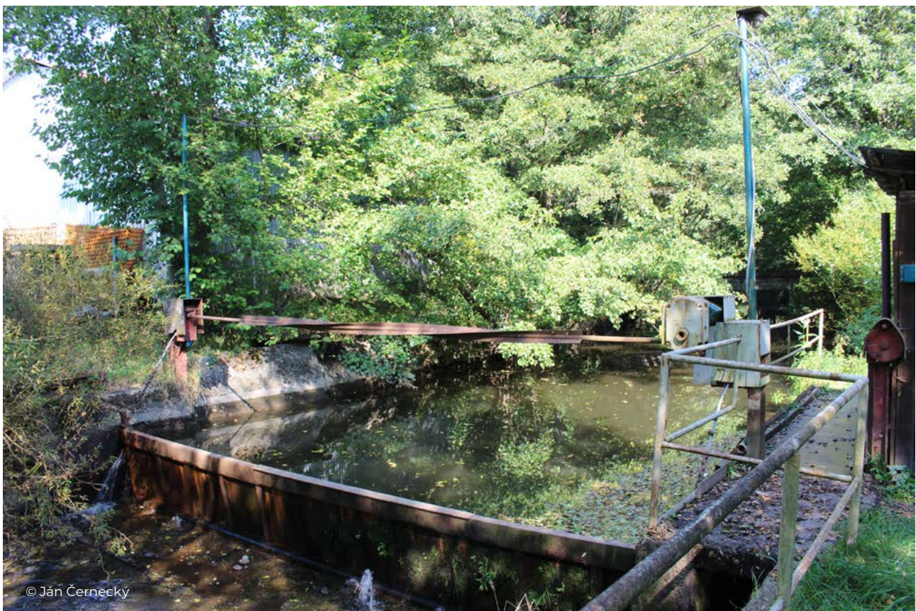
Figure 38 Cross structure on the Slatina River in the town of Hriňová - part of Krivec.
