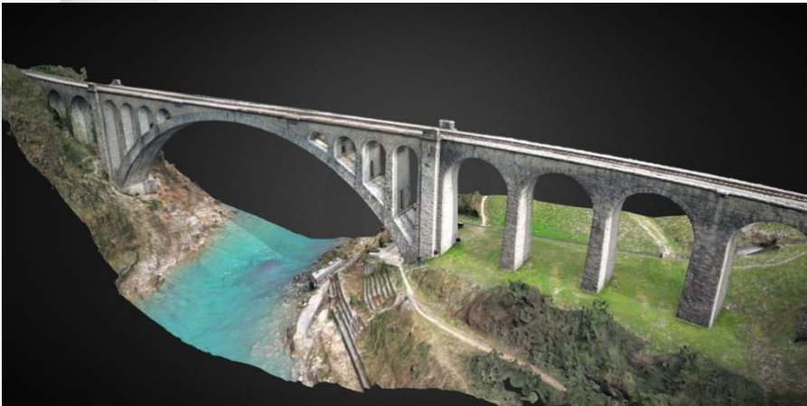
Figure 3: 3D model of Railway Bridge in Solkan (Commissioned by: Javni zavod za turizem Nova Gorica in Vipavska dolina)
