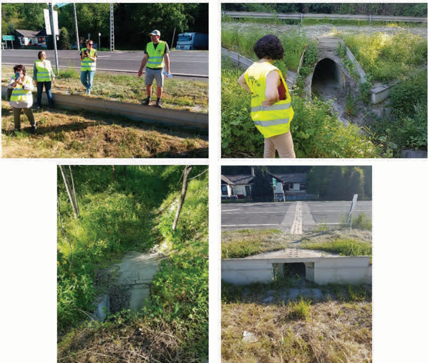
Figure 32 During SaveGREEN Transnational Experience Exchange Workshop we visited “the amphibian guidance (wall) system”
