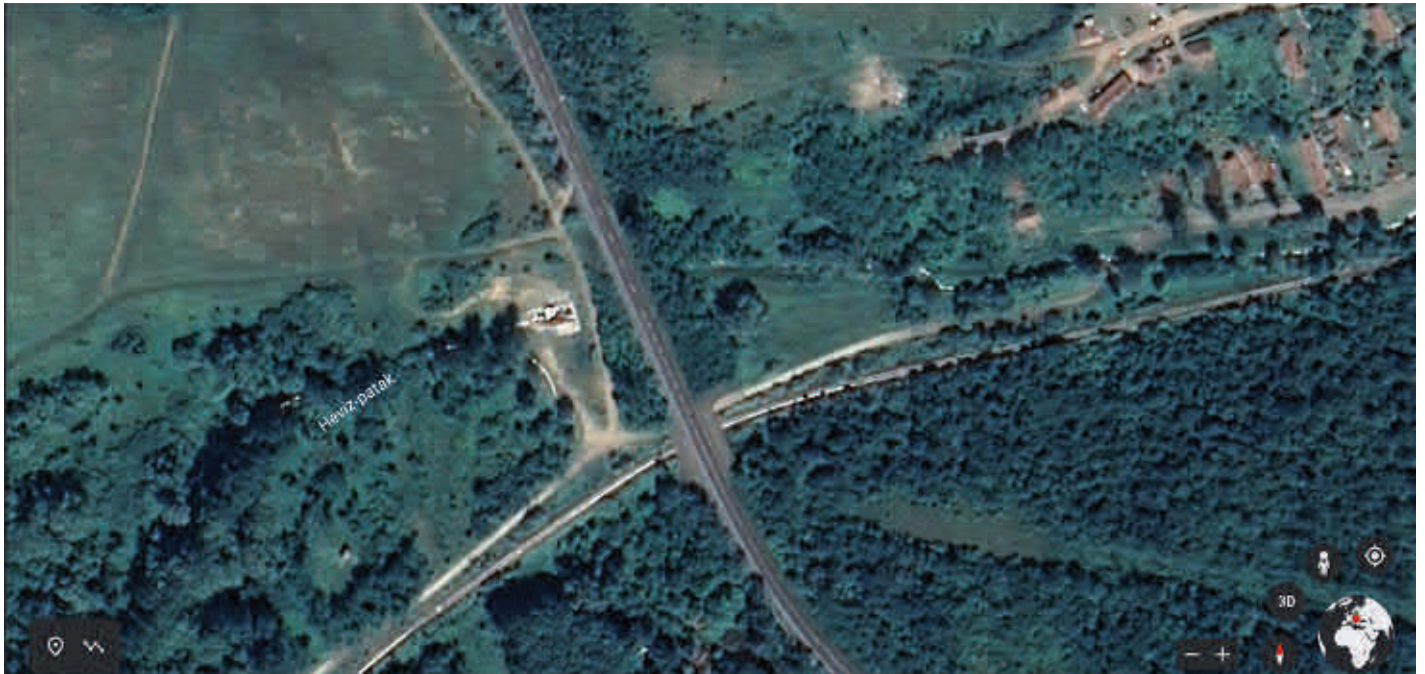
Figure 27 Road No. 2 crossing of the Hévíz-stream with an inappropriately sized culvert on Google Earth
