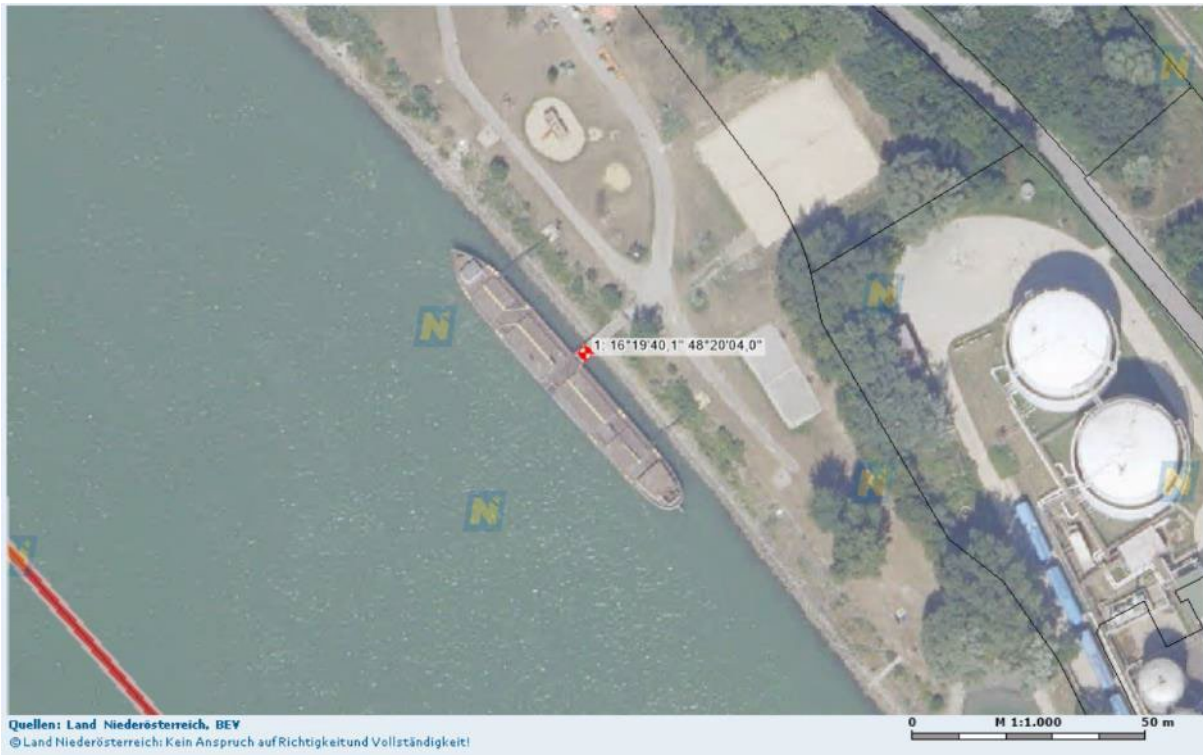
Annex 1: Site plan/coordinates of the sedimentation box and aerial photo of the sampling site in Korneuburg
