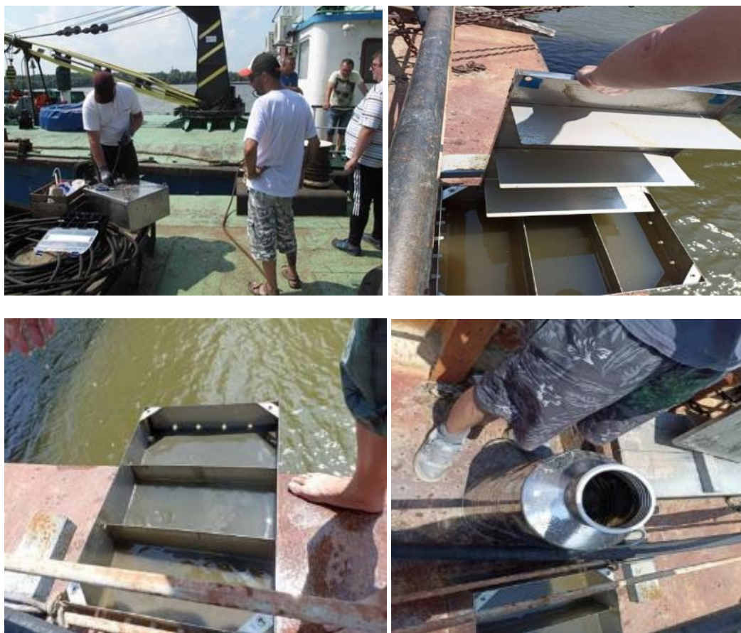
Figure 45: Attaching and removal of the Sedimentation box in Ruse
