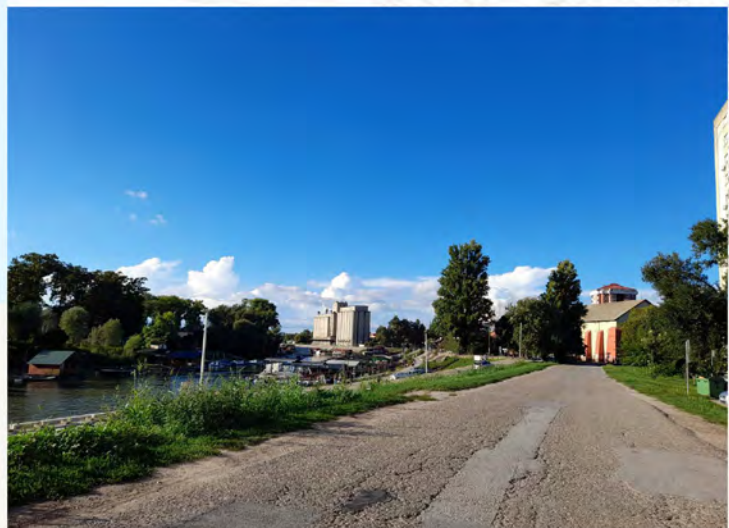
Fig. 280_02: A 'new silo' and 'new port' in Pančevo, which was the most industrialised cities in the former Yugoslavia during socialist decades, with a substantial number of heavy industries. This was followed by intensified demographic growth (Author: D. Milošanović Rodić)
