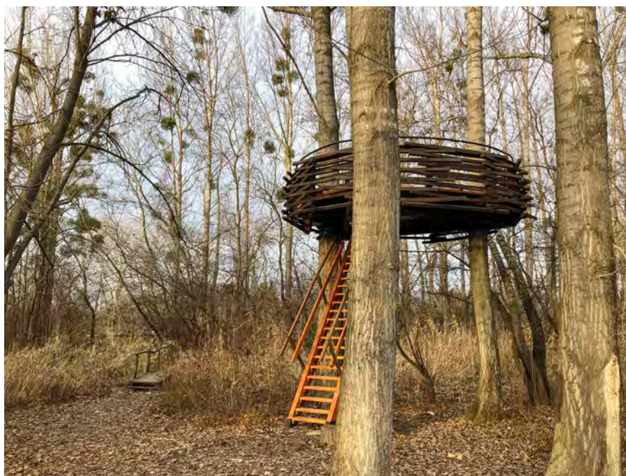
Fig. 328 / Small wooden interventions on the Little Danube: Lookout Tower in Malinovo (Authors: L. Vitková & K. Smatanová).
