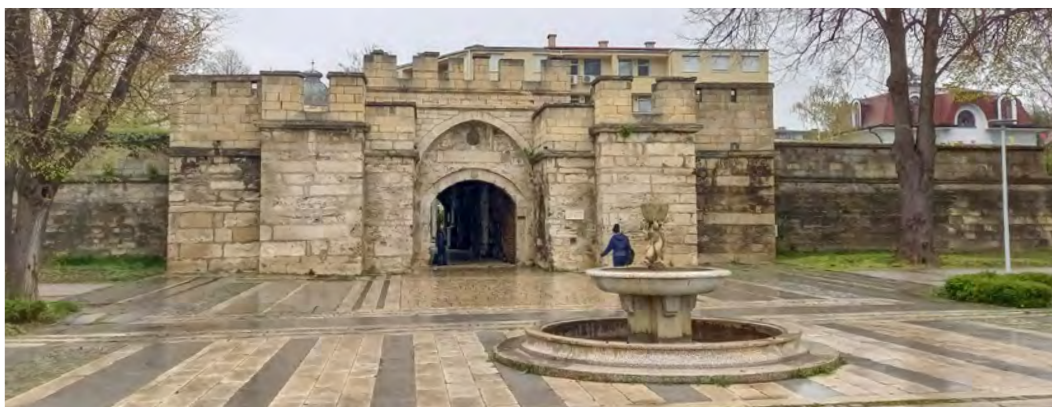
Fig. 296 / The restored zone of the walls of Vidin medieval fortress (Author: G. Georgiev)
