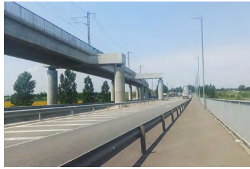
Fig. 255 / “New Europe” Bridge across the Danube bridge between Vidin, Bulgaria, and Calafat, Romania, combines road and railway (Author: Bulgarian Guide, 2022).
