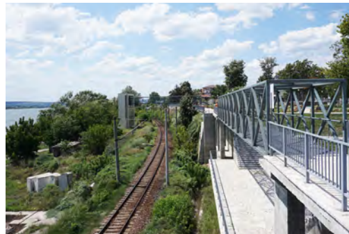
Fig. 315 / The railway overpass to the pier of Trajan's Bridge (Author: M. Găman, 2021).
