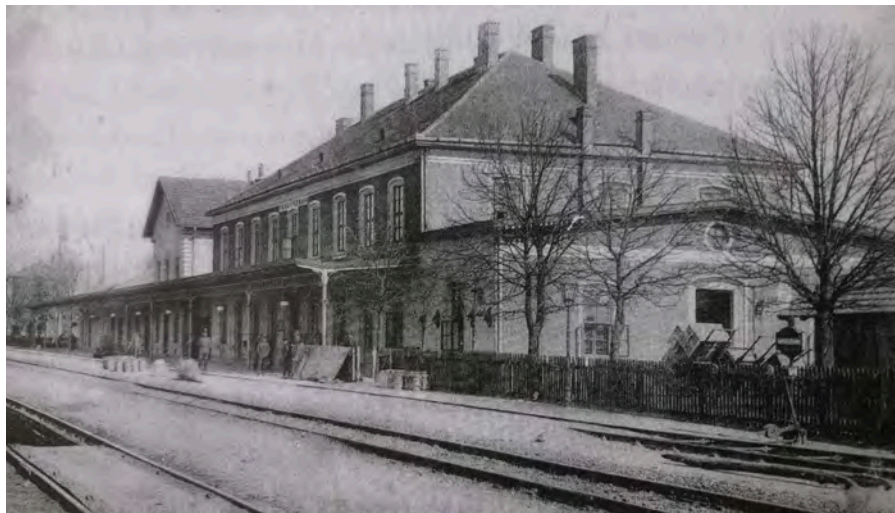
Fig. 093 / Štúrovo – railway station as a node of development in 1920s (Baka, 2021).
