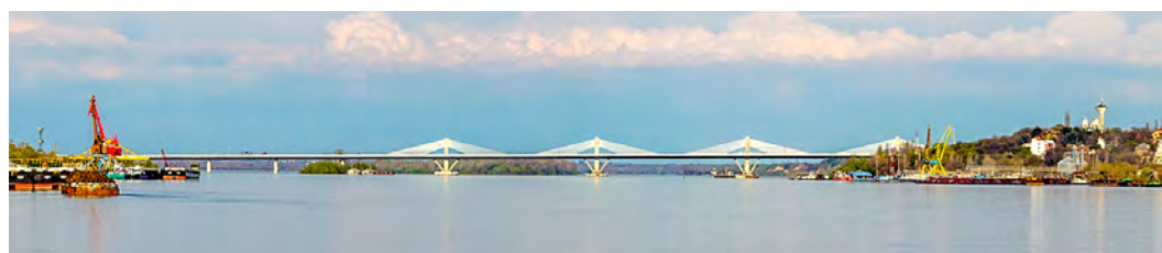
Fig. 206 / The recently opened “New Europe” Bridge between Vidin and Calafat (Author: New Bulgarian Guide, 2022).
