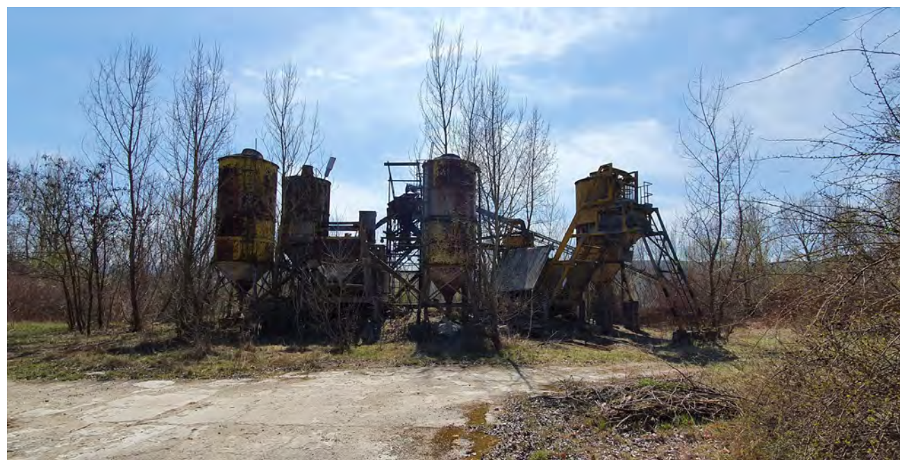
Fig. 179 / Former concrete production line, another industry left in decline in Szob (Author: B. Kadar, 2021).
