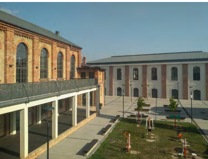
Fig. 072 / The former industrial yard in the silk factory become new open public space in Mohács downtown (author: D. Siljanović Kozoderović, 2022)
