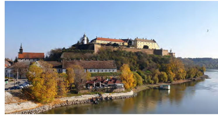
Fig. 253 / Petrovaradin Fortress above the Danube in Novi Sad, the regional centre of northern Serbia and the administrative seat of the Autonomous Province of Vojvodina (Author: P. Morgenstein, 2021).
