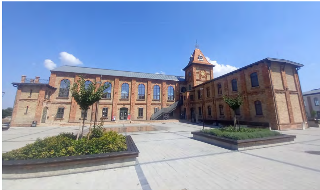
Fig. 071 / The main building of the silk factory of preserved its central role in the complex as an event and business premise (author: KEK, 2022).
