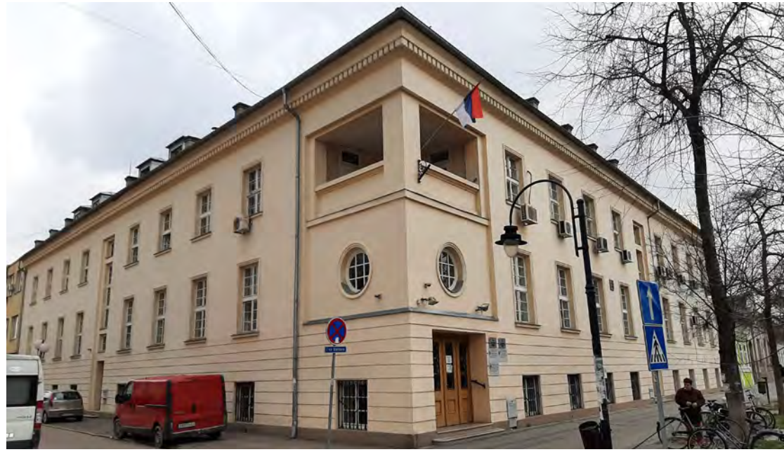
Fig. 103 / Social insurance building (1931) in Sombor is an extremely rare example of Art Deco style in the present-day Serbia (Author: D. Siljanović Kozoderović, 2021).
