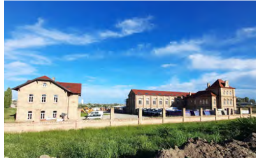
Fig. 082-083 / The Silk factory in Pančevo – before (Author: B. Nikoličić, 2015) and after partial reconstruction (Author: D. Milovanović Rodić, 2022).
