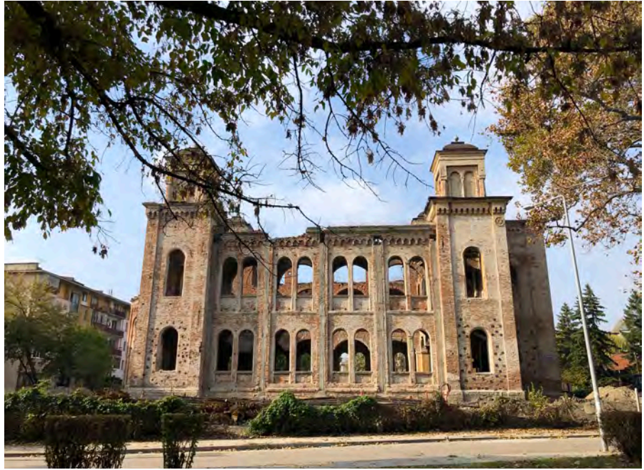
Fig. 320 / Vidin Synagogue under the first phase of reconstruction (Author: M. Jordanova, 2021).
